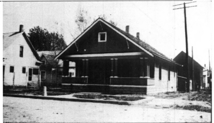
413 E Morris Street, c 1912. First rental home of Ira and Minnie Winders (extant. Not nominated/non-contributing)
