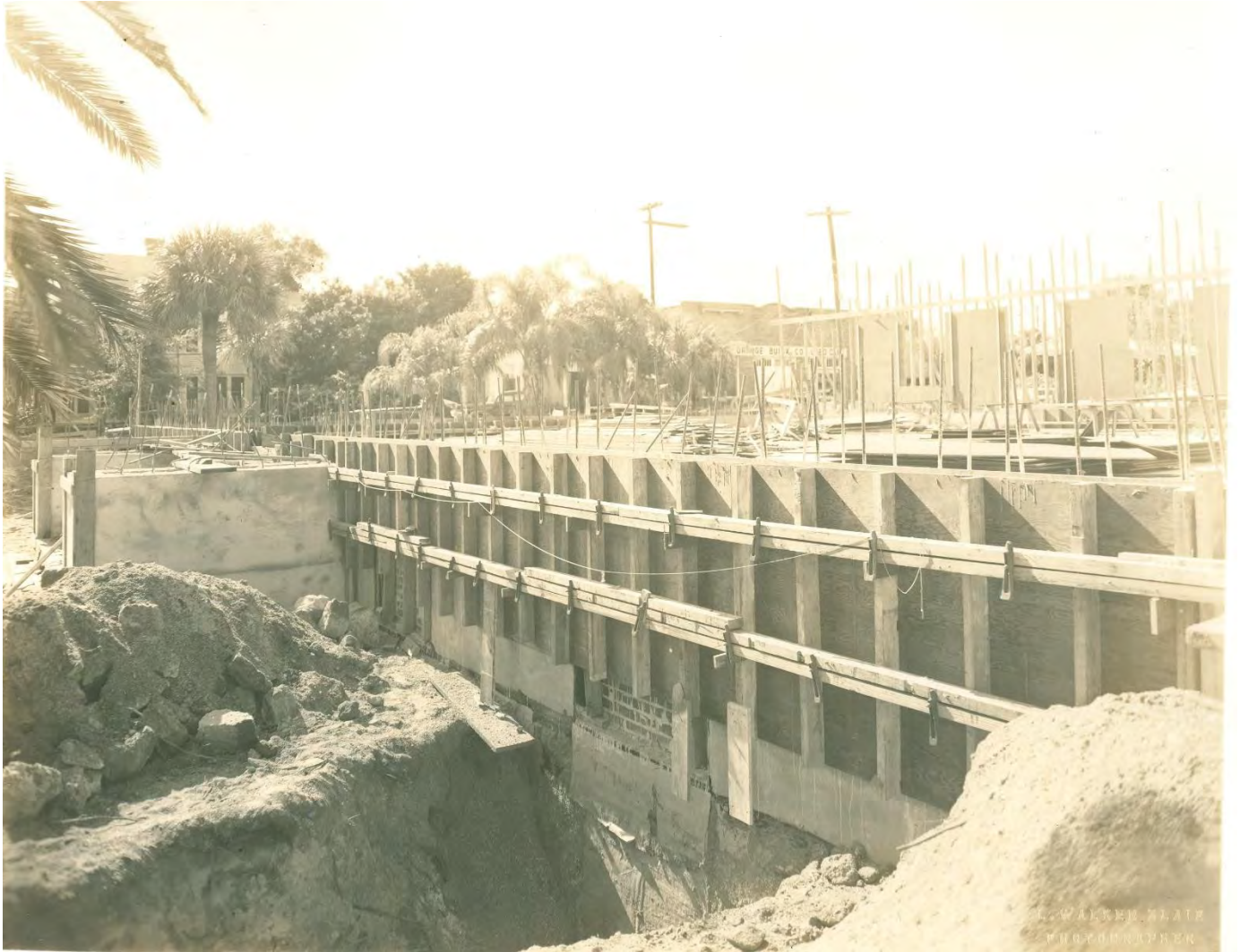
Figure 2: View of the walls of the Cocoa Post Office being poured, captured by an unknown photographer in 1939. Source: Brevard County Historical Commission Archives
