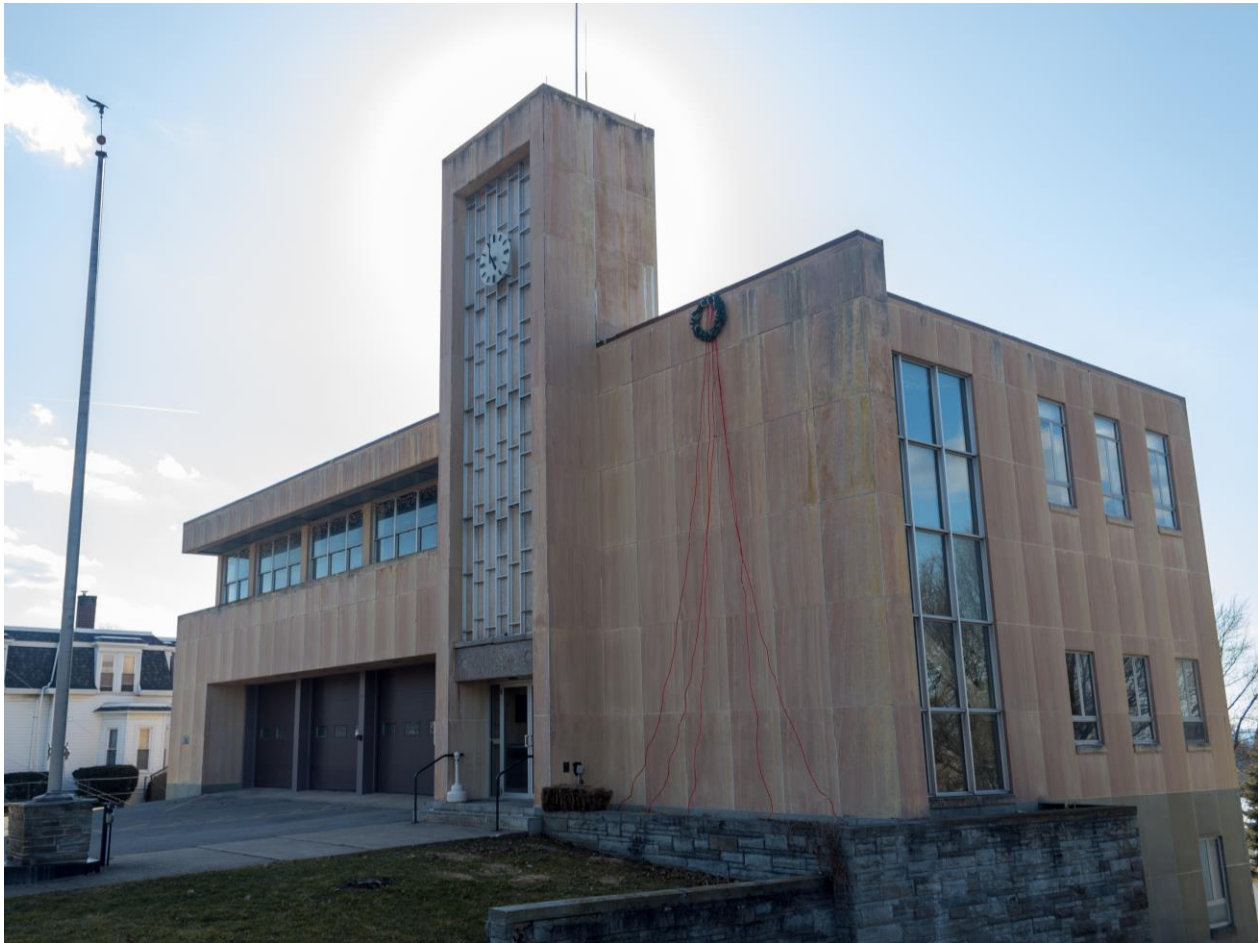
Former Ovid Municipal Building. (Photo courtesy of Edith B. Ford Memorial Library.)
