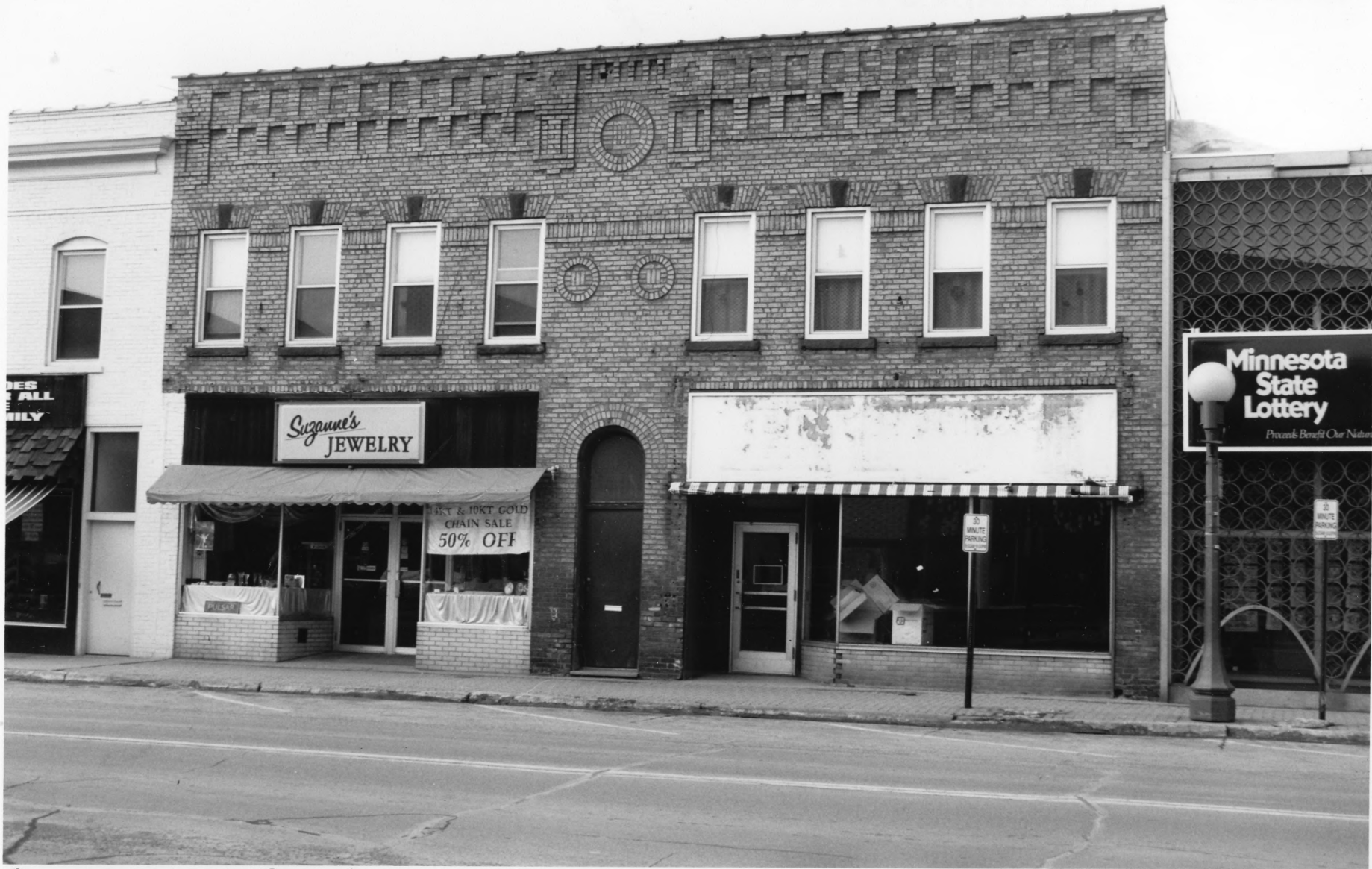
Commercial Building Virginia Commercial Historic District St. Louis Co., MN 012928-16A/17
