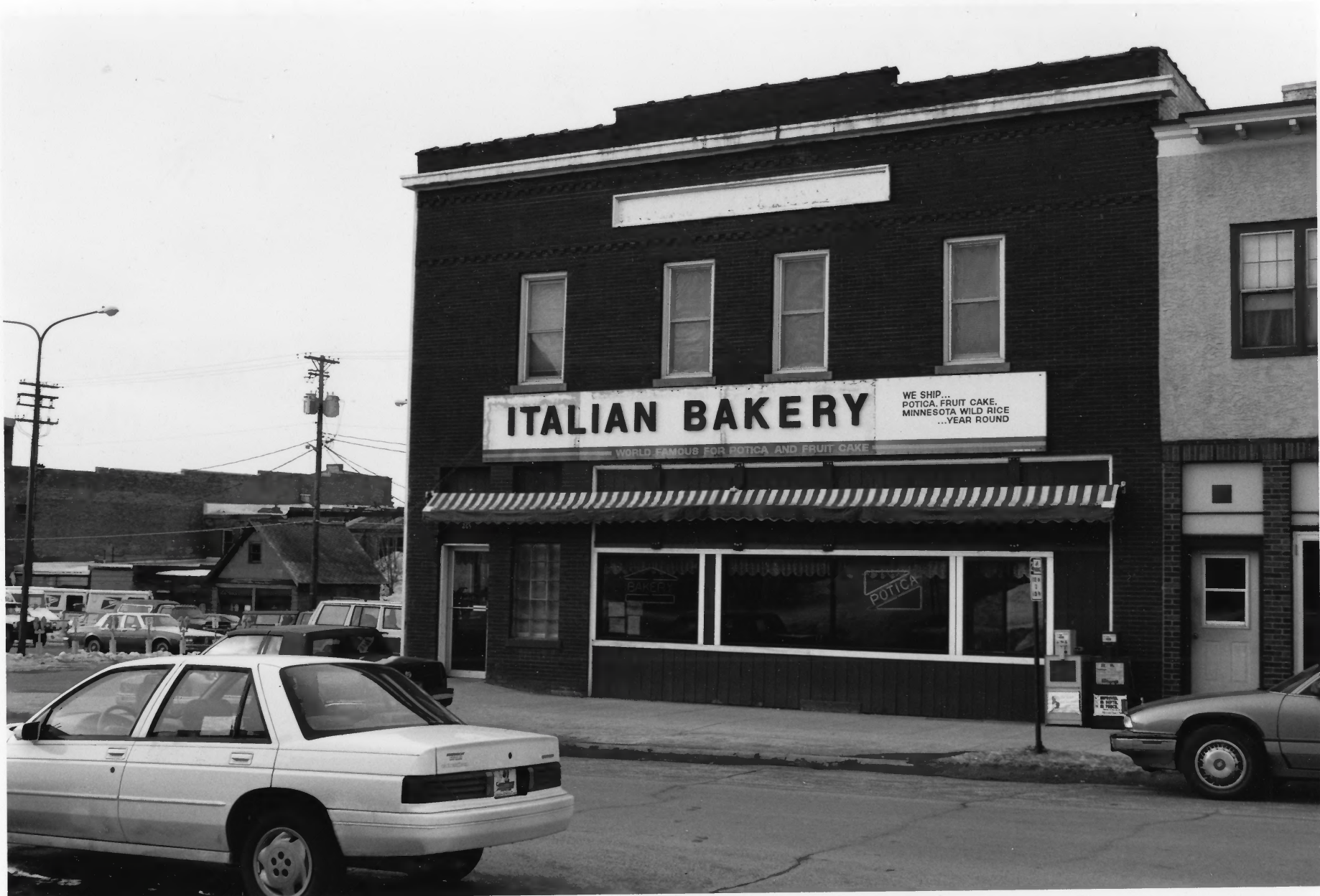
Commercial Building Virginia Commercial Historic District St. Louis Co., Mn 012926-11/11A
