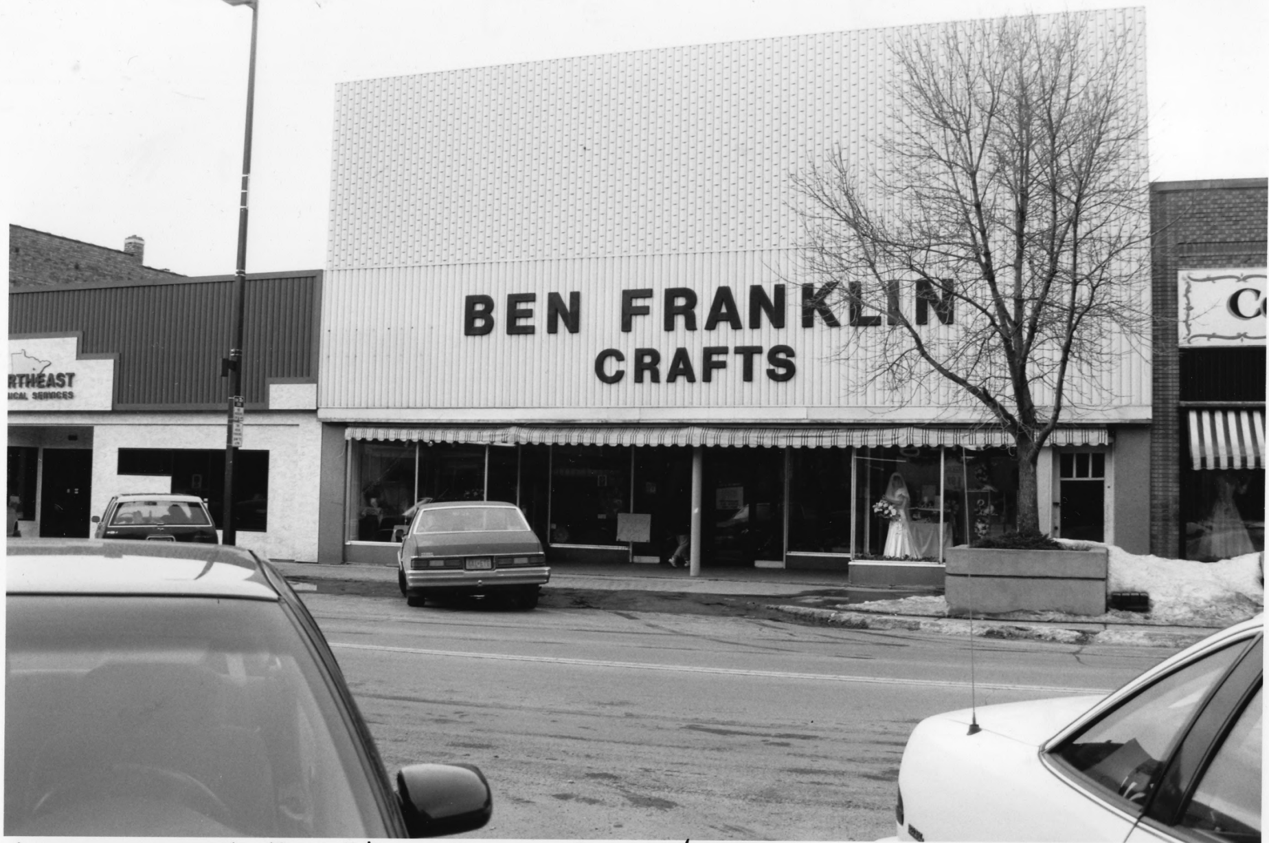
Commercial Building (non-contributing) Virginia Commercial Historic District St. Louis Co., Mn 012928-10A/11
