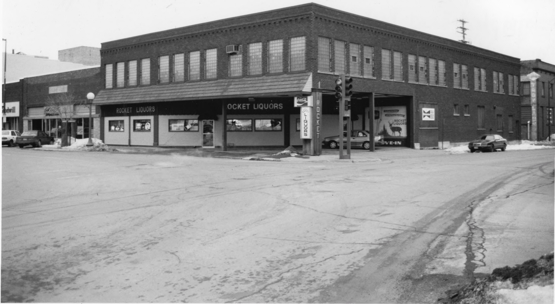
Commercial Building Virginia Commercial Historic District St. Louis Co., Mn 012929-23A/24
