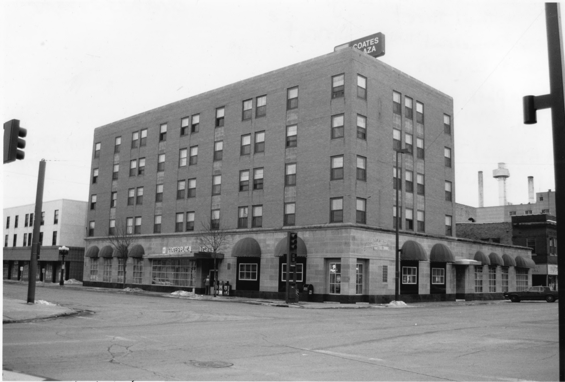
Coates Hotel (non-Contributing) Virginia Commercial Historic District St. Louis Co., Mn 012929-17A/18
