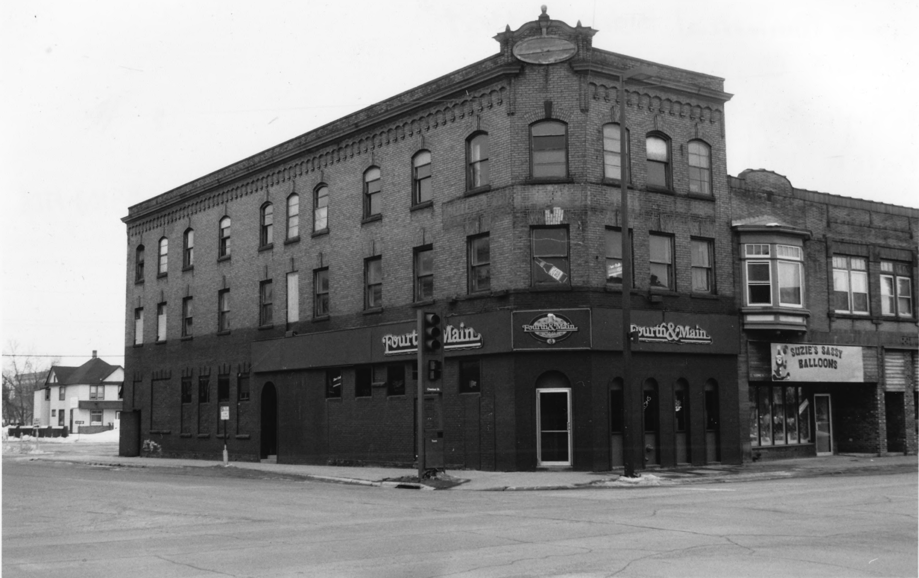
Commercial Building Virginia Commercial Historic District St. Louis Co., MN 012929-3A/4
