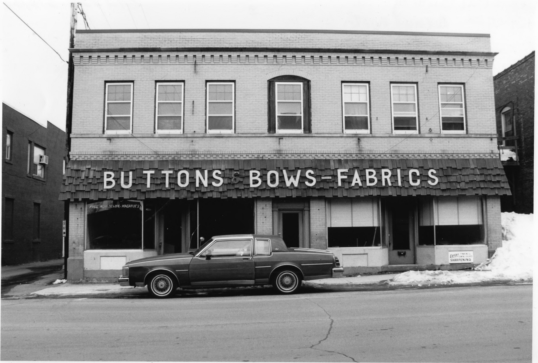
Commercial Building Virginia Commercial Historic District St. Louis Co., Mn 012928 - 21A/22
