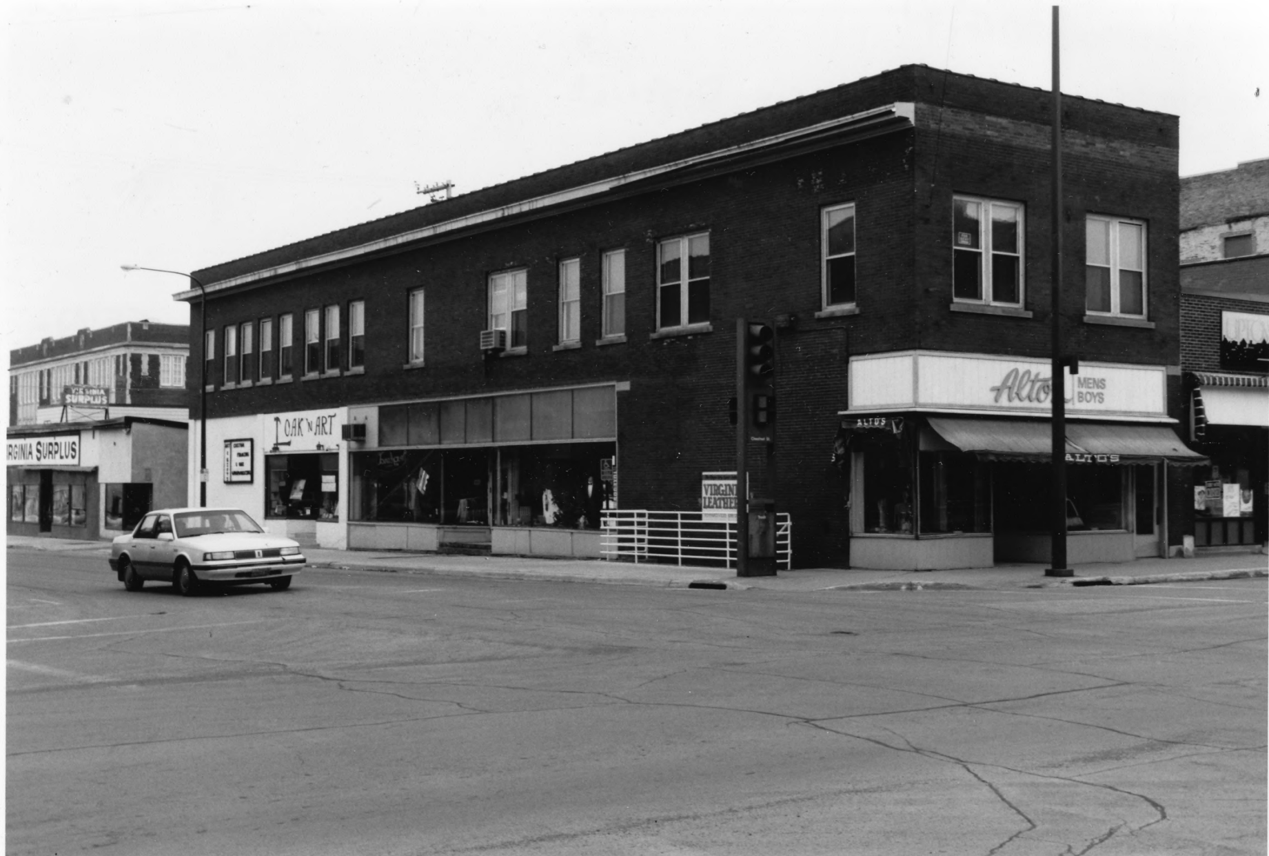
Commercial Building Virginia Commercial Historic District St. Louis Co., Mn 012923-17A18
