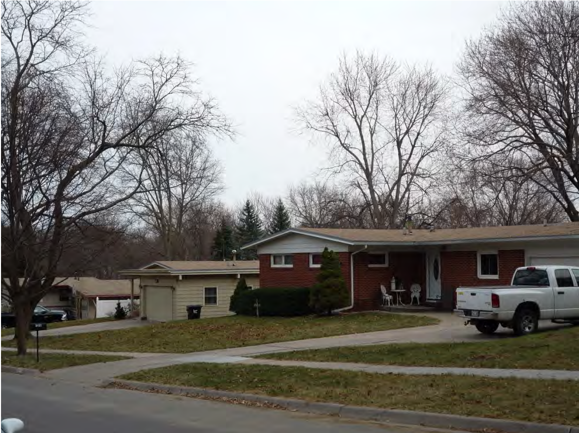
4. Built-up Roofs on Meadowbrook Lane from West (5851 Meadowbrook in foreground, Built in 1956)
