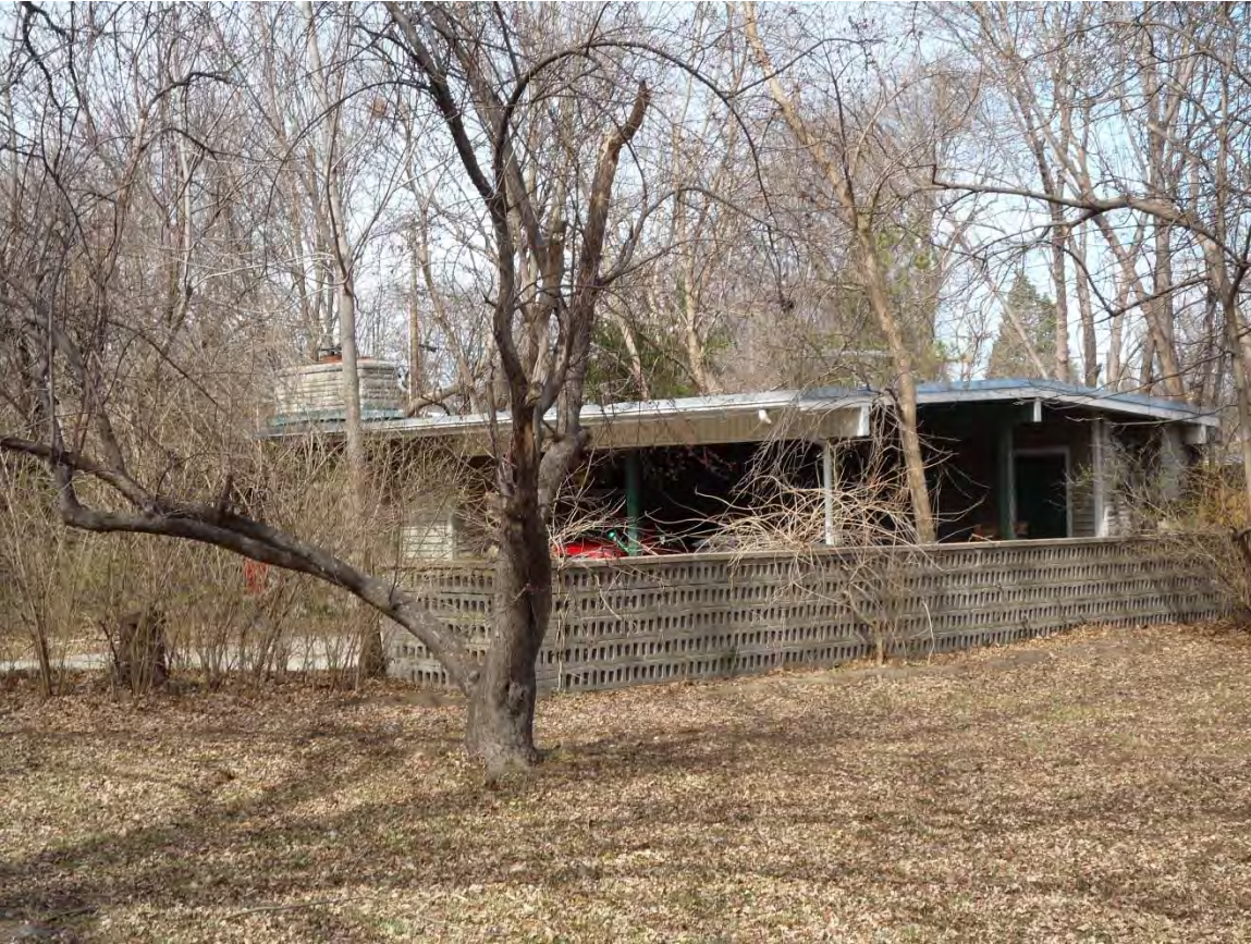
13. Concrete block wall at 930 Dale Drive from Southeast (LC13:G7-021) Built in 1955
