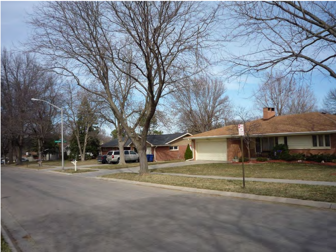
24. Eldon Drive from Southwest (1250 Eldon in foreground, Built by Evans & Evans in 1963)
