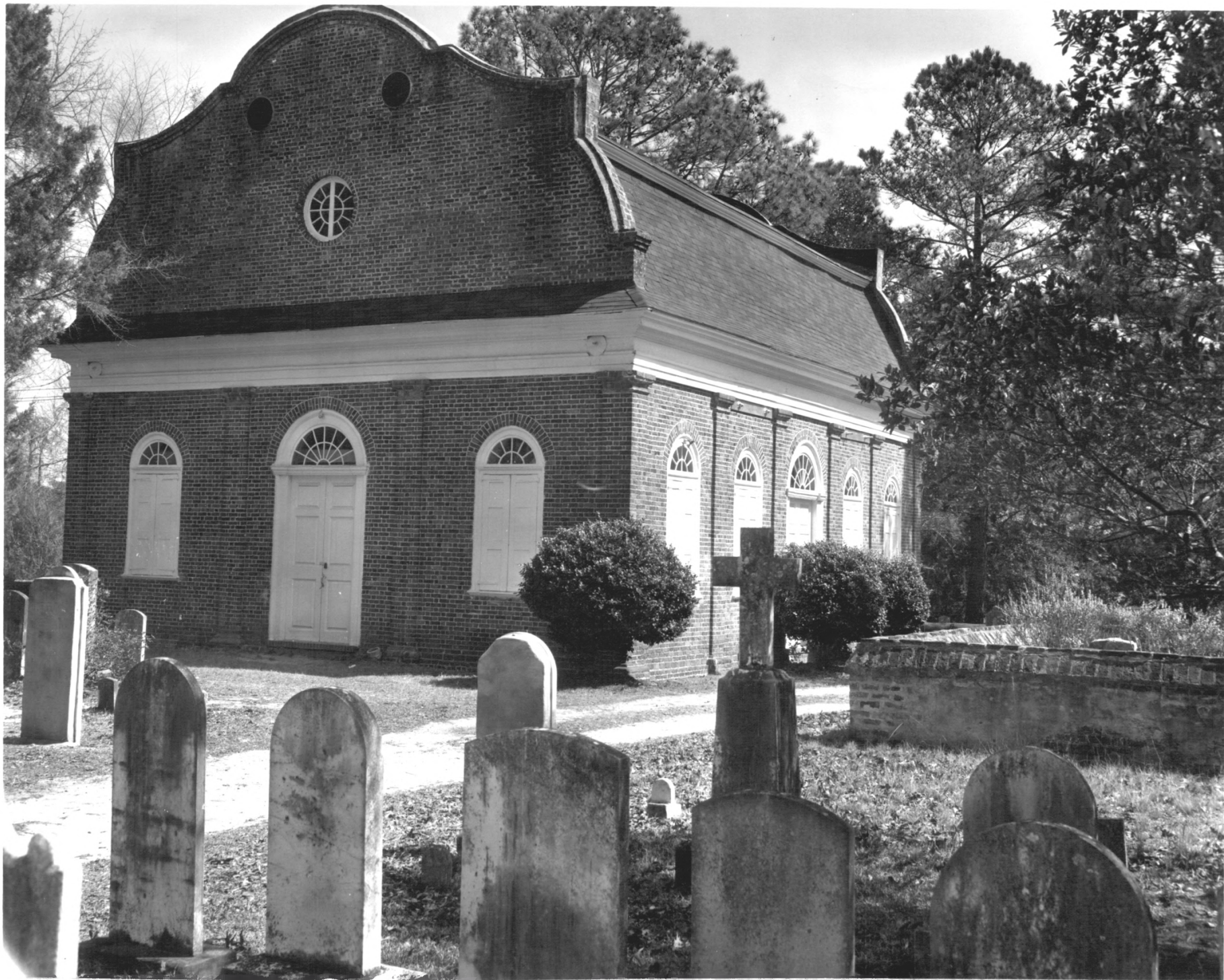
St. Stephen's Church (West or front elevation and south side), St. Stephen, South Carolina. NPS Photo 1969
