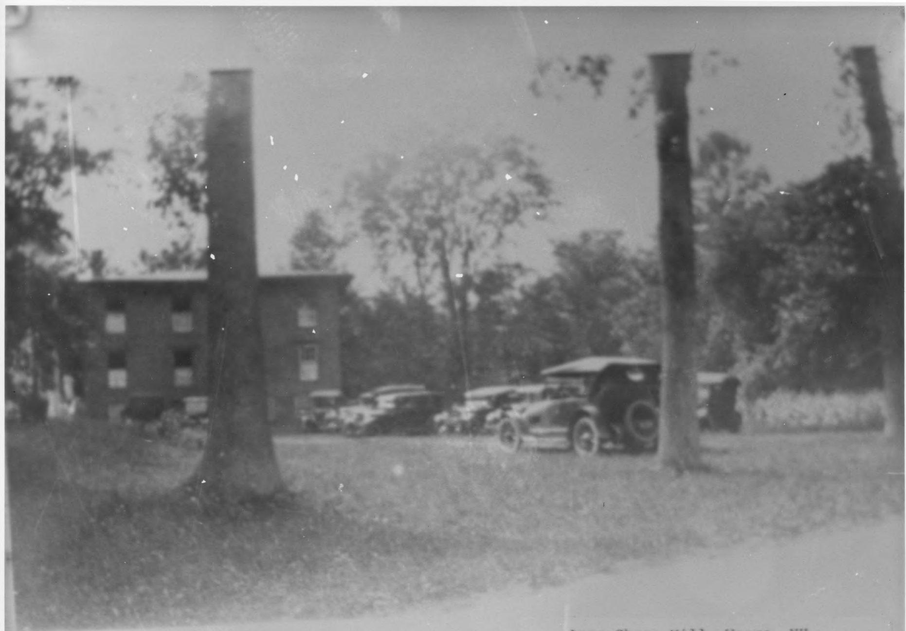
Amos Chase Mill, Weare, NH View looking at east elevation taken 1920's
