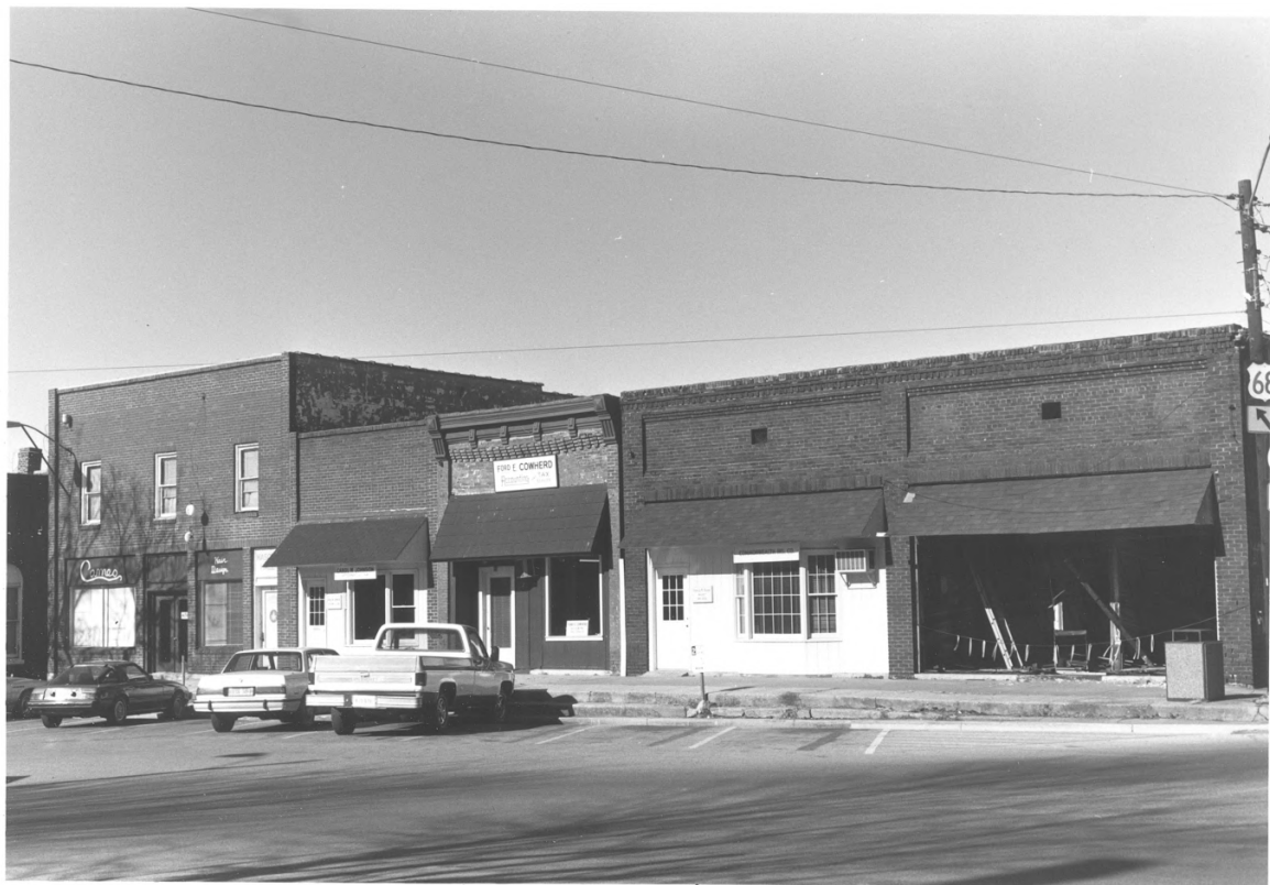
Elkhorn Commercial Historic District, Elkhorn, KY 60-65 Public Square Thomson and Assoc., 2/19/89, View: NW, Photo # 12 of 16
