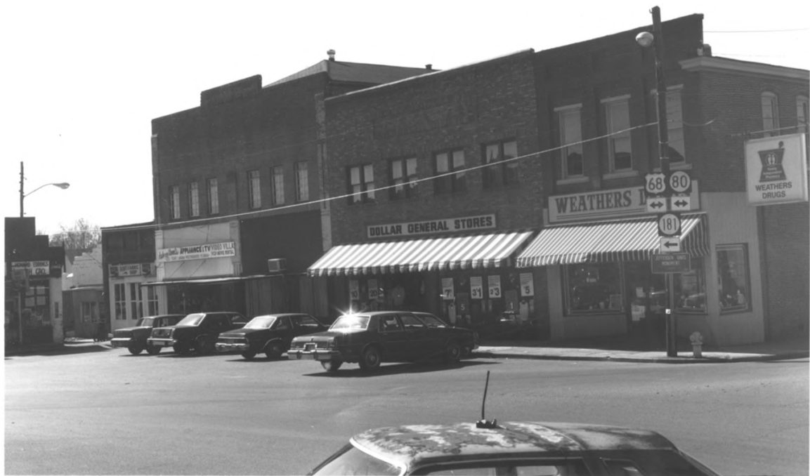
Elkton Commercial Historic District, Elkton, KY, 39-44 Public Square Thomason & Assoc. 2/9/89, View: SW, Photo # 7 of 16
