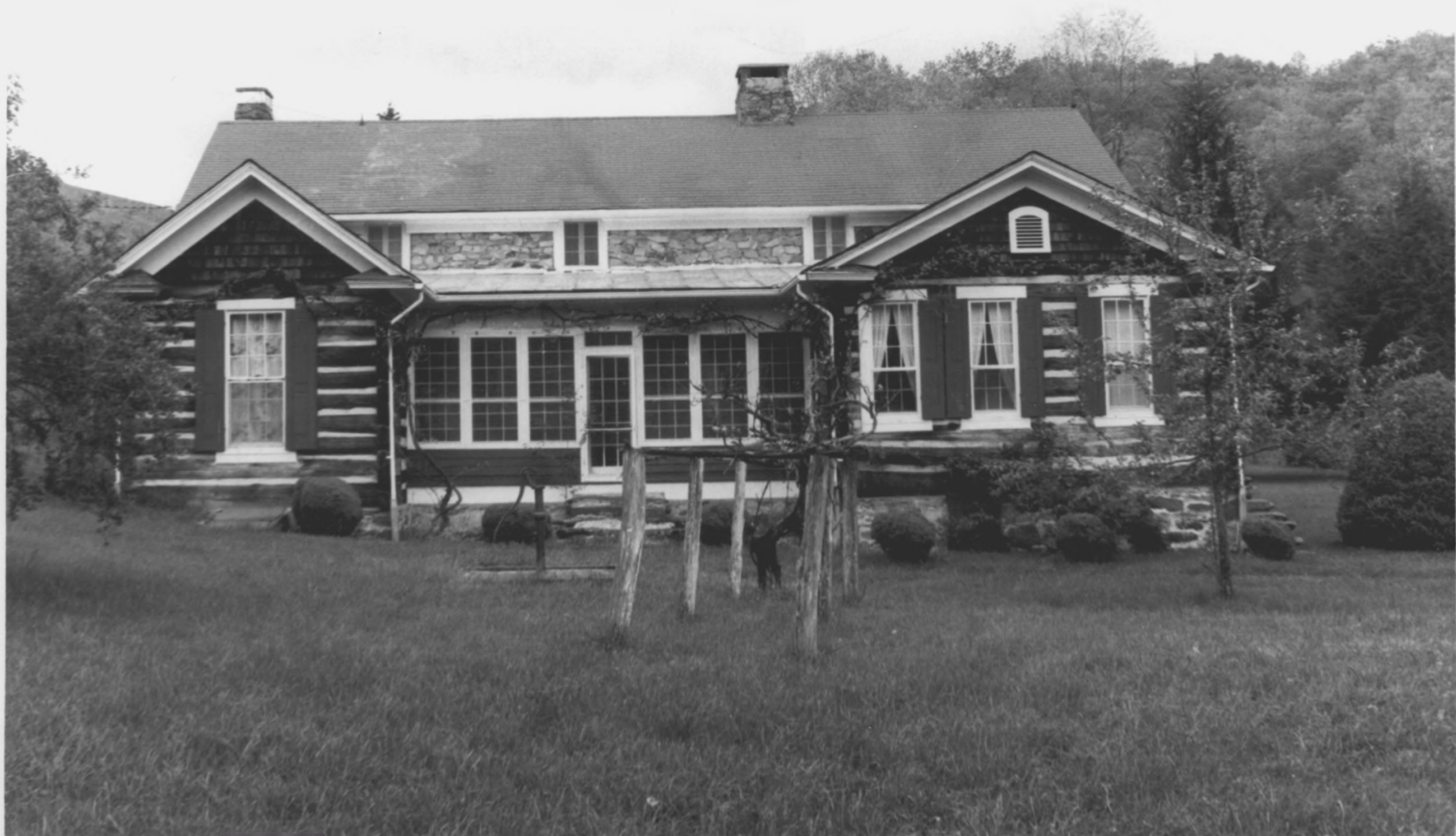
Sherwood Anderson House ("Ripshin Farm"), Trout Dale, Virginia
