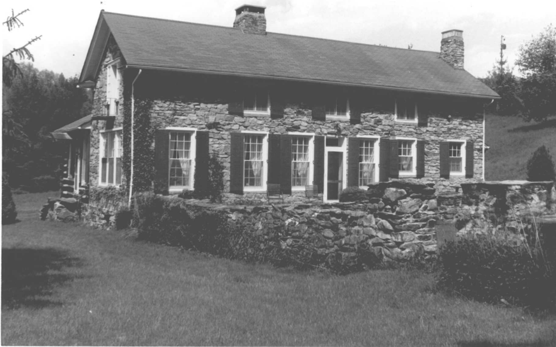
Sherwood Anderson House ("Ripshin Farm"), Trout Dale, Virginia
