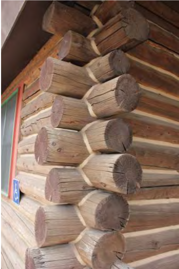
Description of Photograph(s) and number: detail of saddle notching at southwest corner. MT_GlacierCounty_GlacierParkWomen'sClub_0006 of 0011.
