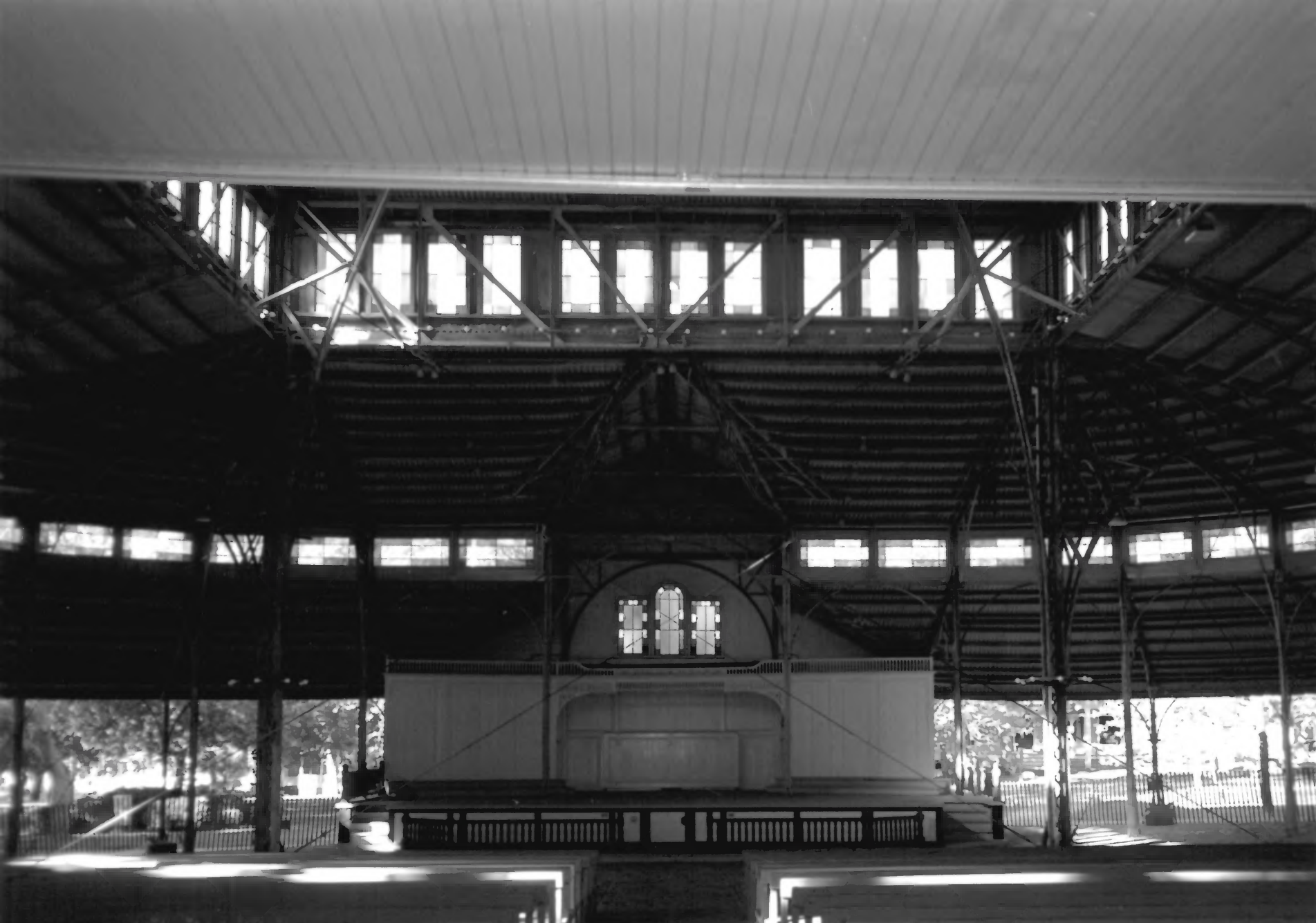
WESLEYAN GROVE Oak Bluffs, Massachusetts Tabernacle interior, from the main (east) entrance Photograph by Sally W. Dagnall, Fall 2002
