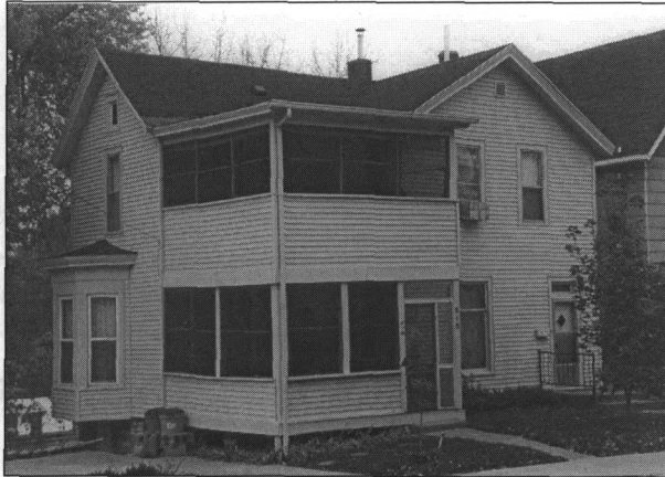
515 Arlington, view northeast (photo by J. Jacobsen, November 2003).
