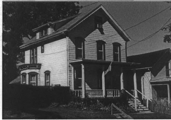
1283 Walnut, view northwest (photo by J. Jacobsen, November 2003).
