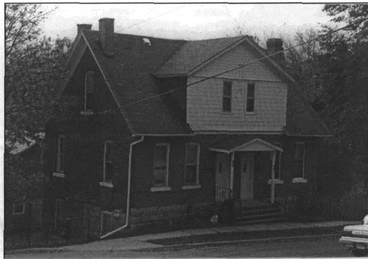
634-36 Jefferson (photo by J. Jacobsen, November 2003).
