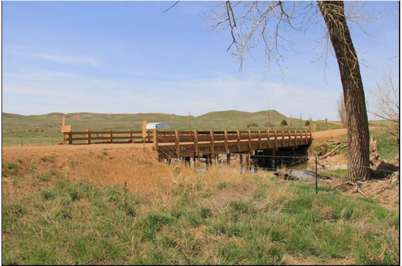
Photo 0003. Cottonwood Creek Bridge. View to the northwest.
