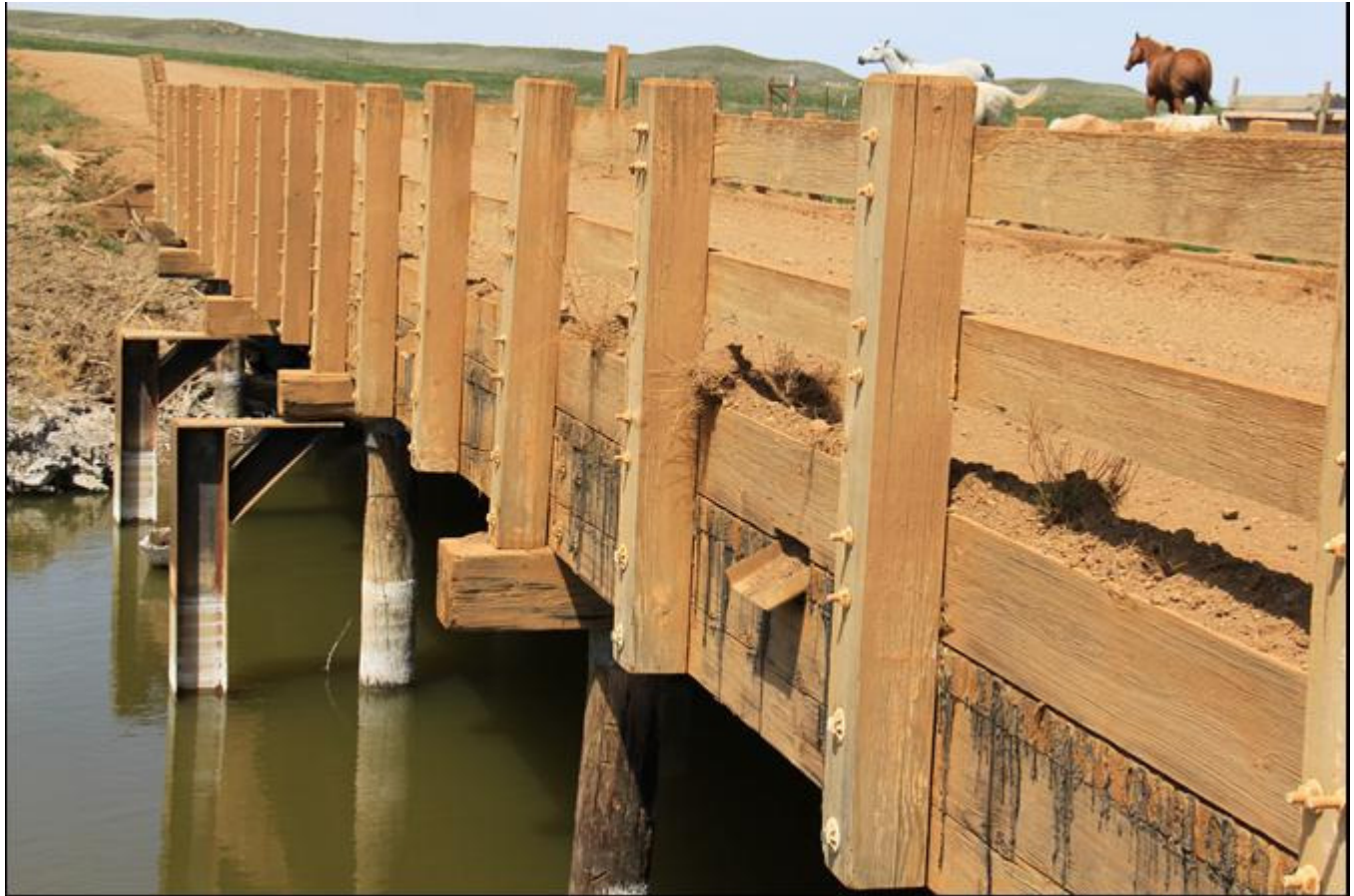
Photo 0006. Detail of Cottonwood Creek Bridge. View to the northeast.
