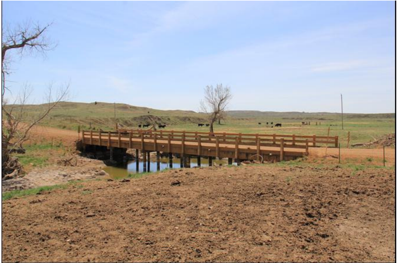
Photo 0004. Cottonwood Creek Bridge. View to the southwest.
