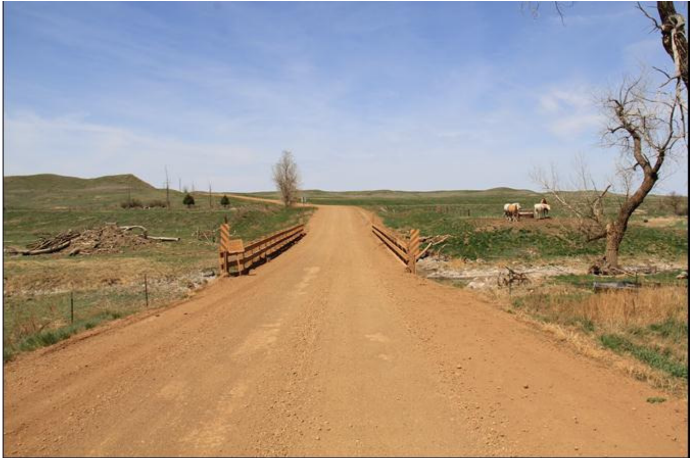
Photo 0002. South portal of Cottonwood Creek Bridge. View to the north.
