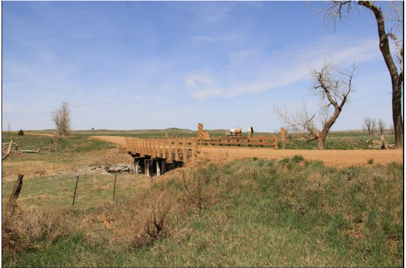
Photo 0001. Cottonwood Creek Bridge. View to the northeast.
