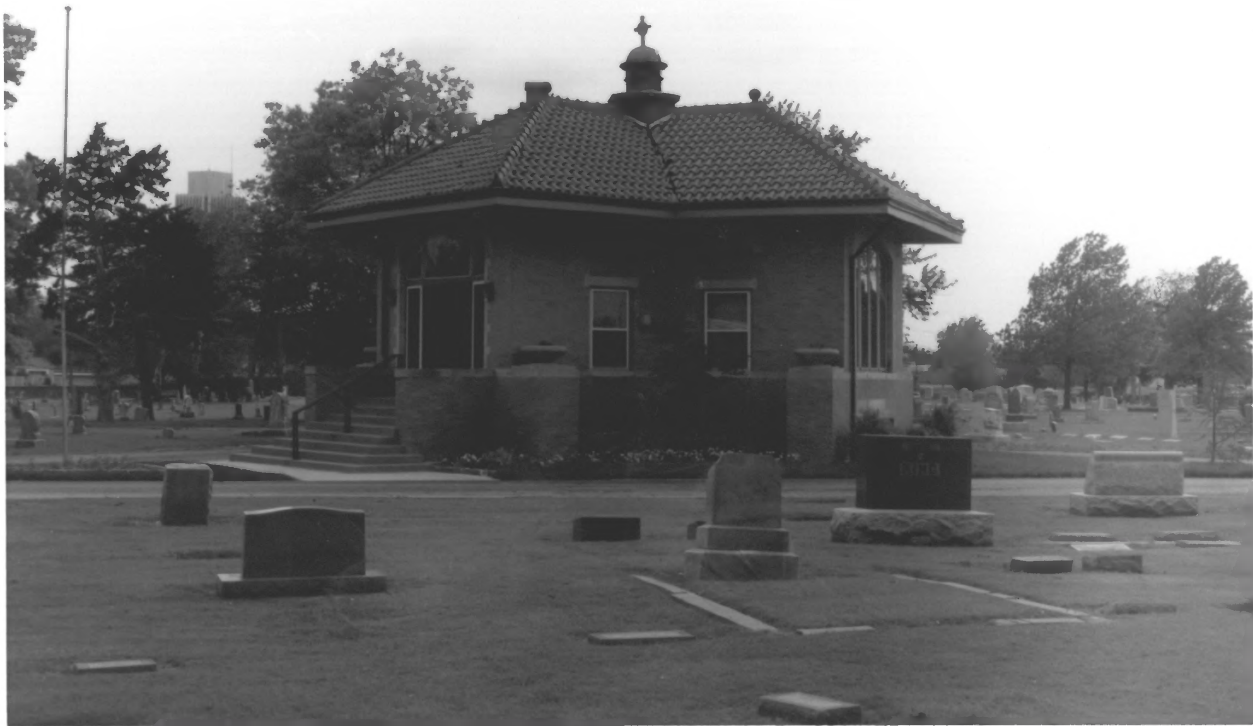
1. FAIRLAWN CEM. CHAPEL, 2700 N. SHARTEL AVE. 2. OKLAHOMA COUNTY, OK. PASCO H.D. #34
