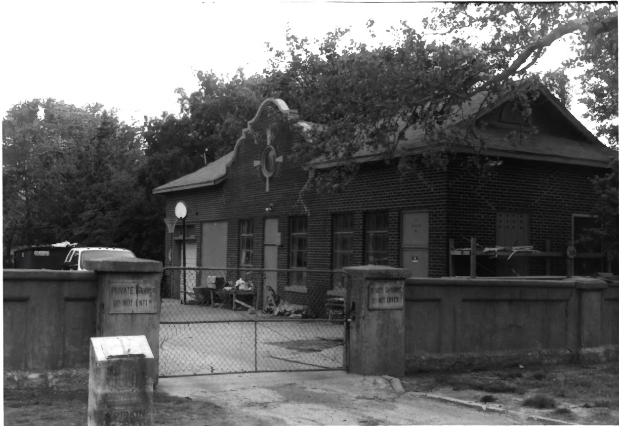
1. FAIRLAWN CEM. MAINT. BLDG., 2700 N. SHARTEL AVE. 2. OKLAHOMA COUNTY, OK. PASEO H.O. #33
