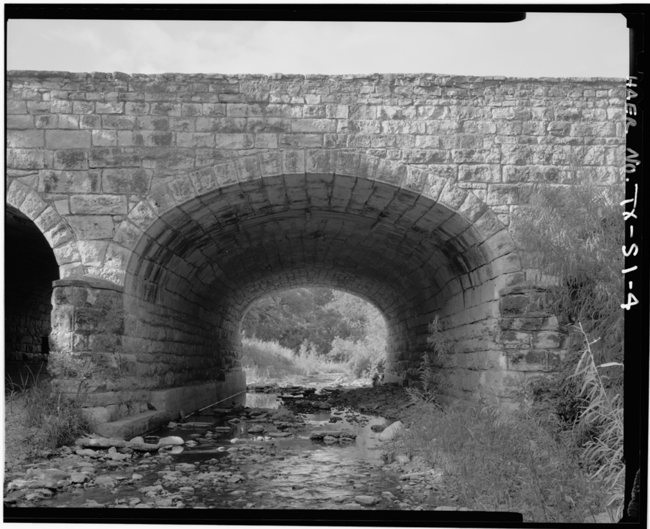
1996 HAER Photo 4 Elevation of central arch, from south
