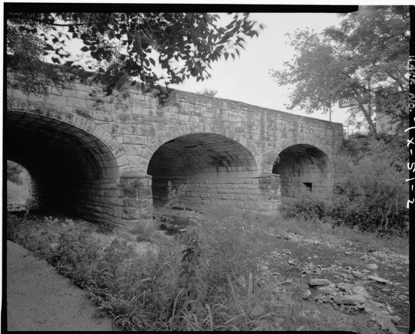
1996 HAER Photo 2 Three-quarters view from southwest
