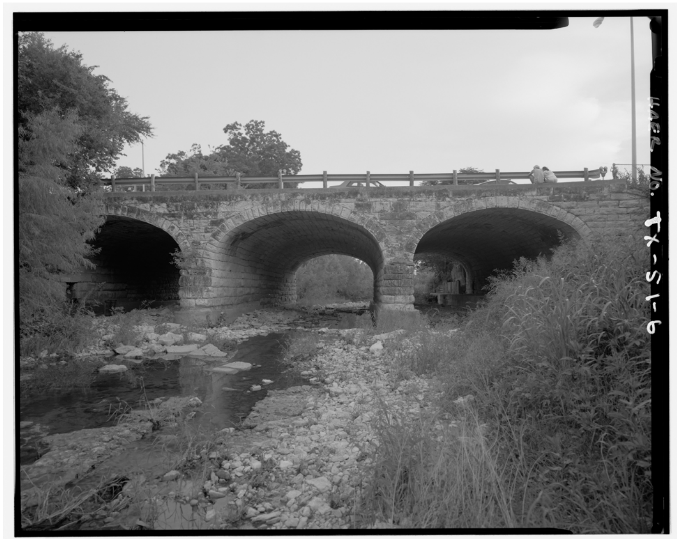
1996 HAER Photo 6 Elevation, from north
