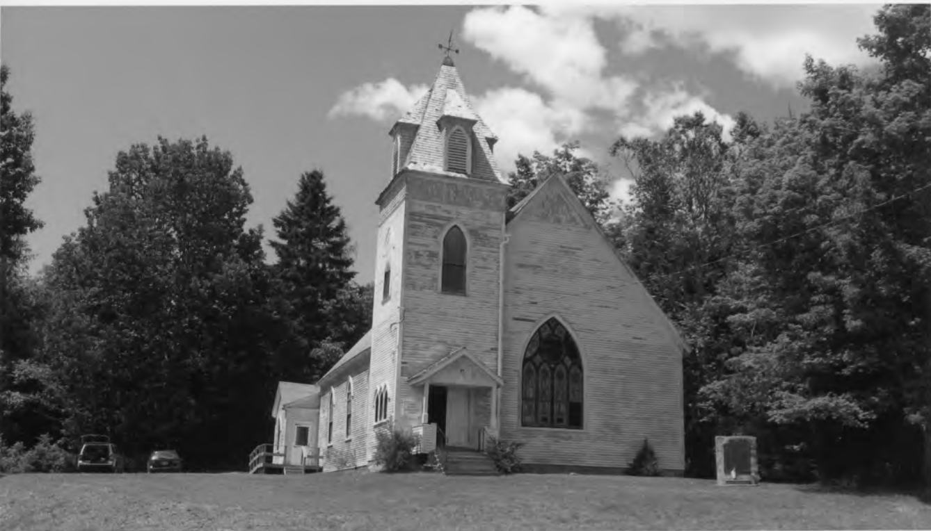
SEWALL MEMORIAL CONGREGATIONAL CHURCH ; WASHINGTON CO., ME
