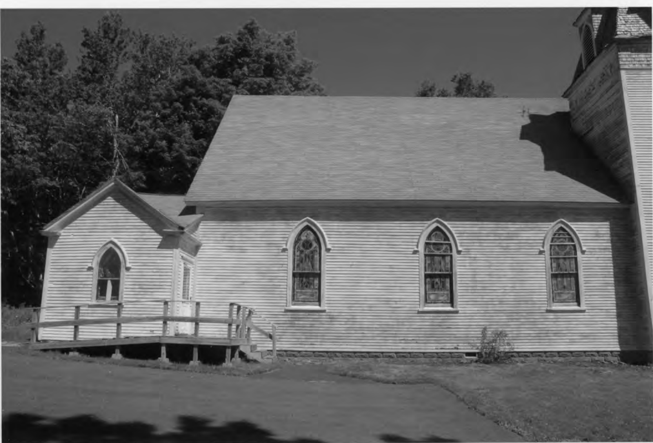
SEWALL MEMORIAL CONGREGATIONAL CHURCH; WASHINGTON CO., ME
