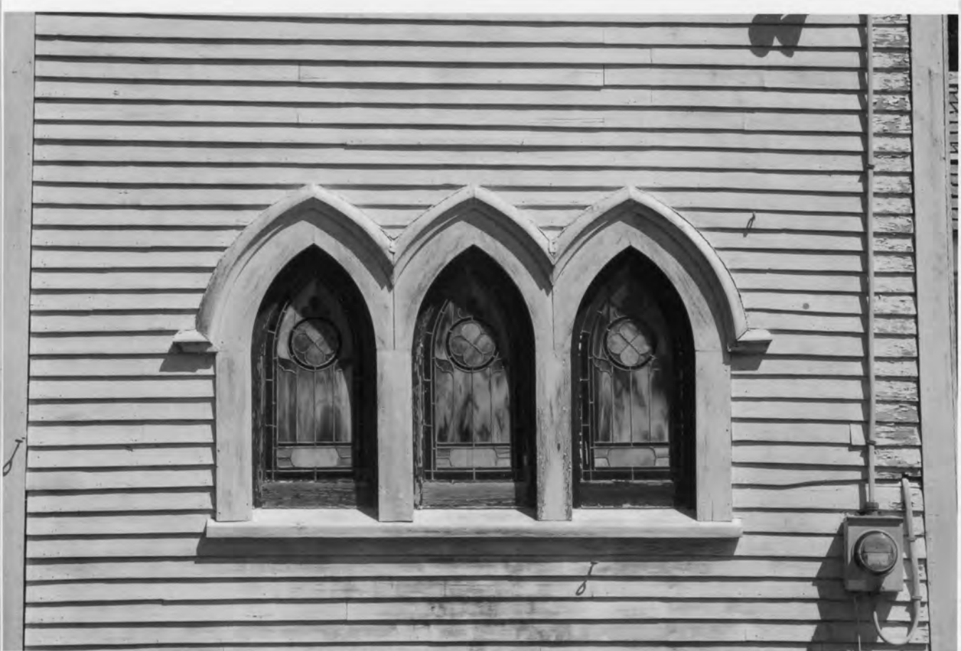
SEWALL MEMORIAL CONGREGATIONAL CHURCH; WASHINGTON CO., ME 30F
