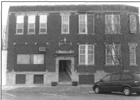
201 South Fifth, view west (Photo by Doug Pierson, January 19, 2005)
