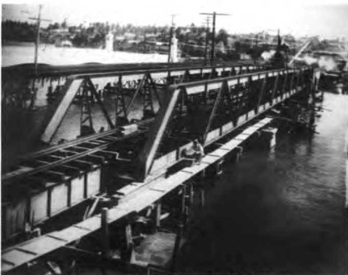
Figure 3. Work on superstructure. December 4, 1931.
