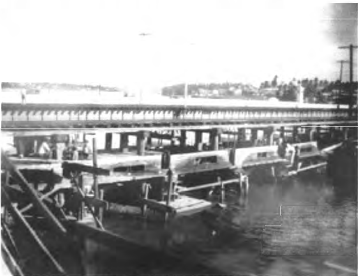
Figure 7. Placement of precast concrete arcade in northern section. January 13, 1932.
