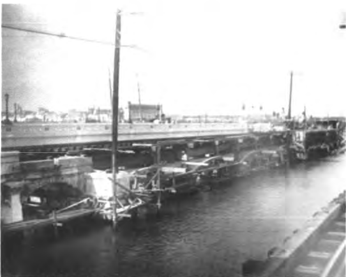
Figure 11. View of work on central arcade. February 1, 1932.
