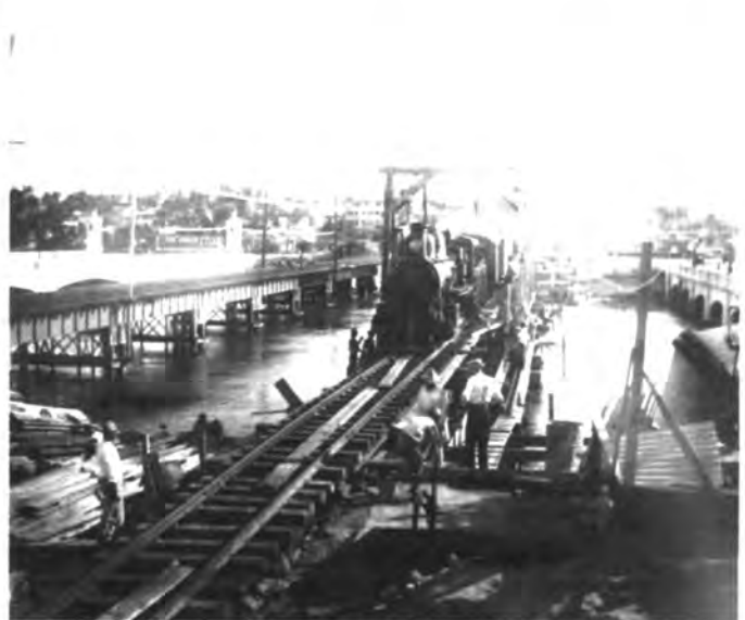
Figure 6. Work on the abutments. January 5, 1932.
