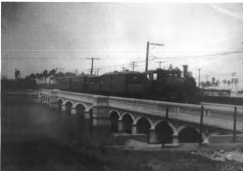
Figure 18. View of Completed bridge. April 2, 1932.
