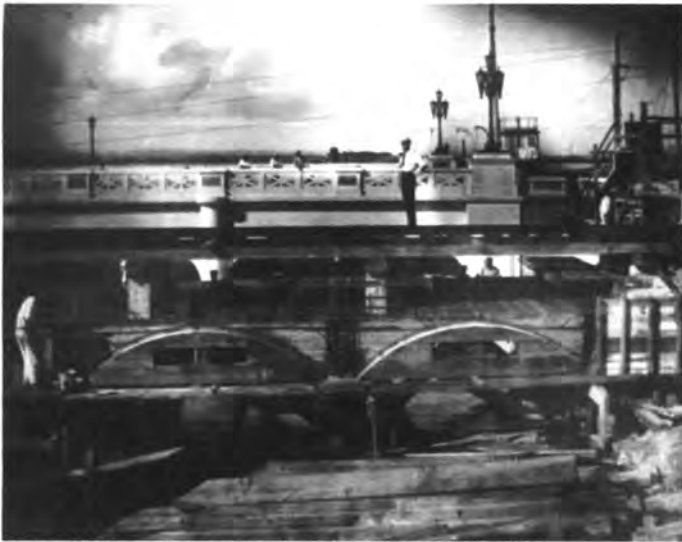
Figure 9. Close up of precast arches. January 21, 1932.
