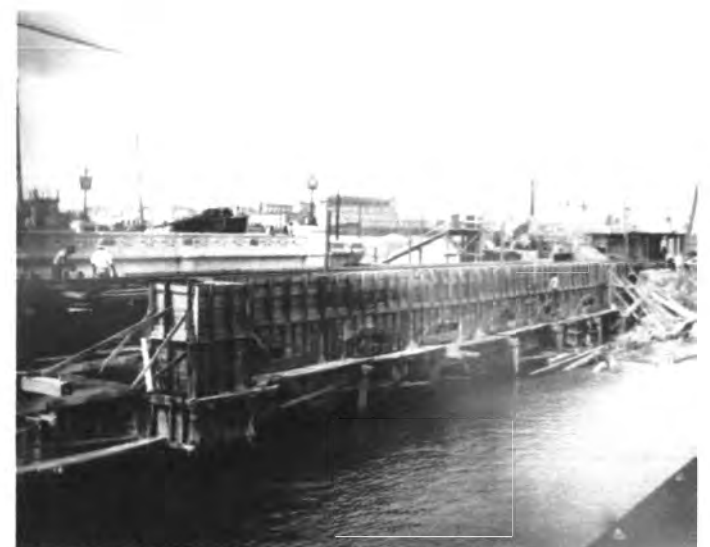
Figure 12. View of work completed on central arcade. Feb. 1, 1932.
