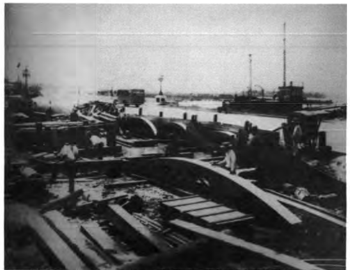
Figure 2. Precast arches ready to insert. December 4, 1931.
