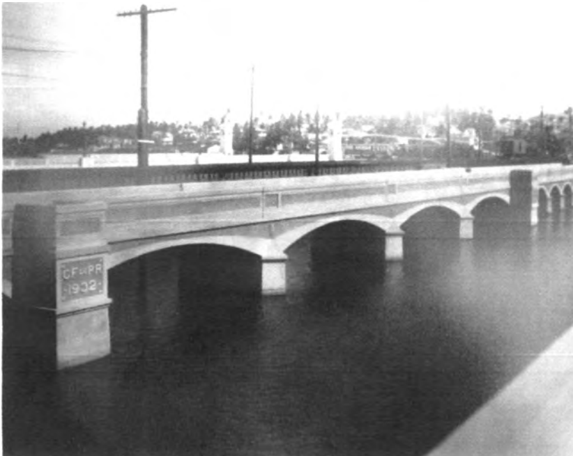
Figure 17. View of finished central arcade. April 2, 1932.
