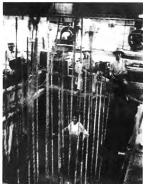
Figure 4. Rod placement for pouring cement for the foundations. Dec. 11, 1931
