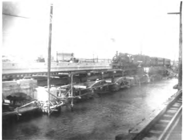
Figure 10. Train crossing central arcade. Feb. 1, 1932.
