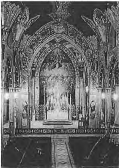
Figure 30. Church Interior ca 1950s. Photographer unknown. 57
