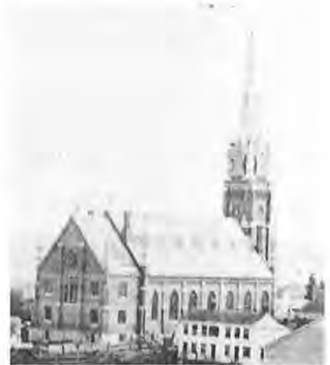
Figure 12. St. Mary's Church ca 1867. West Facade. 11
