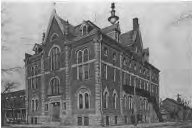
Figure 21. St. Mary's Casino as originally constructed. Date unknown (pre 1959). 20
