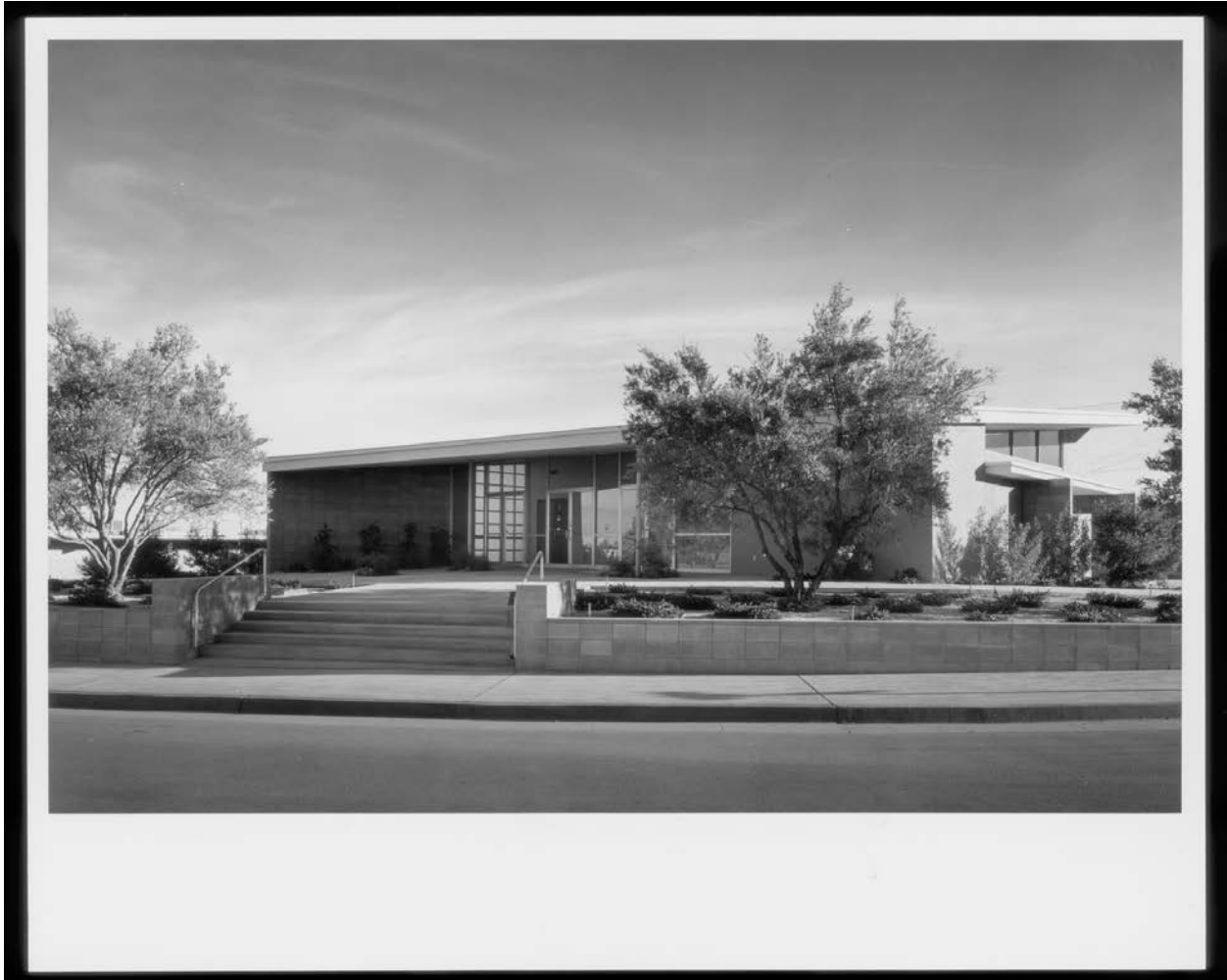
Figure 2. Primary (north) and west elevations, looking southeast 1959.
