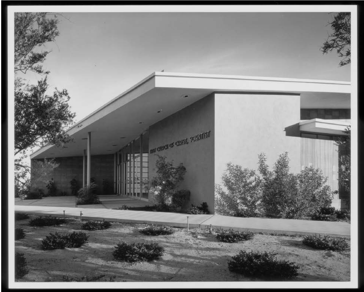
Figure 3. North and west elevations, looking southeast, 1959.
