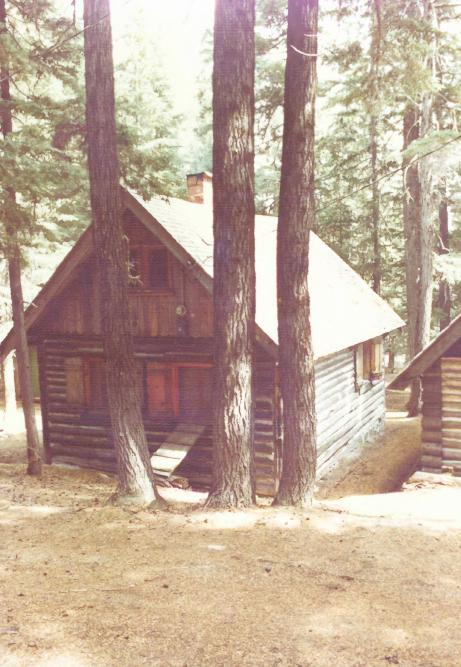
Series B 6 of 6 Cabin #10, West Group West and south elevations, showing method of siting on an ascending grade.
