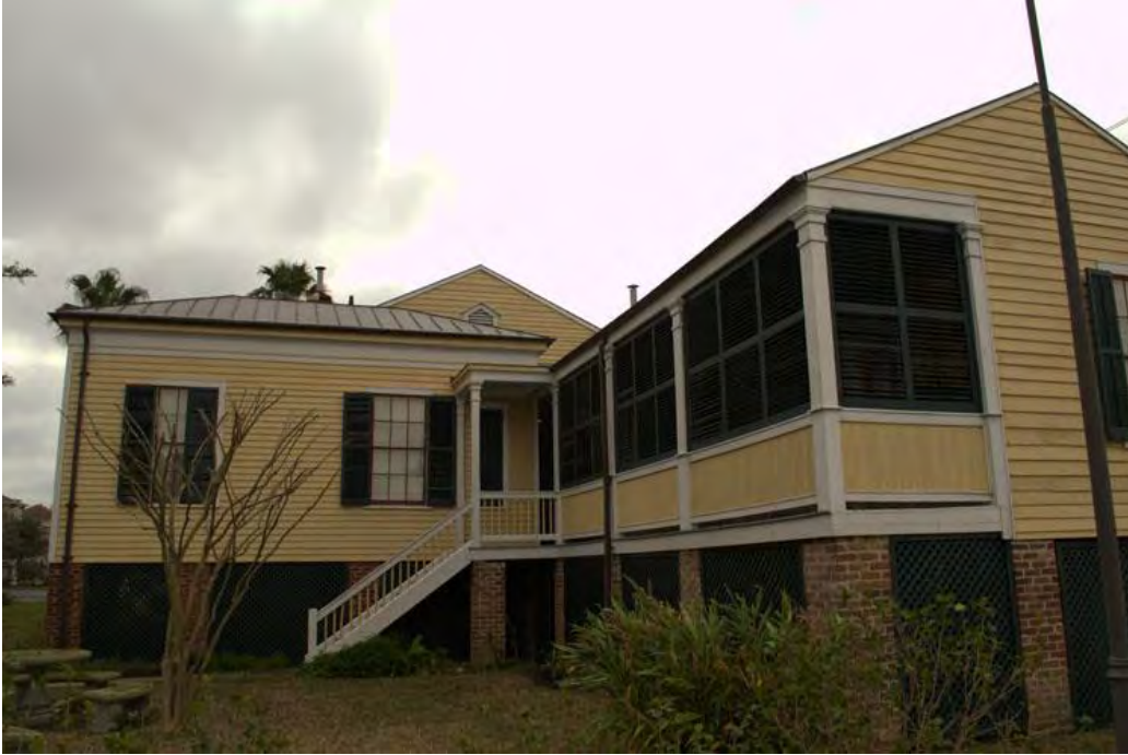
Photo 5: North elevation of ell, rear addition breezeway; camera facing southwest
