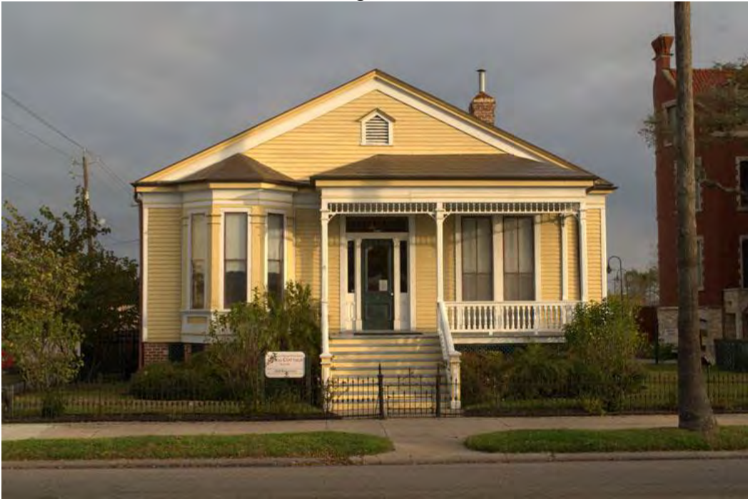
Photo 1: South elevation; camera facing north
