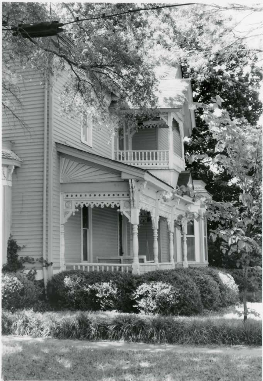
MIDTOWN HISTORIC DISTRICT, CORINTH, ALABAMA CO. MS PHOTO 11 OF 31
