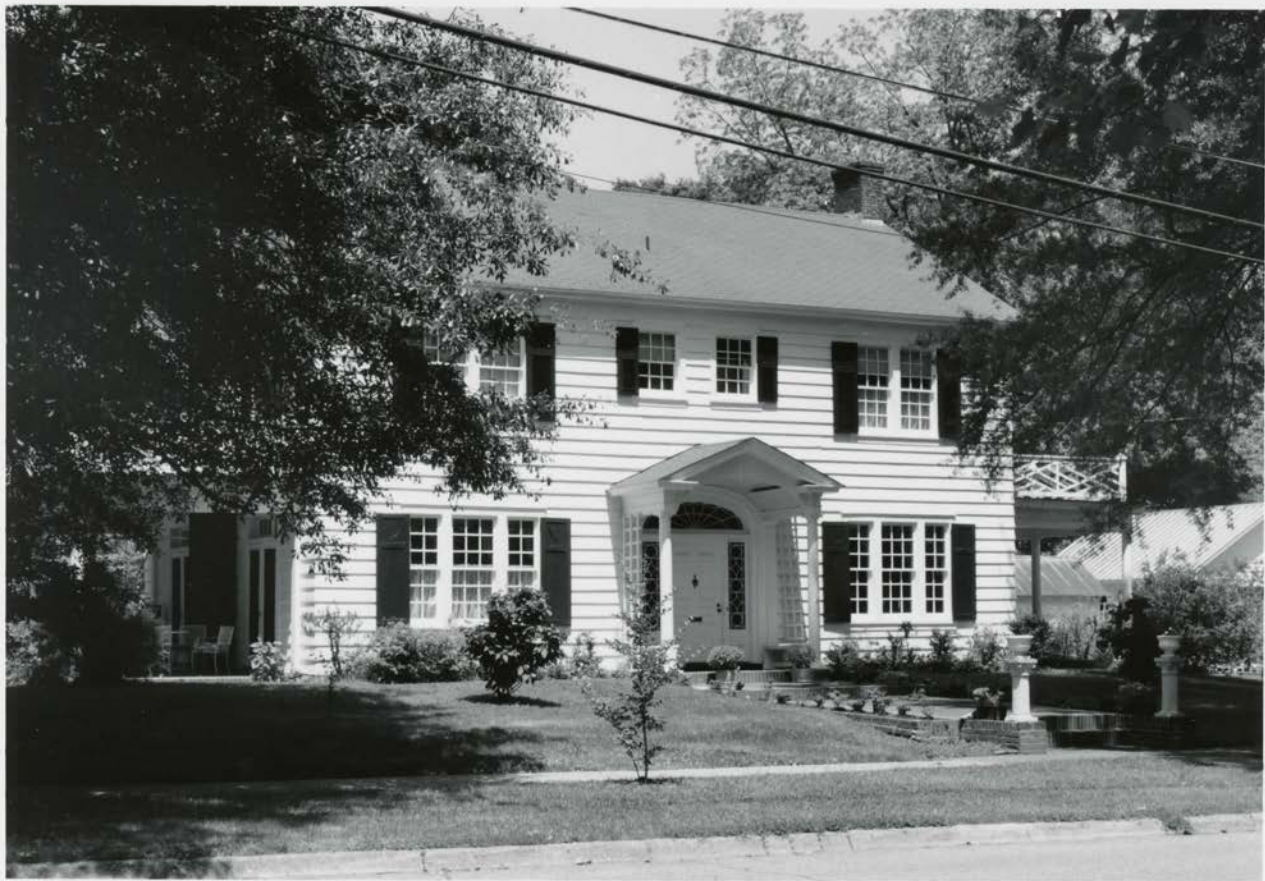
MIDTOWN HISTORIC DISTRICT, CORNICH, SLOORN CO., MS
