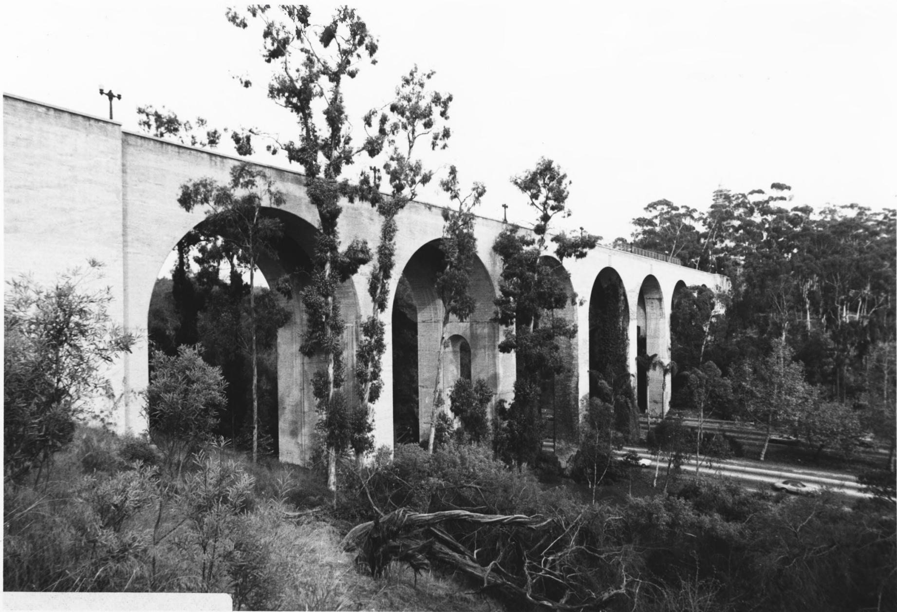
Cabrillo Bridge View from the South
