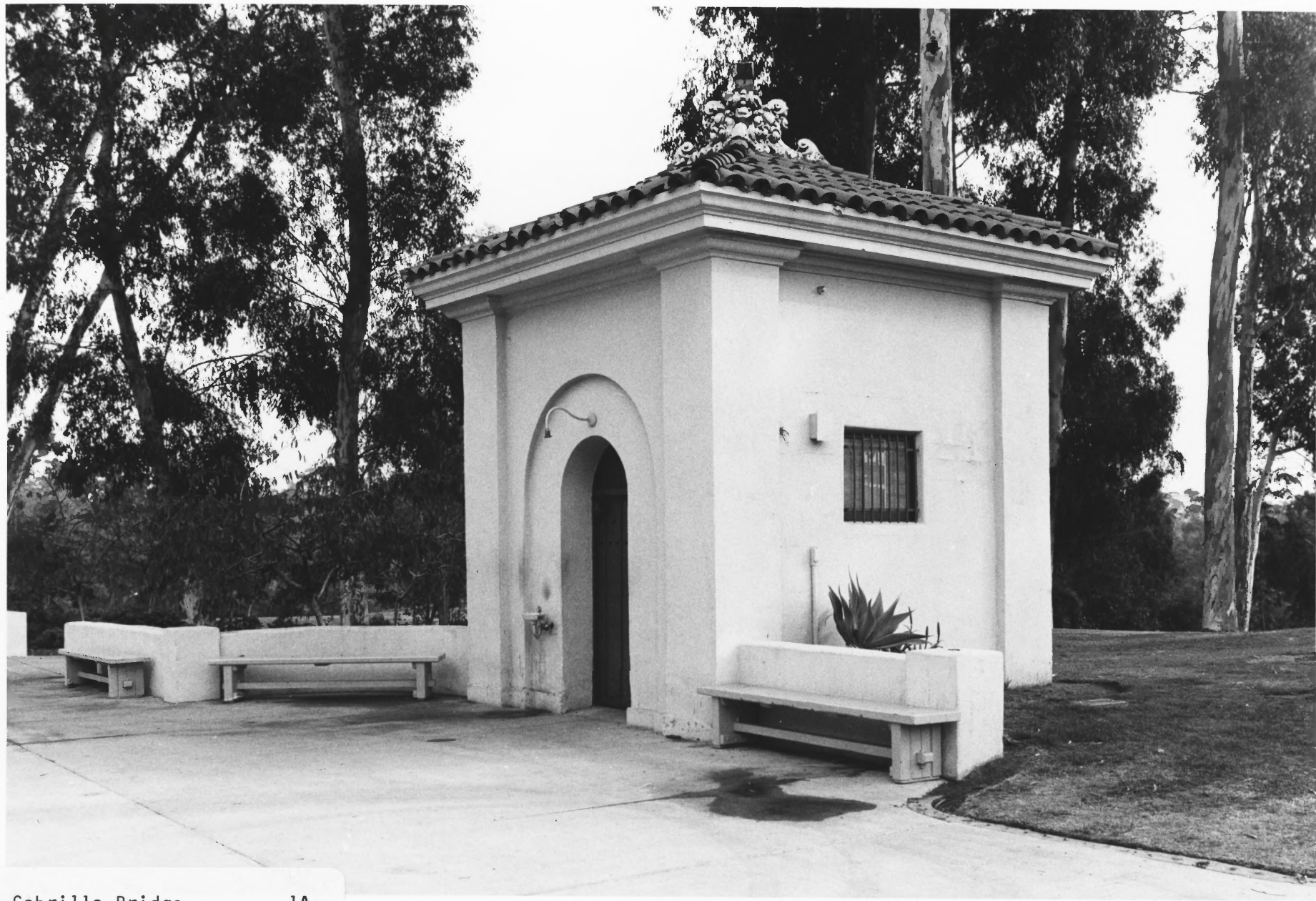
Cabrillo Bridge 1A West Approach - Guardhouse on South Side of El Prado
