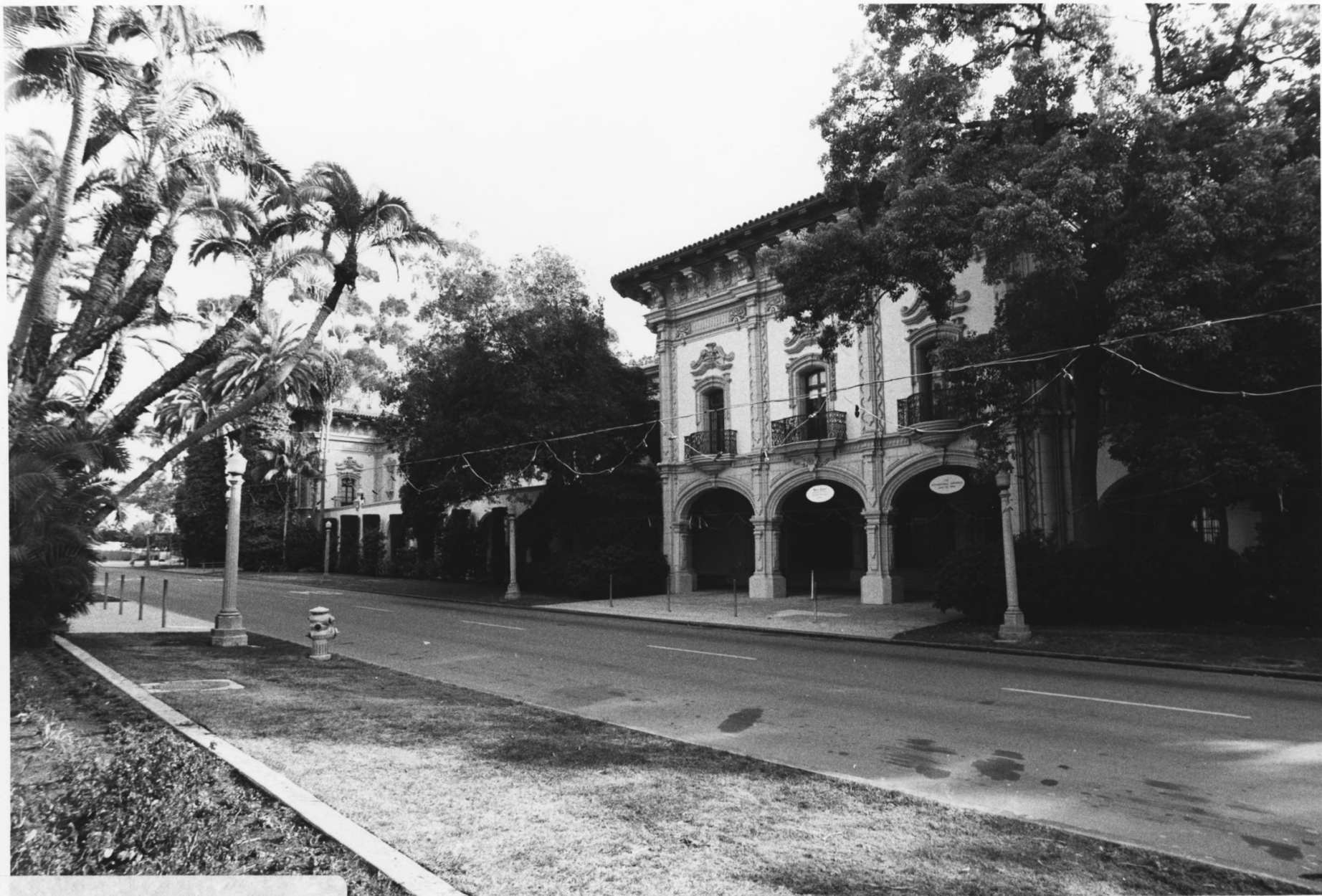
ELECTRICAL BUILDING View from North
