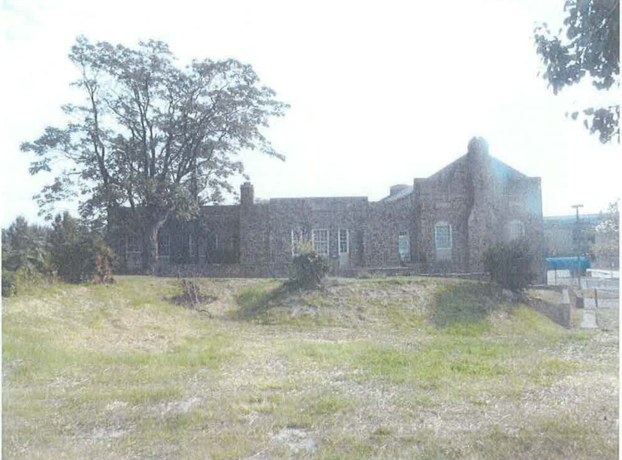
MD_BaltimoreCity_MSUMemorialChapel_0005.tif South Elevation, 06/29/2012 5 of 7
