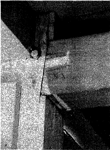
Fig 4. Mortise and tenon joint identified by roman numbers for its assembly
