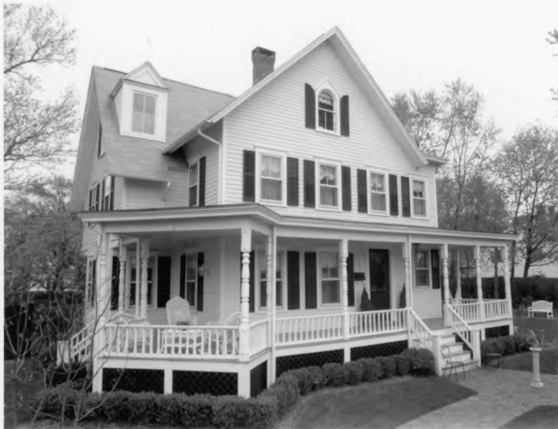
Photo 8. 86 Rowayton Avenue: Capt. John Monsell House, c.1885 Norwalk, Fairfield County, Connecticut view southeast, September 7, 2008 Rick Pank
