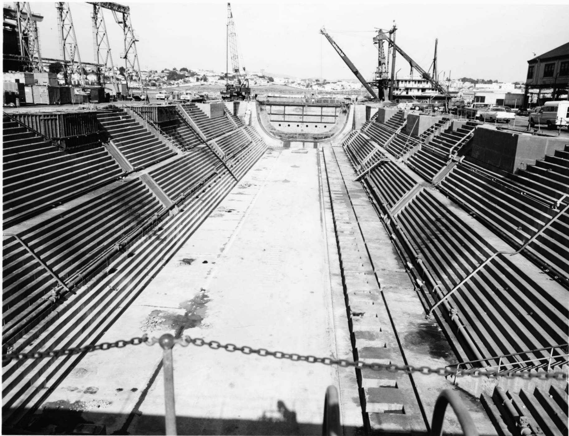
Mare Island Naval Shipyard, Vallejo, California; Drydock 1.
