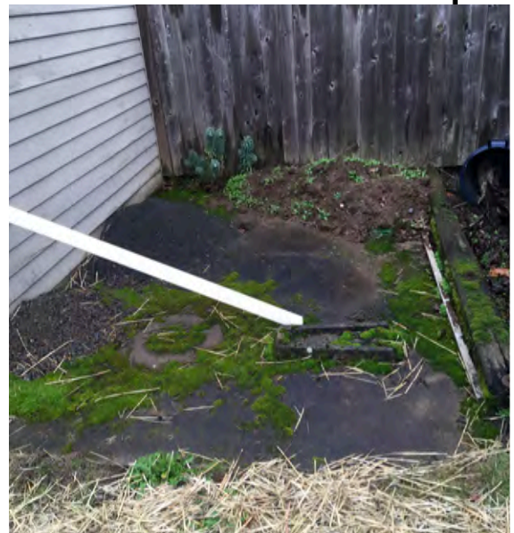
Figure 7: Concrete pad and bolted timber behind garage
