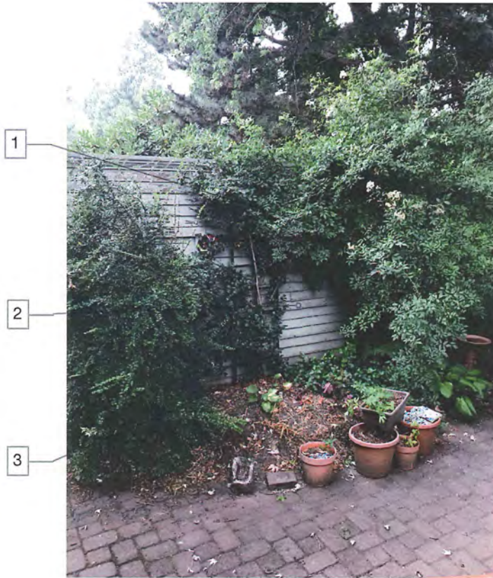
GARAGE WEST FACADE
