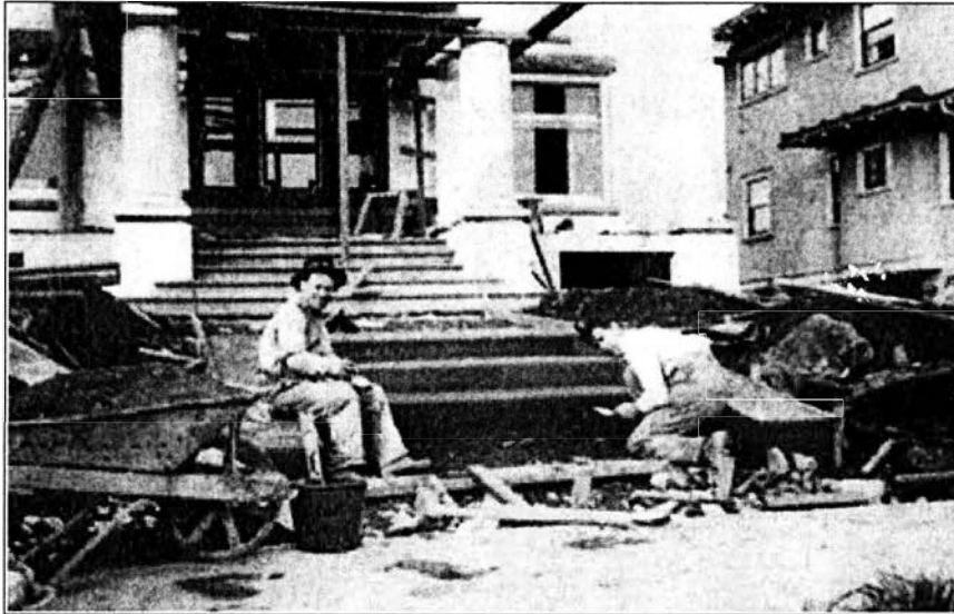
Figure 20: T. L. Seufert residence (2009 N.E. Brazee) attributed to architect Ellis Lawrence, c. 1910. Image from Residential Portland, 1911 , published by the News Syndicate, original copy from the collection of Jim Heuer and Robert Mercer.
