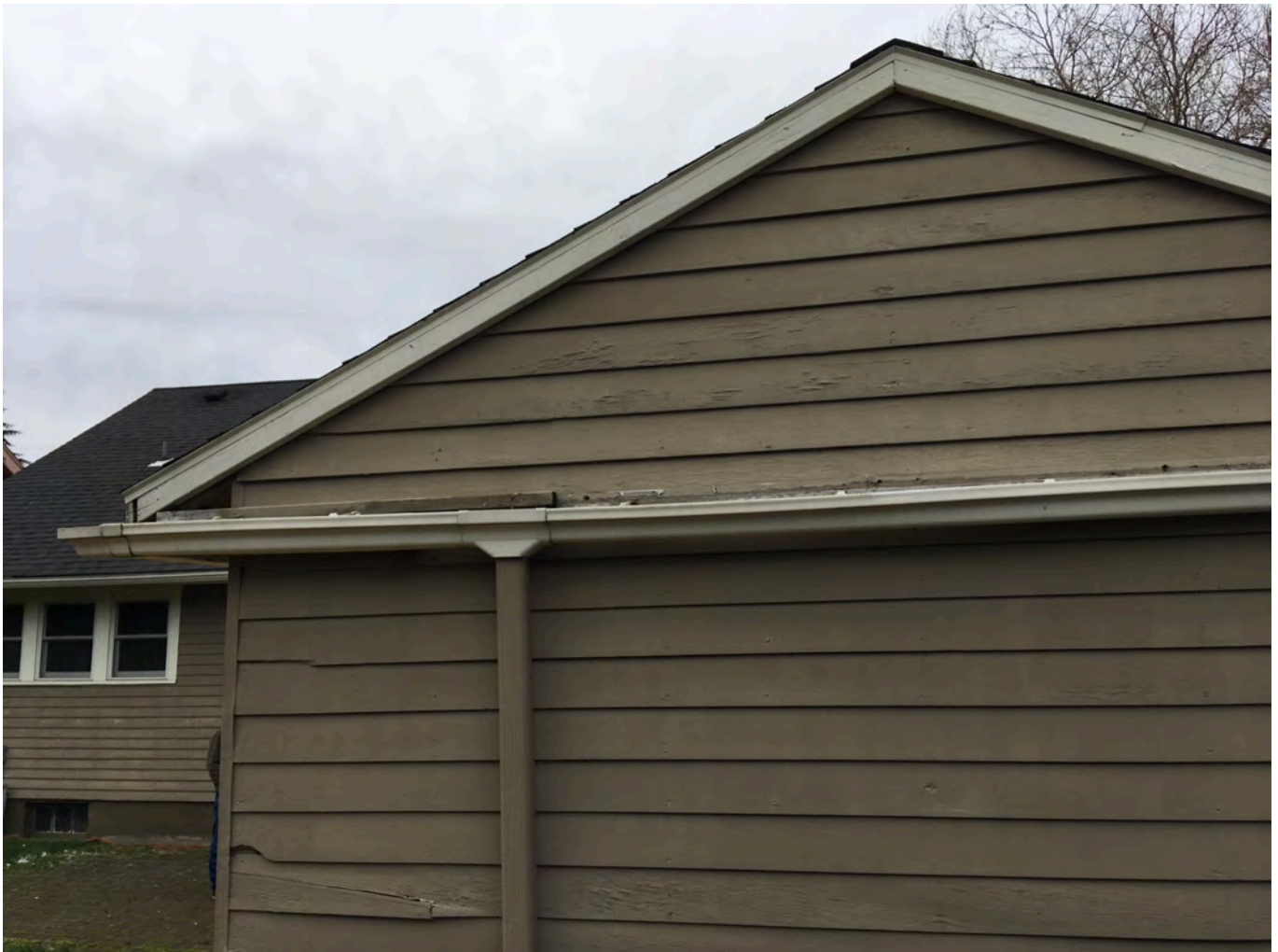
Figure 4: Partial rear/East elevation
