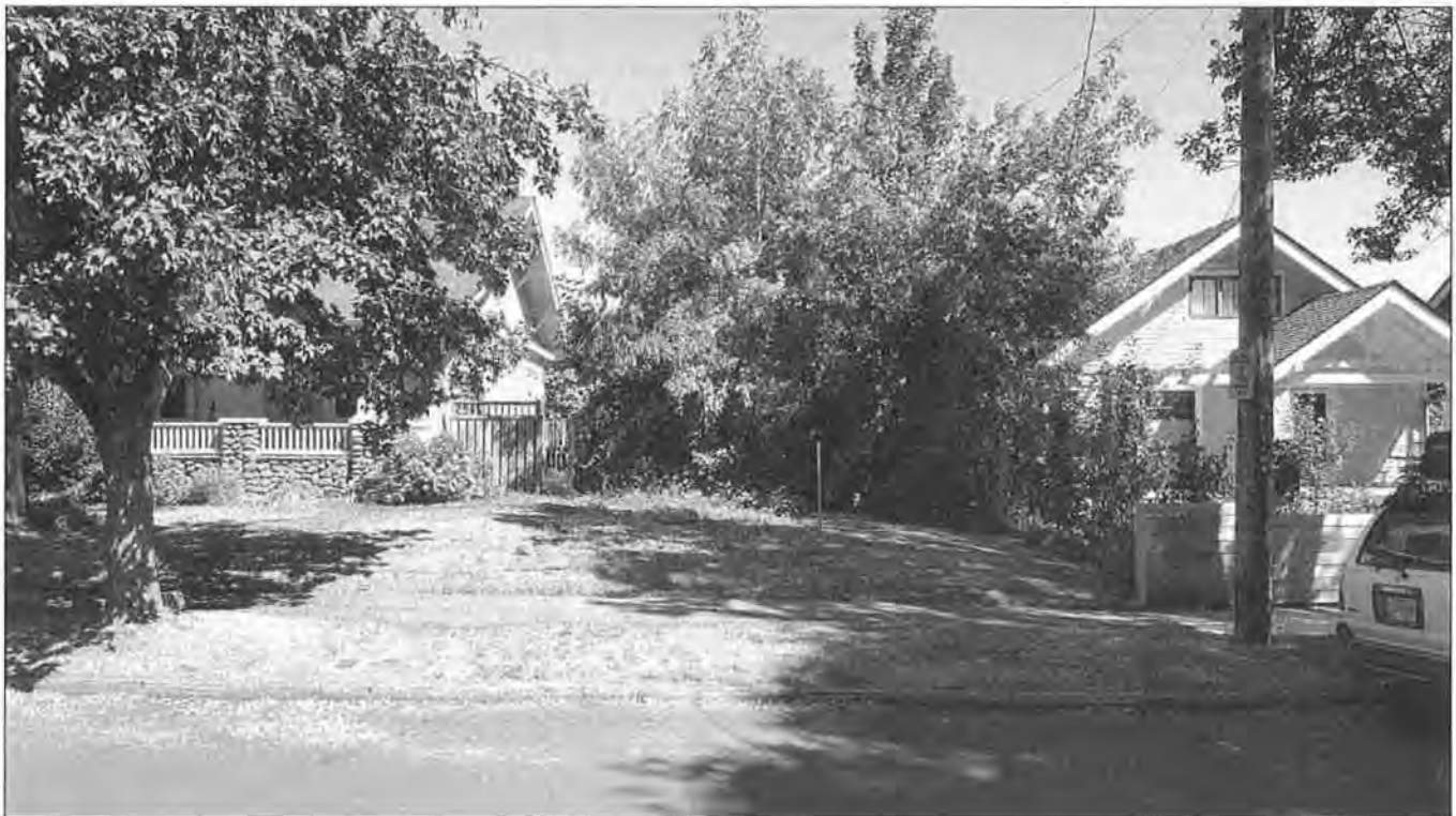
2240 NE 11 th Ave, (building to left) west (left) and south (right) facades, facing east
