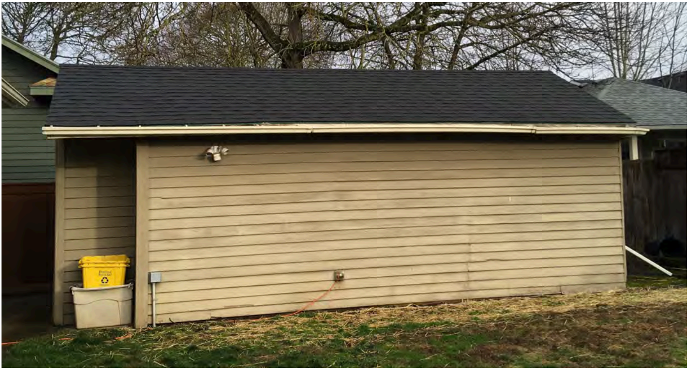
Figure 3: South elevation of existing garage
