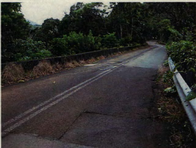
Figures 17 and 18: "Hogsback", near Mile Marker 4.0 Basalt (lava rock) retaining wall at Hogsback.
