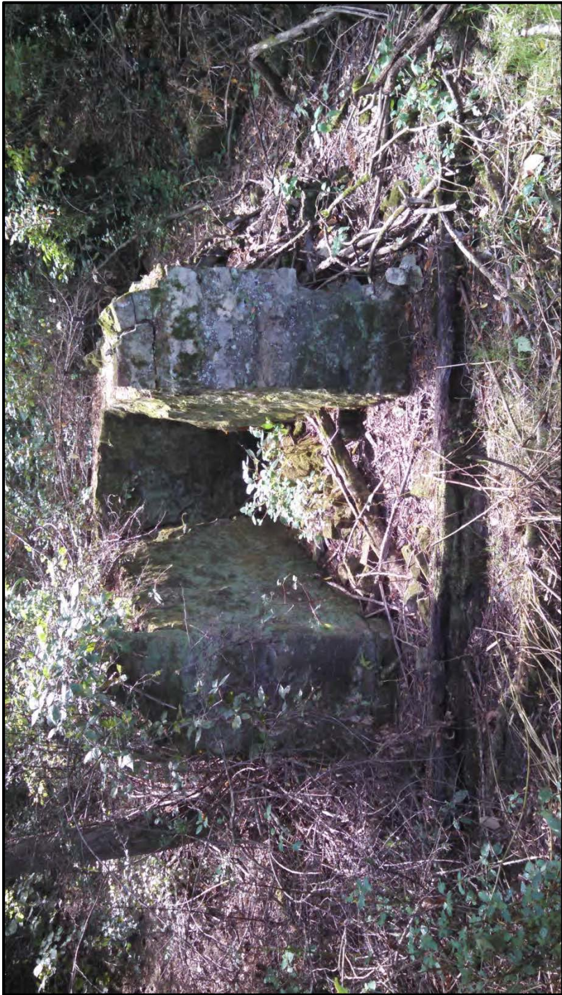
Figure 26. Spring House, Masonry walls.
