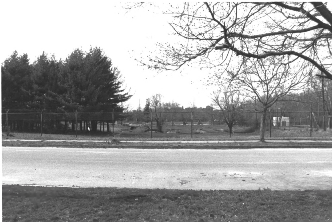
General view of site and Serpentine Canal from Liverpool Avenue. Atlantic County, NJ (# 14 of 40); Dr. Smith's Sanitarium Site, Egg Harbor City.
