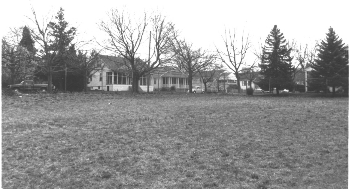
Houses along Liverpool Ave. from canal site, Dr. Smith's Sanitarium Site, Atlantic County, NJ (# 13 of 14) Egg Harbor Site
