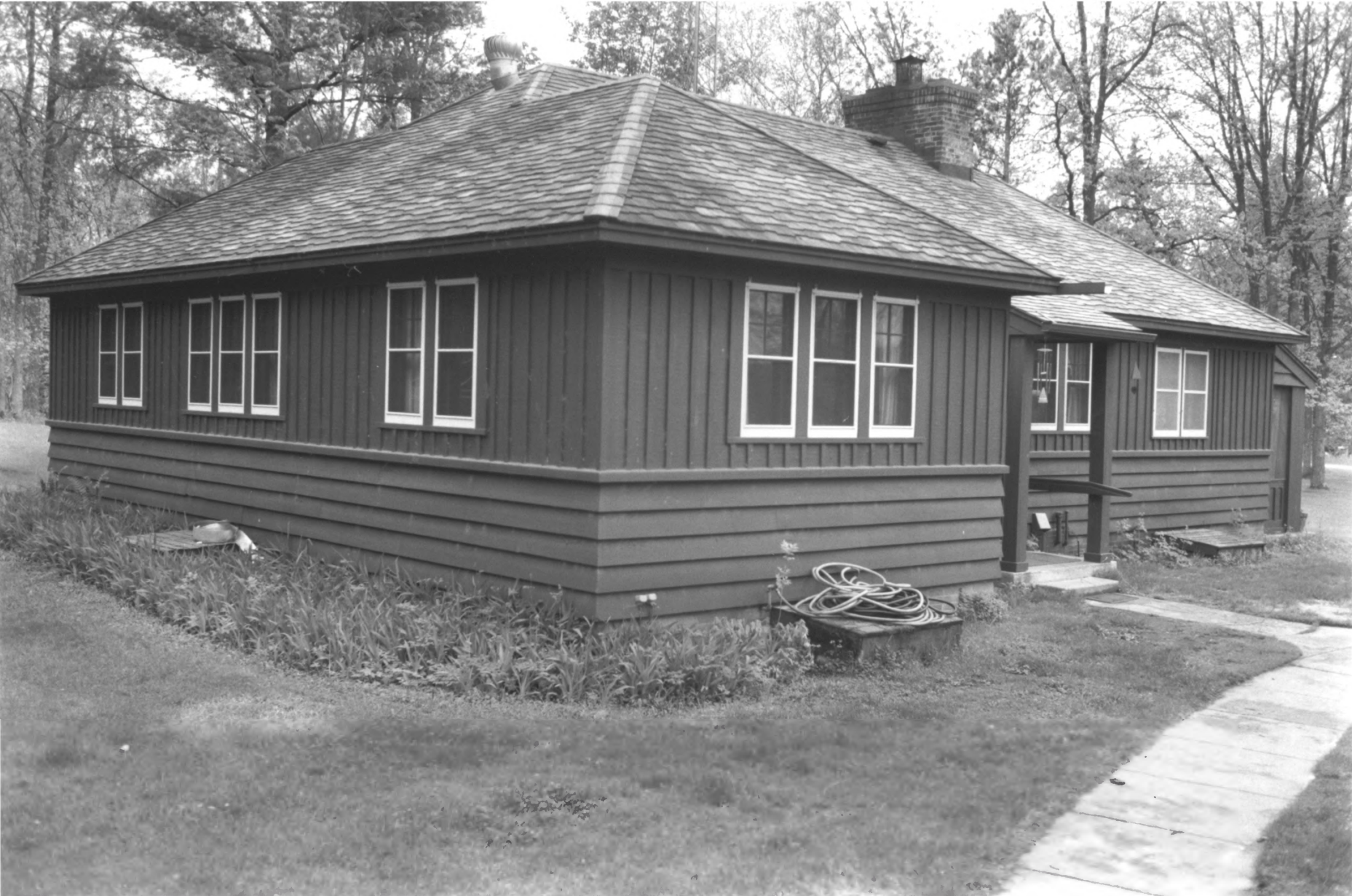
ITASCA STATE PARK CCC/WPA/RUSTIC STYLE HISTORIC RESOURCES CLEARWATER ; HUBBARD CDS MN BLDG # 51 PHOTO I.D. 09772 # 4
