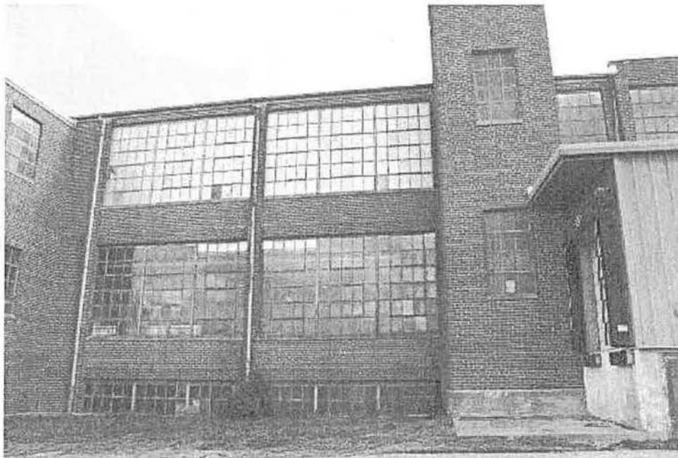
Figure 5: Elevator and window features.
