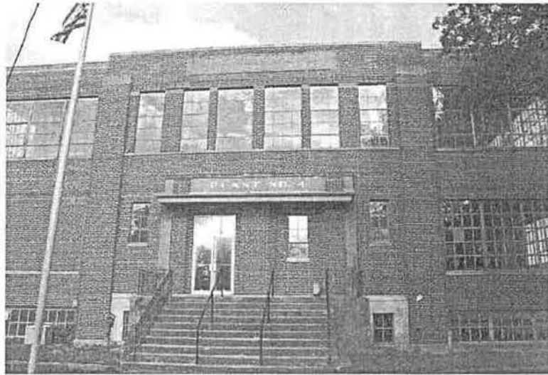
Figure 3: Front Facade facing east.
