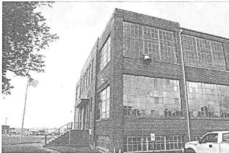
Figure 13: View showing basement, first and second floor windows.
