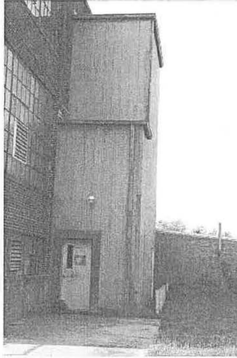
Figure 8: Rear stairwell enclosure.
