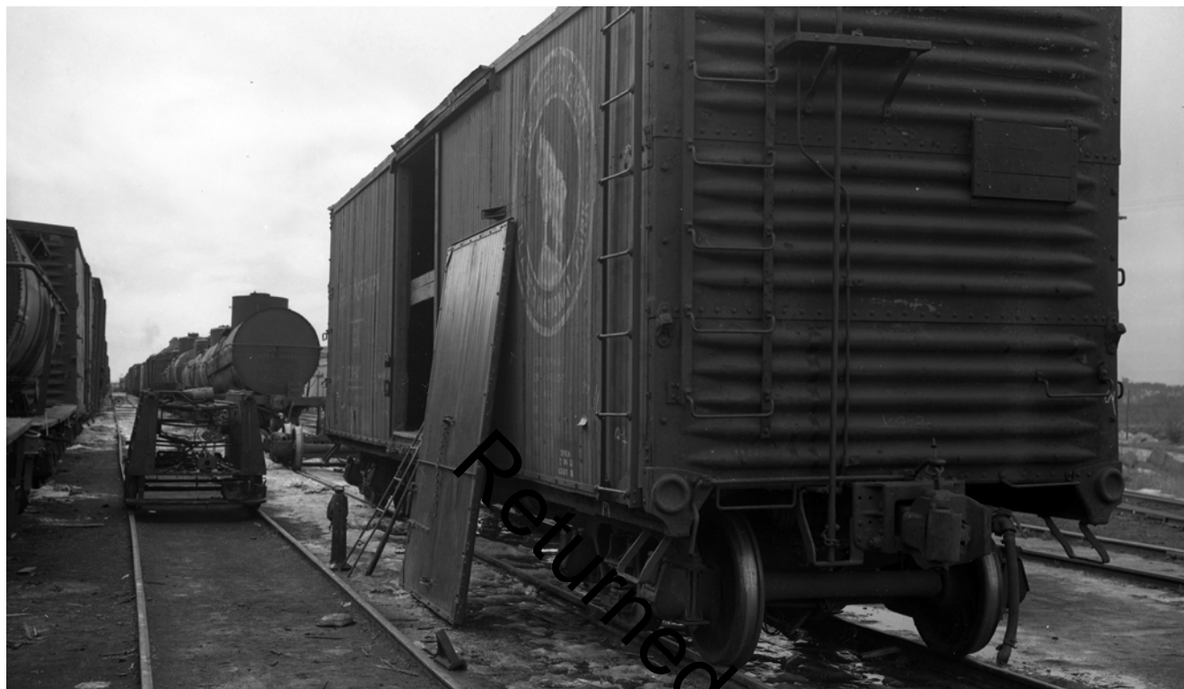
Historical Image: Box Car under repair on RIP (Repair-in-Place) Track
