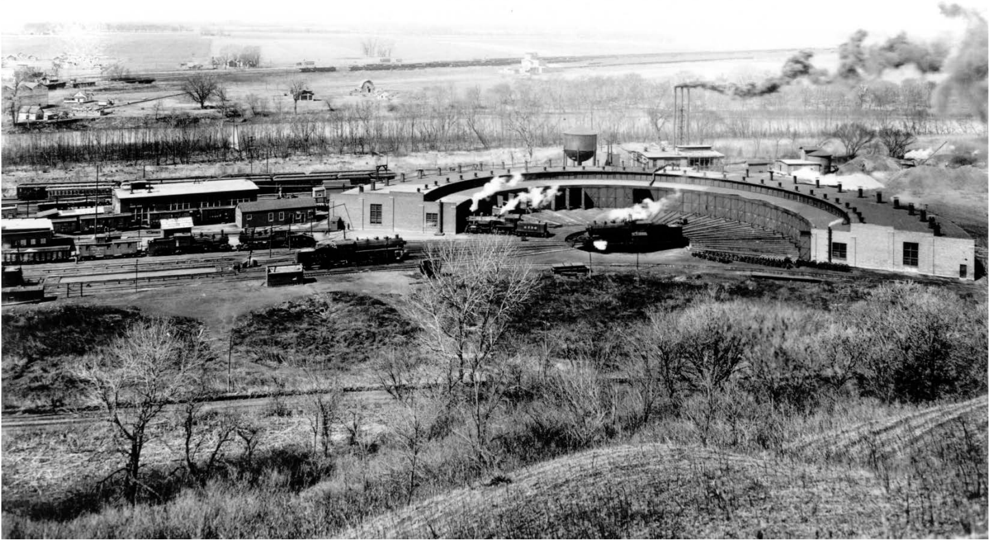
Figure 6: The Roundhouse building in 1920 anchoring the northern portion of the Sioux City Repair Shops. In the background are the various smaller repair shop buildings. View: Camera facing west (State of South Dakota in the background). Photographer: Woodworth Commercial Photos. Source: Sioux City Public Museum.
