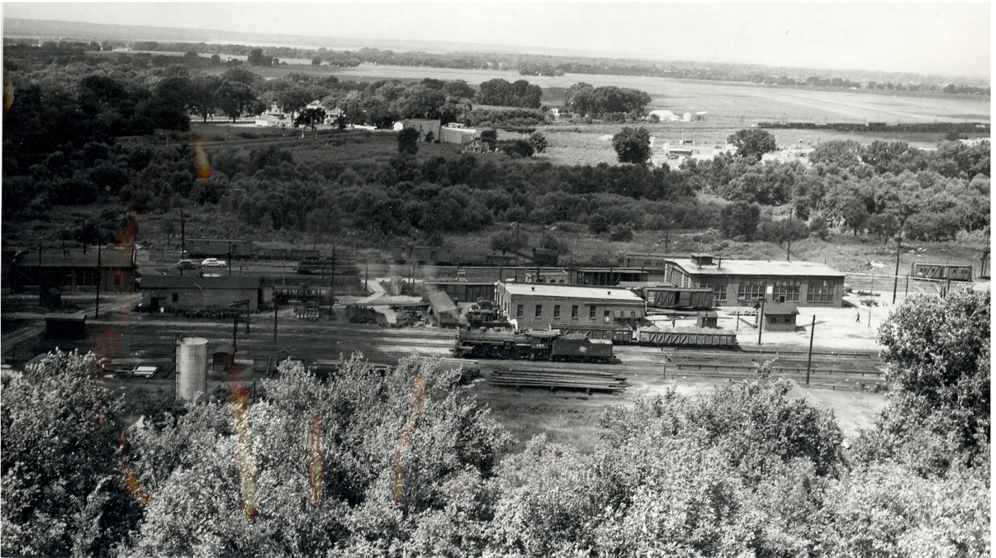
Figure 7: The center portion of the Sioux City Repair Shops in 1951. Buildings shown in this image (left to right) are the car department planing mill, oil house, store house and machine shop building. The new diesel fuel servicing terminal is in the foreground. Repair-in-Place (RIP) tracks and caboose storage area are in the background. View: Camera facing west. Photographer: George Berkstressor. Source: Archives of the Sioux City Railroad Museum.
