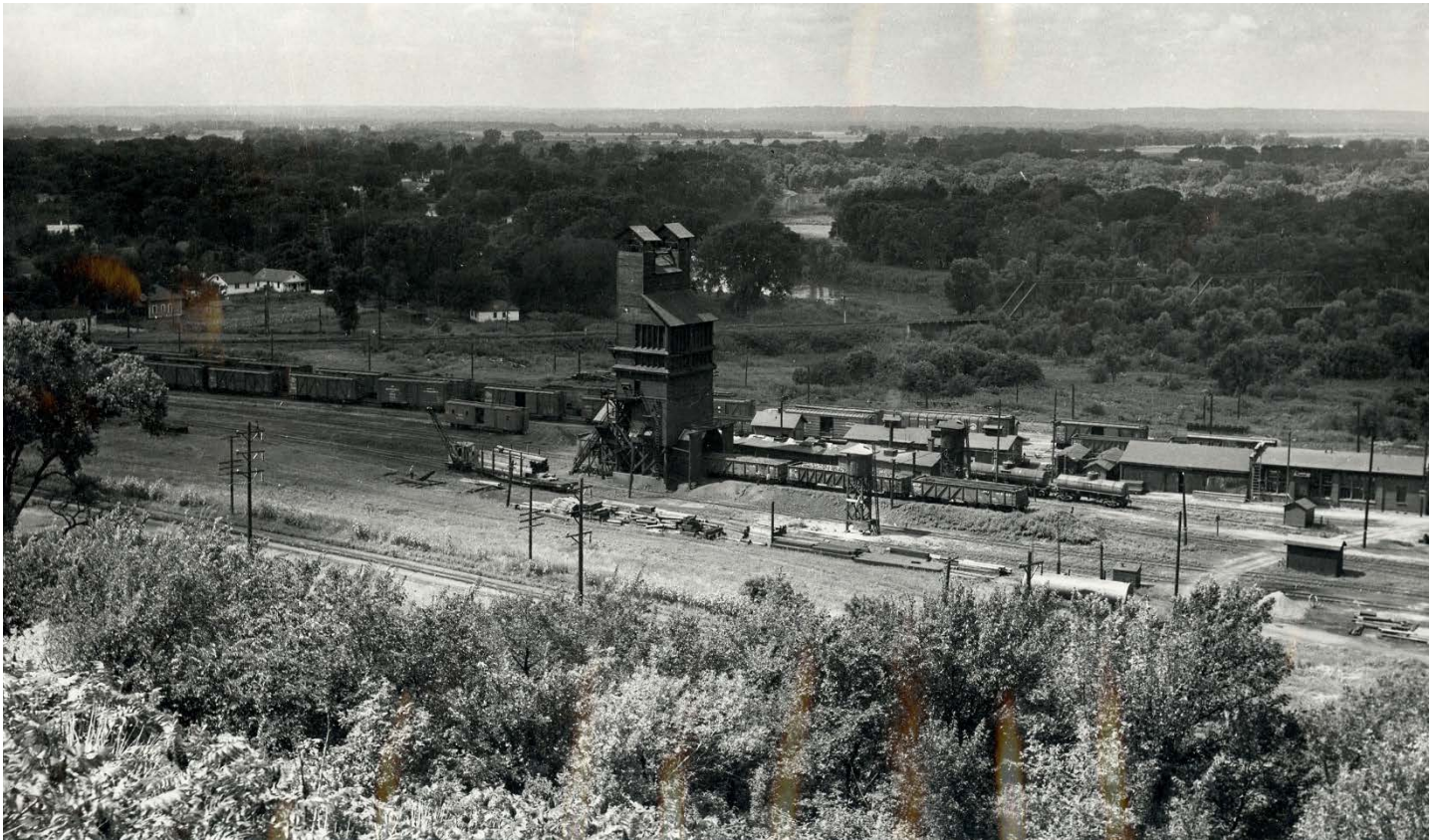
Figure 8: South portion of the Sioux City Repair Shops in 1951. This image shows the coal tower structure, sand drying towers, and various smaller shop buildings for the car repair department. Part of the work train and staging yard for the bridge and building department are in the foreground. View: Camera facing west. Photographer: George Berkstressor. Source: Archives of the Sioux City Railroad Museum.
