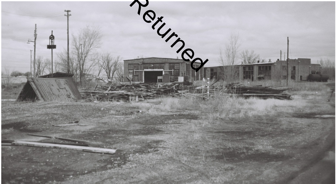
Historic Photo: Complex after abandonment in 1980. View: Looking northwest with the Machine/Blacksmith Shop Building and Roundhouse Photographer: Unknown, Morris Peterson Collection, Sioux City Railroad Museum
