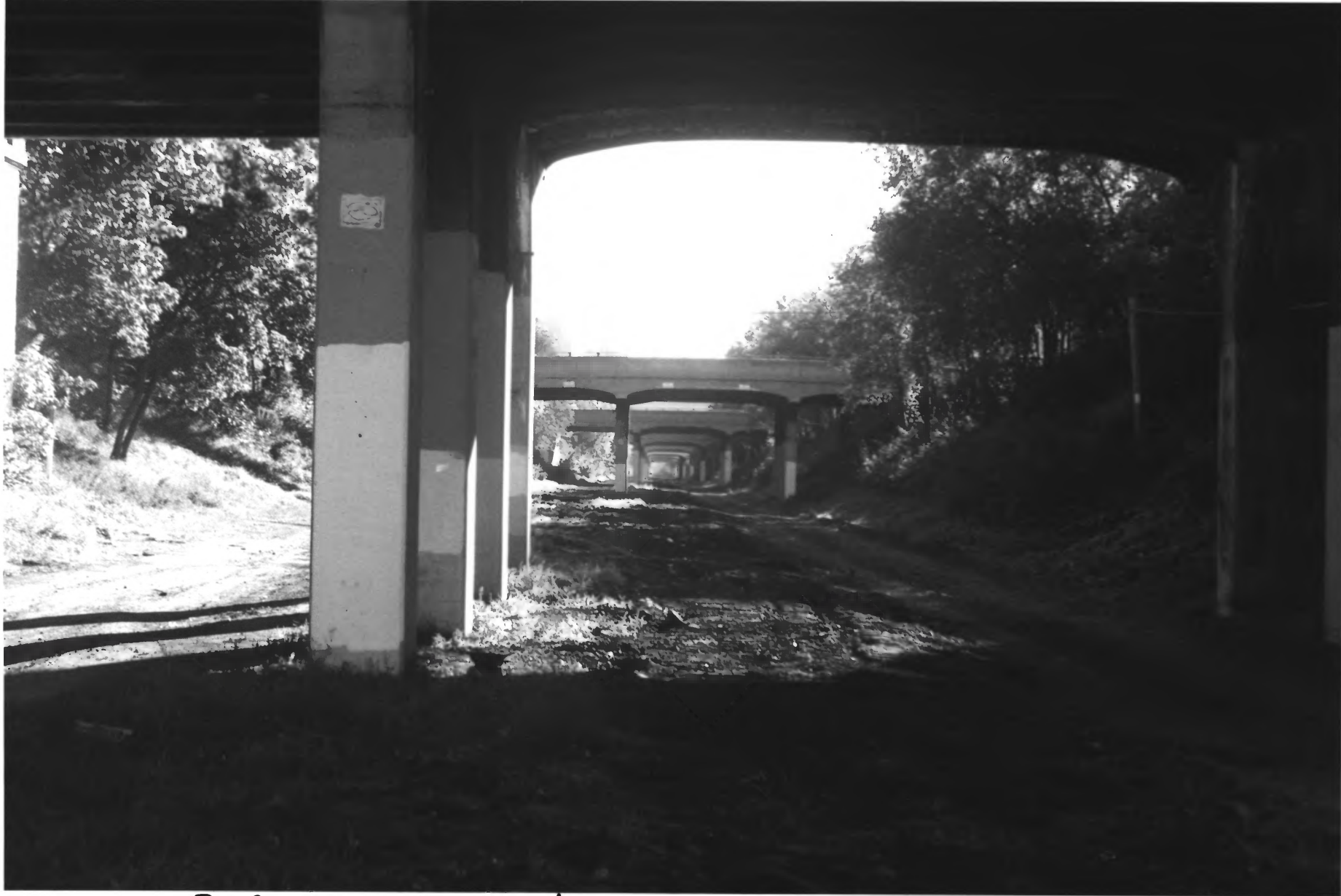
© M + ST P Grade Separation Hennepin Co., Mn 014509- 11/11A
