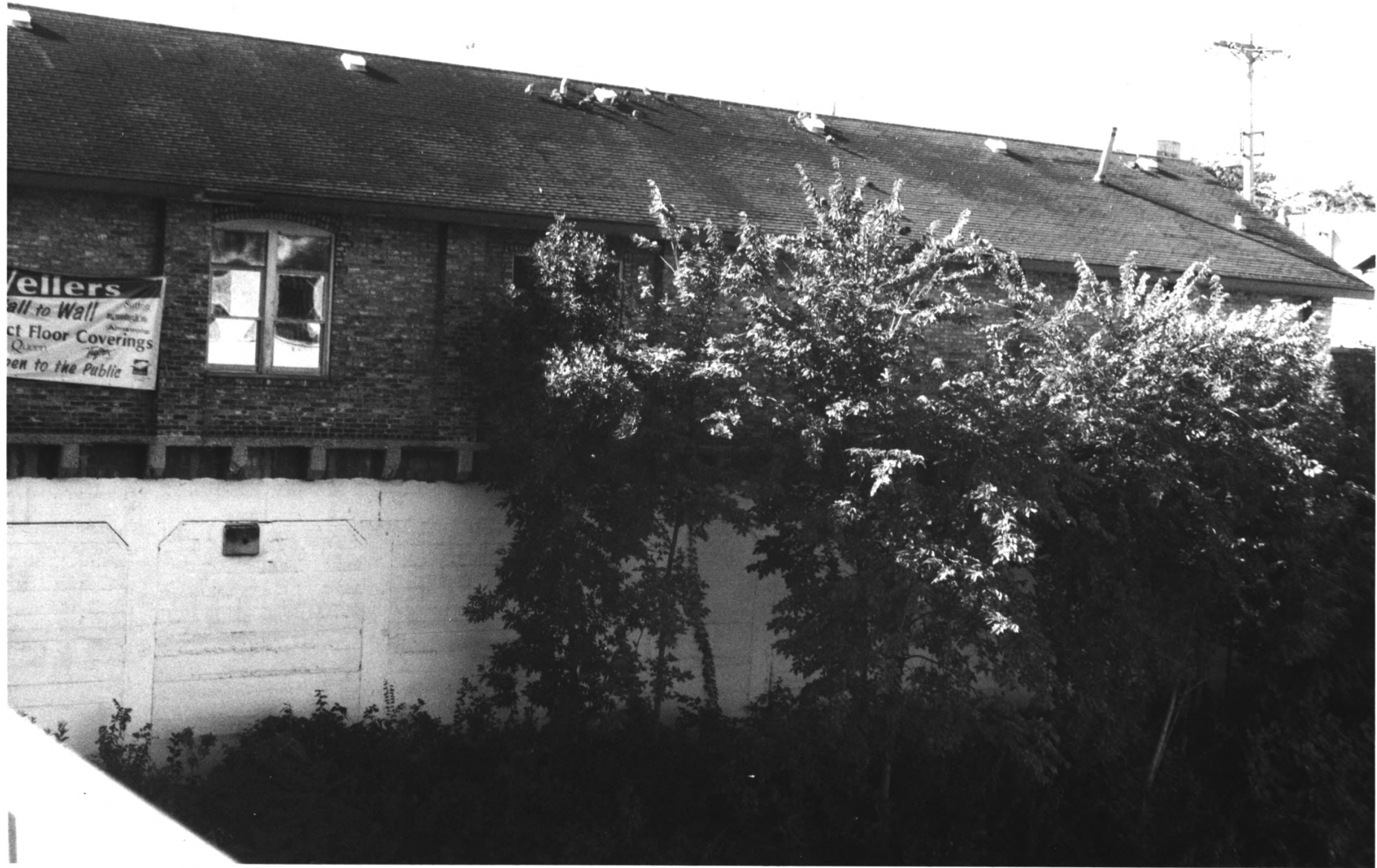
CM & St P Grade Separation Hennepin Co., Mn 014510 - 5A/6
