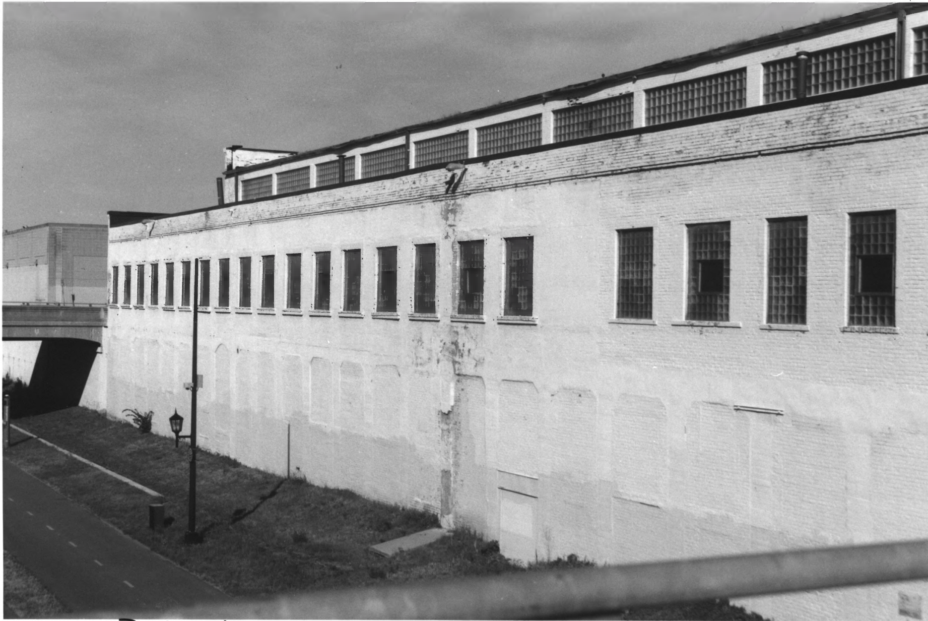
CM & ST P Grade Separation Hennepin Co., Mn 014510-1A
