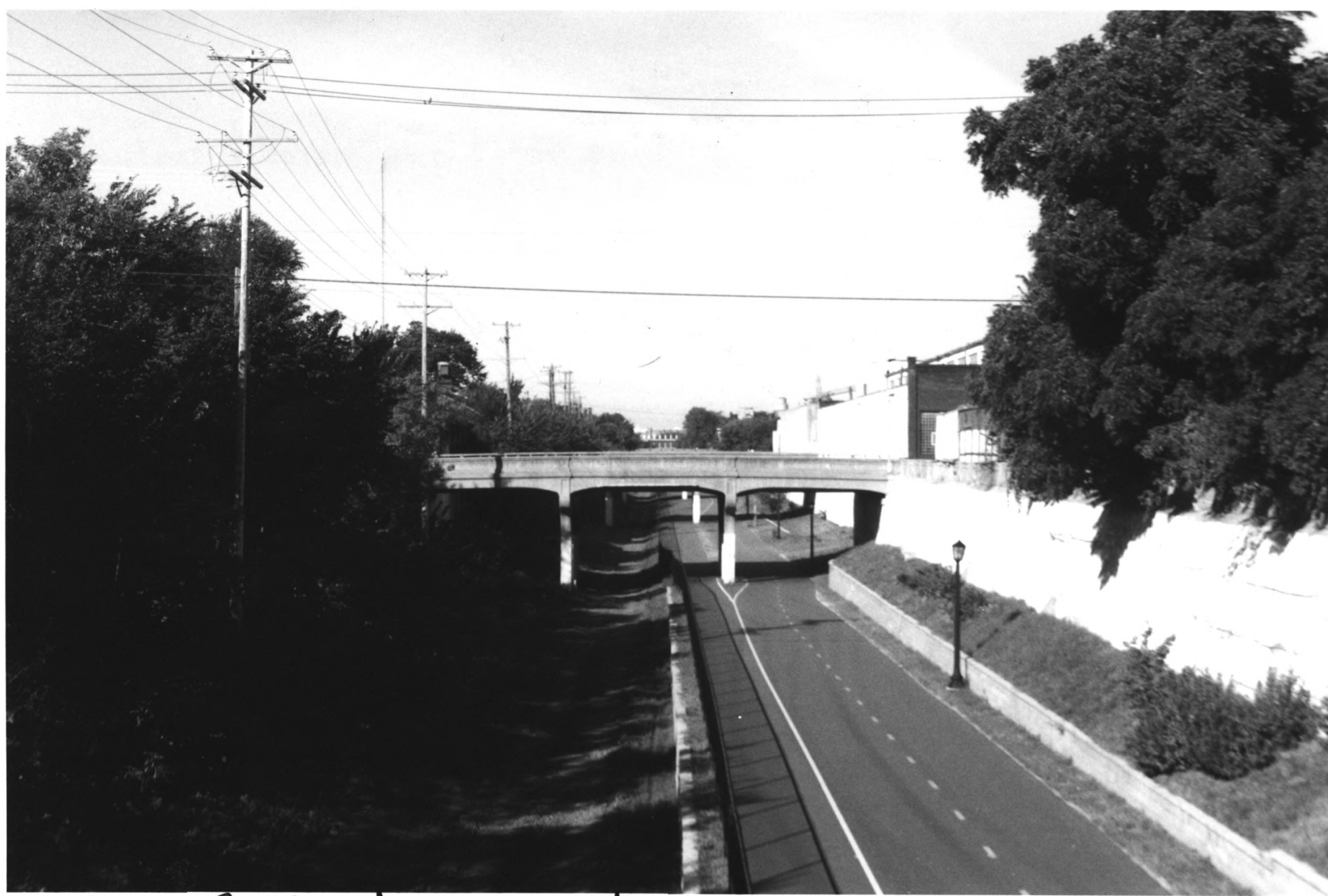
@ M + St P Grade Separation Hennepin Co., Mn 014510-0A
