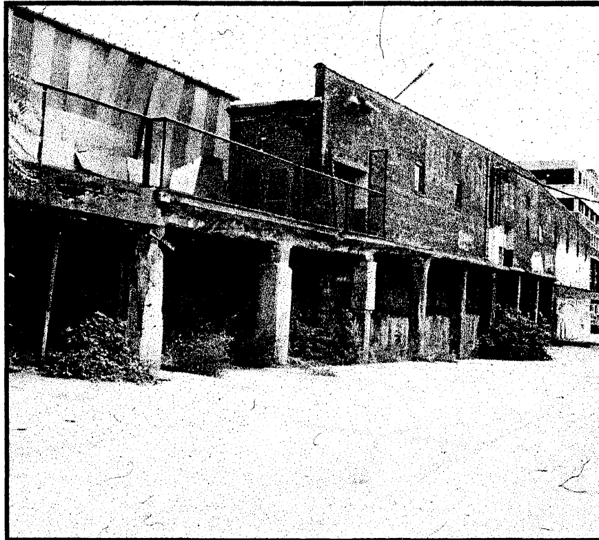
Figure 6, Loading dock and location of railroad spur.
