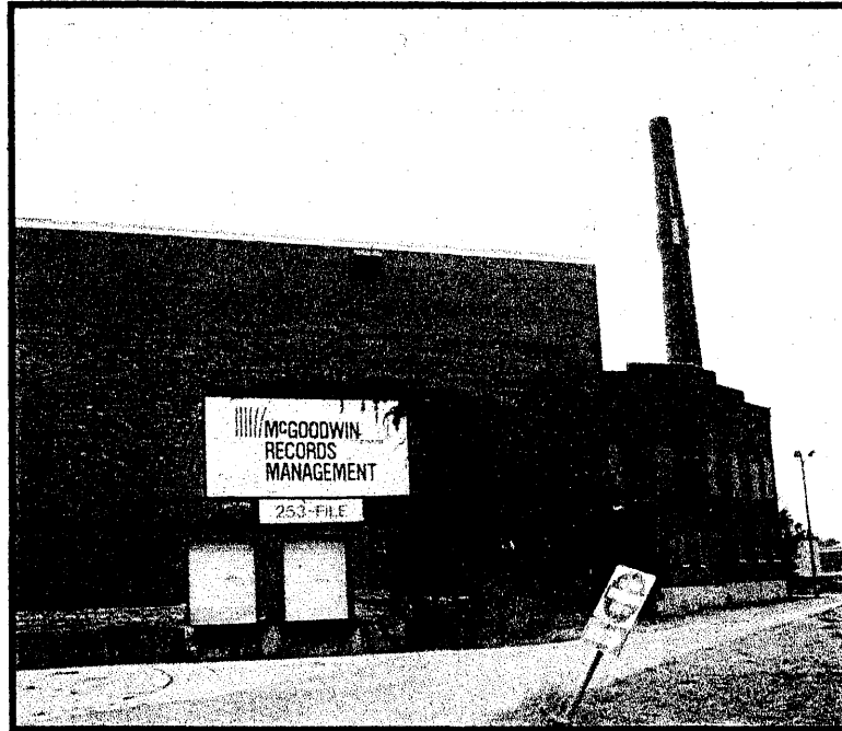
Figure 13, Truck loading dock alteration.
