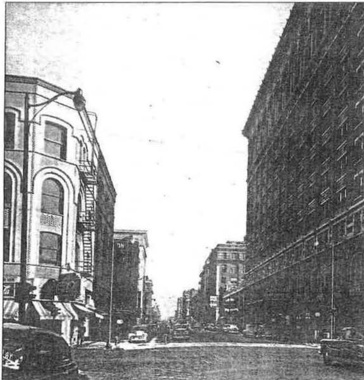
1949 photo of Germond Block, southwest façade corner (left side of photo)
