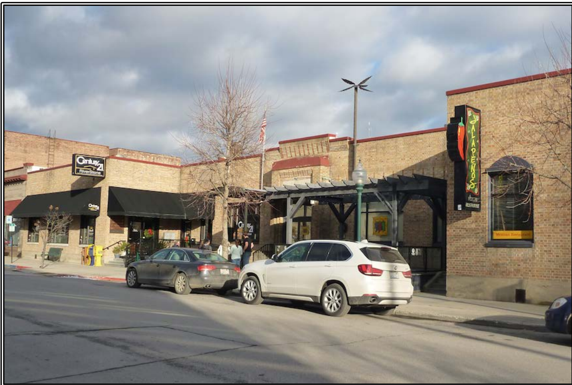
Figure 14: Current view of the Elks Lodge (Site 46)
