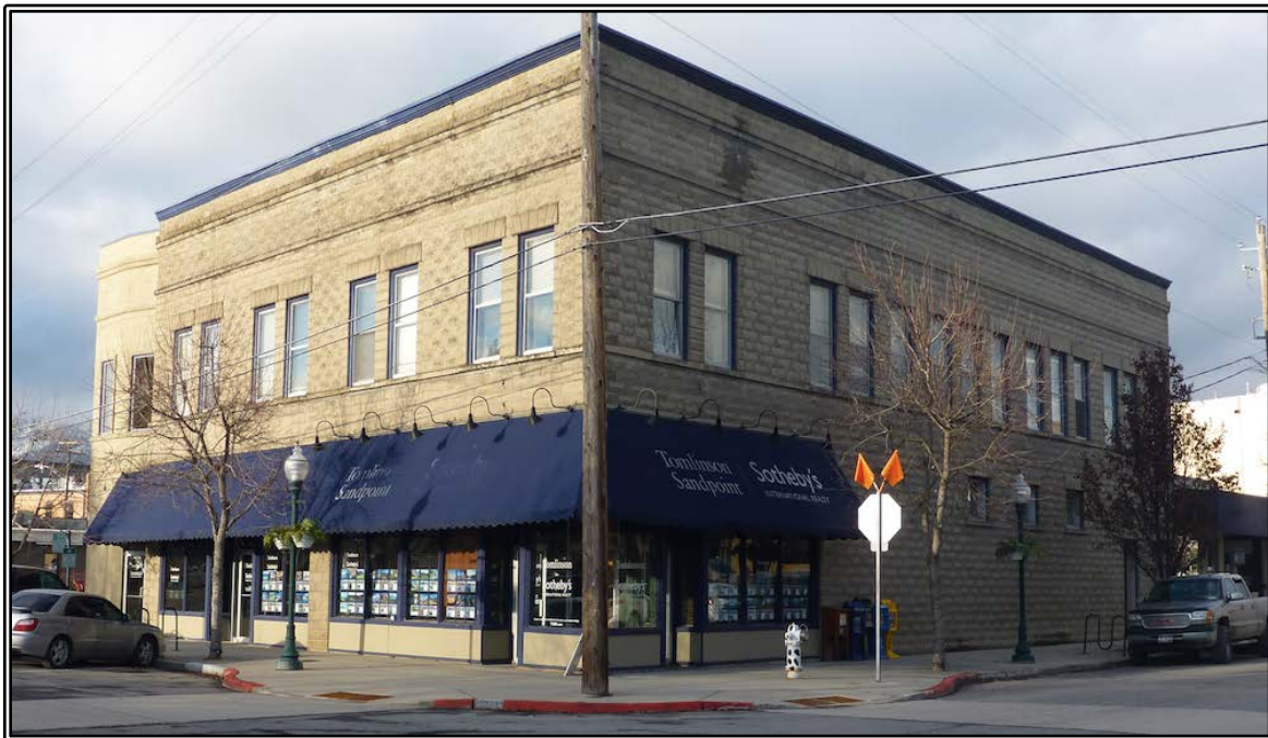
Figure 16: Current view of the building at Site 43
