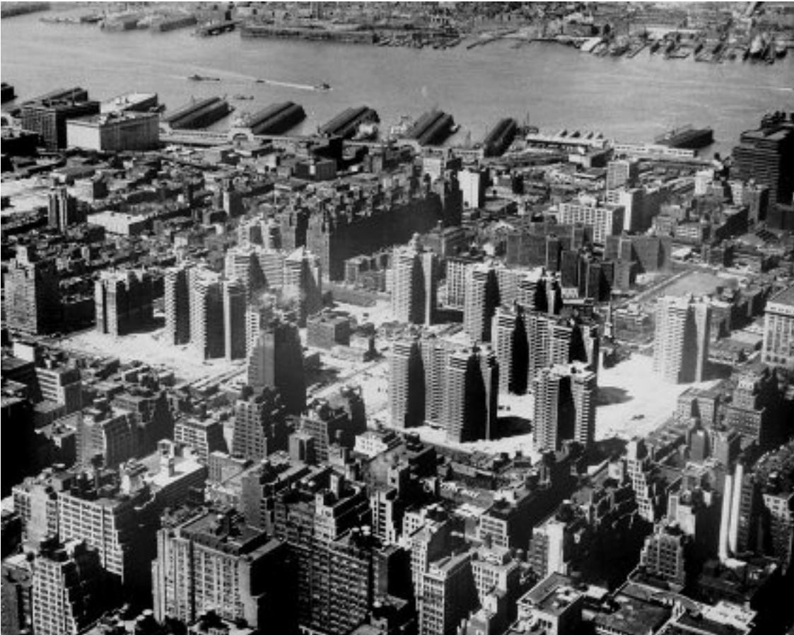
Penn South Construction Photo
