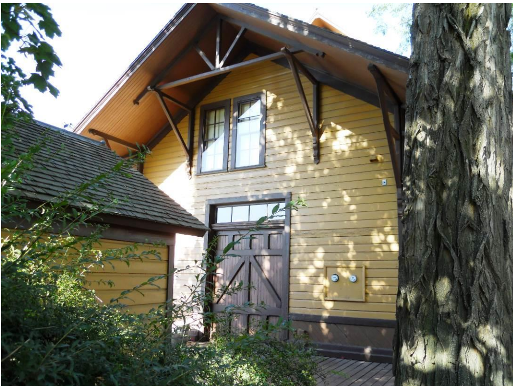
3 of 19. West façade of Depot, 2016.
