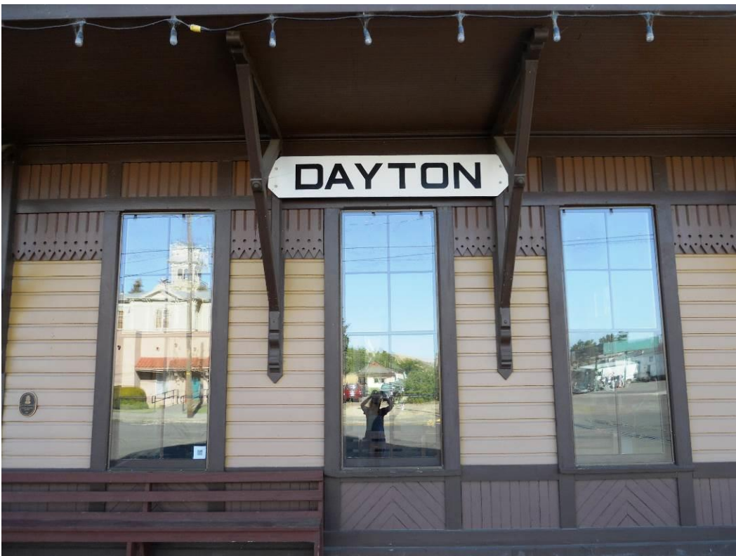
5 of 19. Close-up of east façade of Depot, 2016.
