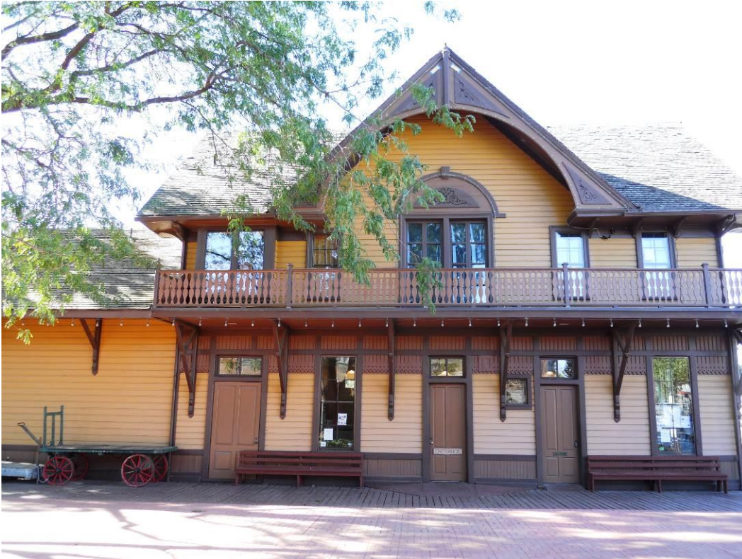
4 of 19. South façade of Depot, 2016.
