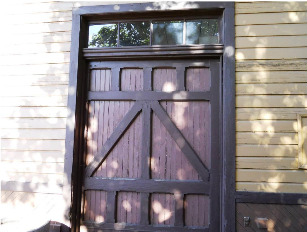
7 of 19. Freight door on west end of Depot, 2016.
