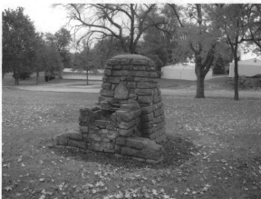
Typical small stone fireplace (12) on west hill to southeast Note golf cart storage buildings in background (Naumann photo October 2006)
