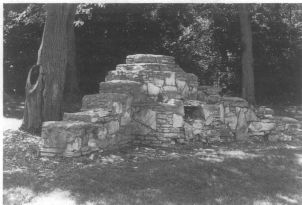
Large stone fireplace (10) on west hill to west (Patterson photo July 2006)
