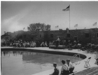
Swimming Pool (20) dedication July 4, 1937 to southwest (Photo from State Historical Society of Iowa, Special Collections, Iowa City, IA)
