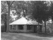
North shelter house (23) to northeast (Naumann photo August 2004)
