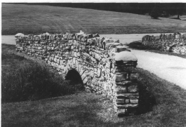
West bridge (7) to northeast (Patterson photo July 2006)
