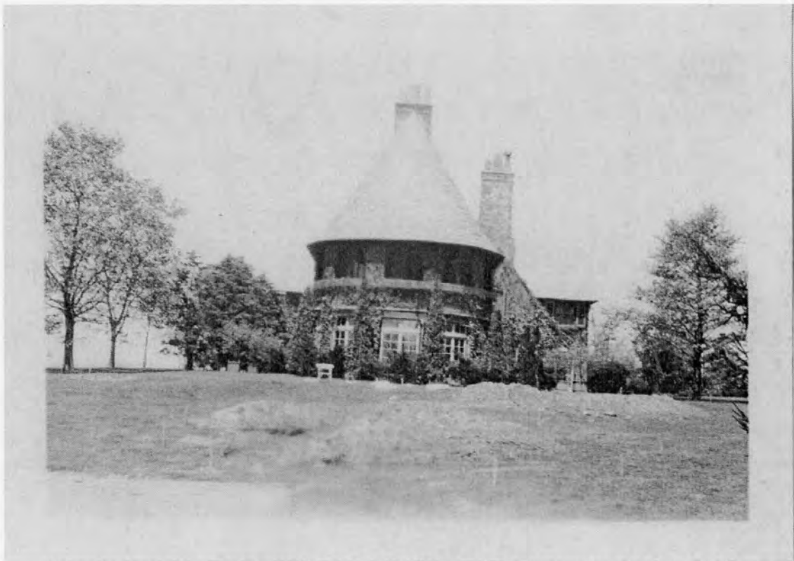
Historic photo circa 1928. East side of House as Boxwood Garden construction is beginning.
