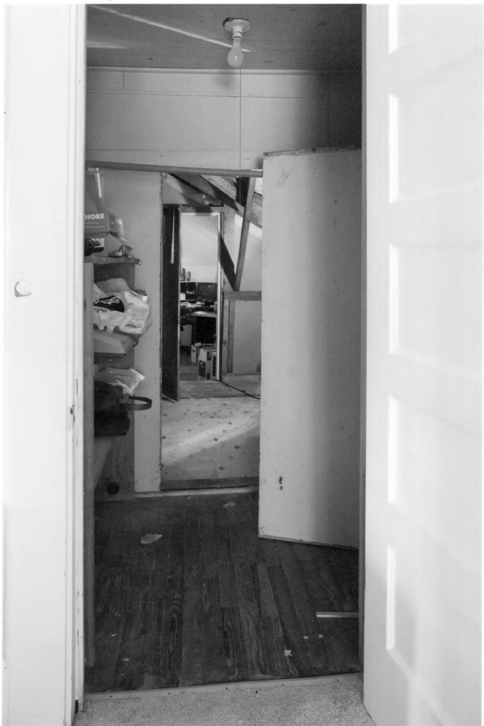
Boyd and Sallie Gilleland House Dawson County, Georgia Photograph 23 of 32
