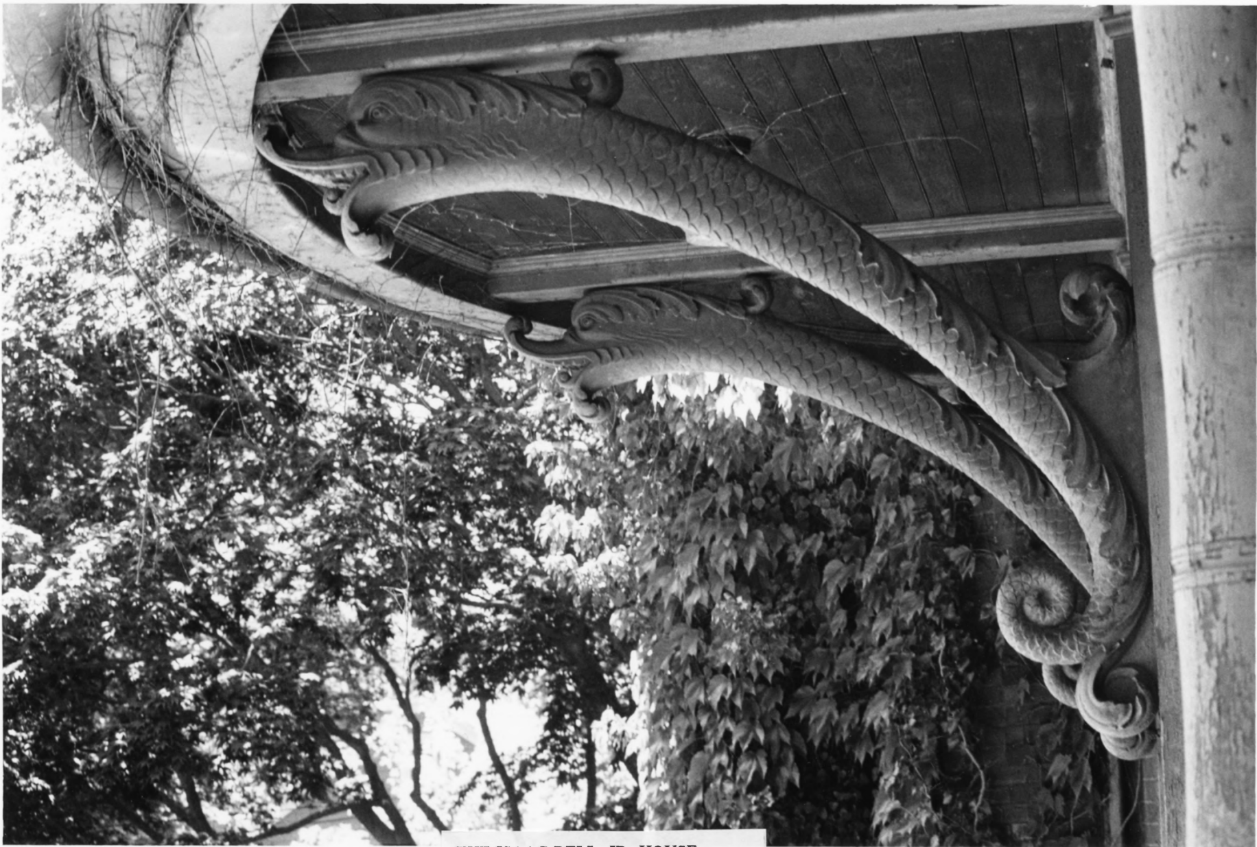
THE ISAAC BELL, JR. HOUSE Newport, Rhode Island Dolphins brackets Photo: Mesick, Cohen, Wilson, Baker, AIA, 1995
