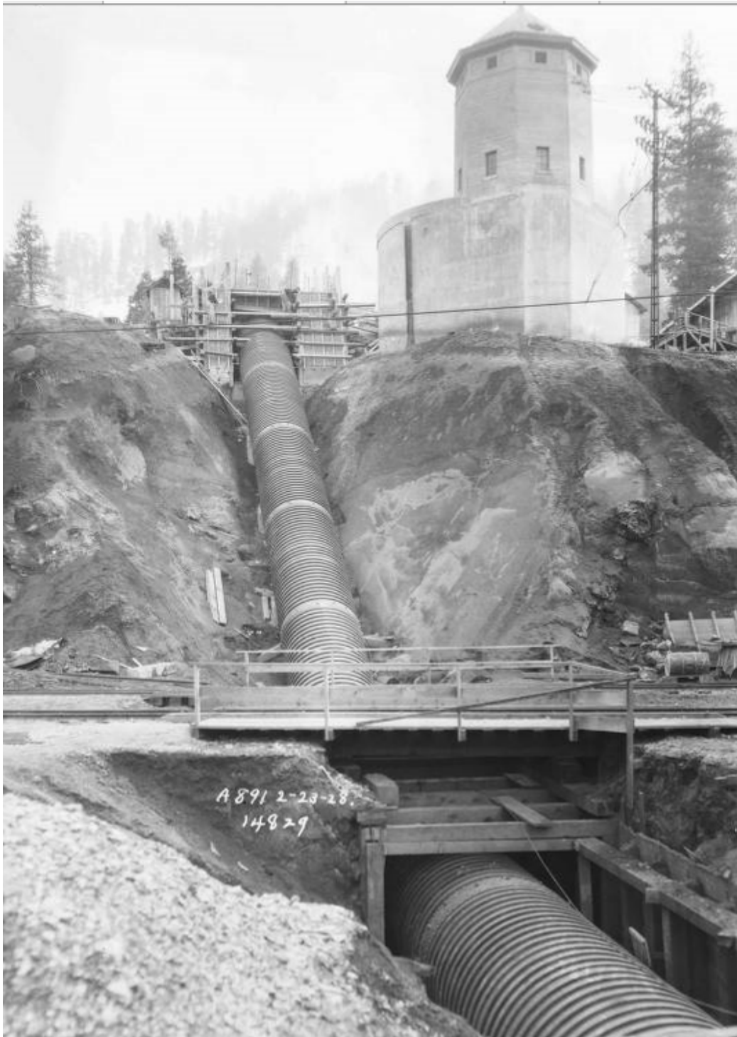
Figure 86: Powerhouse No. 2A Penstock, 1928. Image No. SCE-02-14829, Huntington Digital Library.
