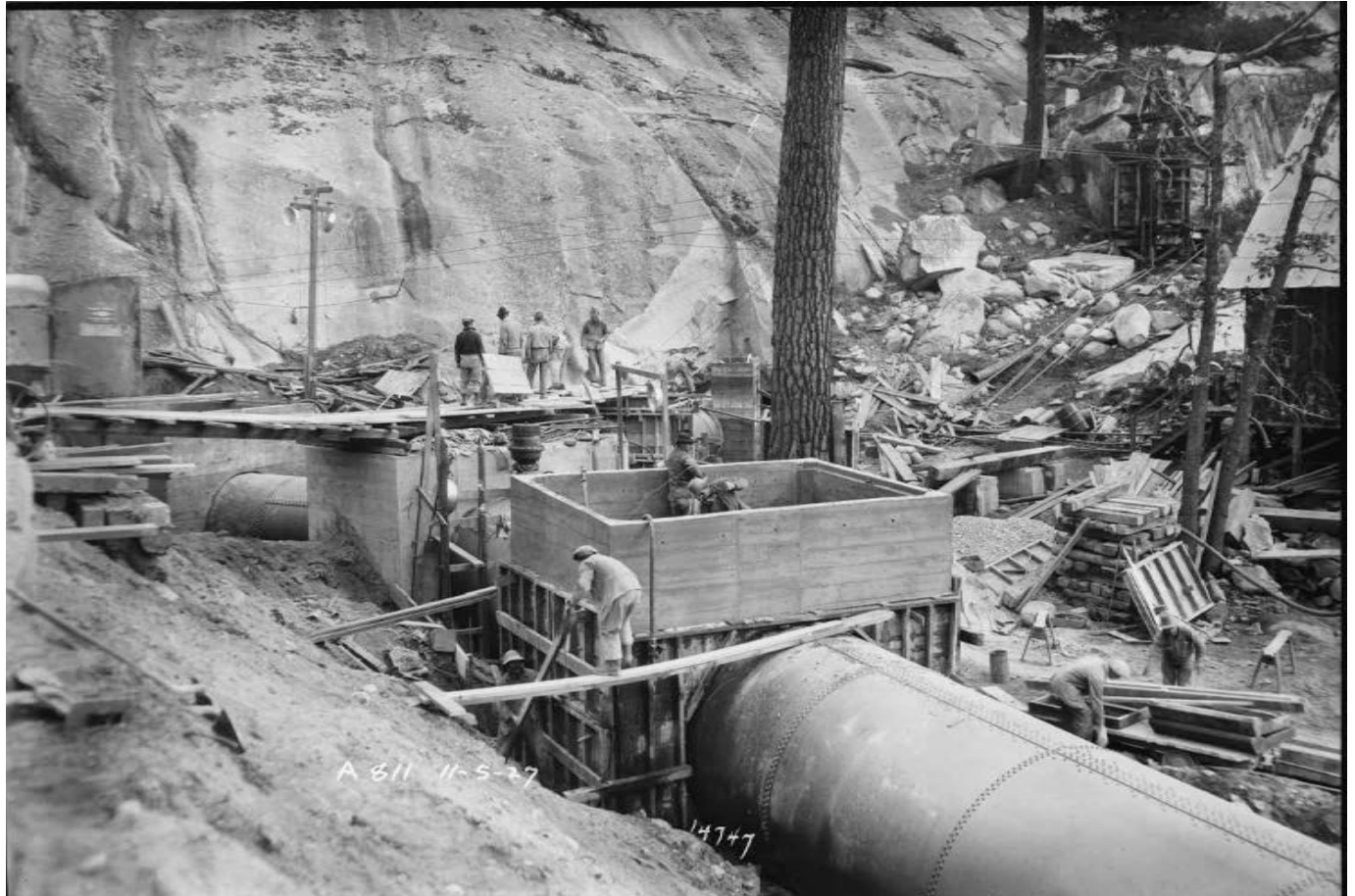
Figure 77: Intersection of Mono and Bear Tunnels with Mono Bear Siphon, 1927. Image No. SCE-02-14747, Huntington Digital Library.
