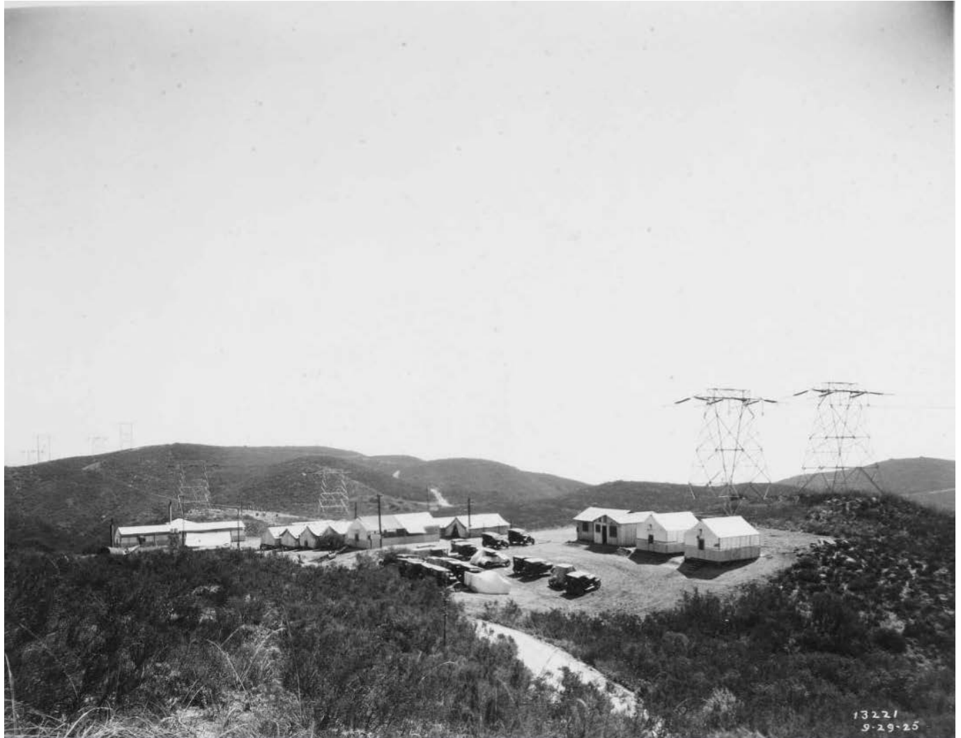
Figure 92: Vincent Transmission Line at site of Gould Substation, 1925. Image No. SCE-02-13221, Huntington Digital Library.
