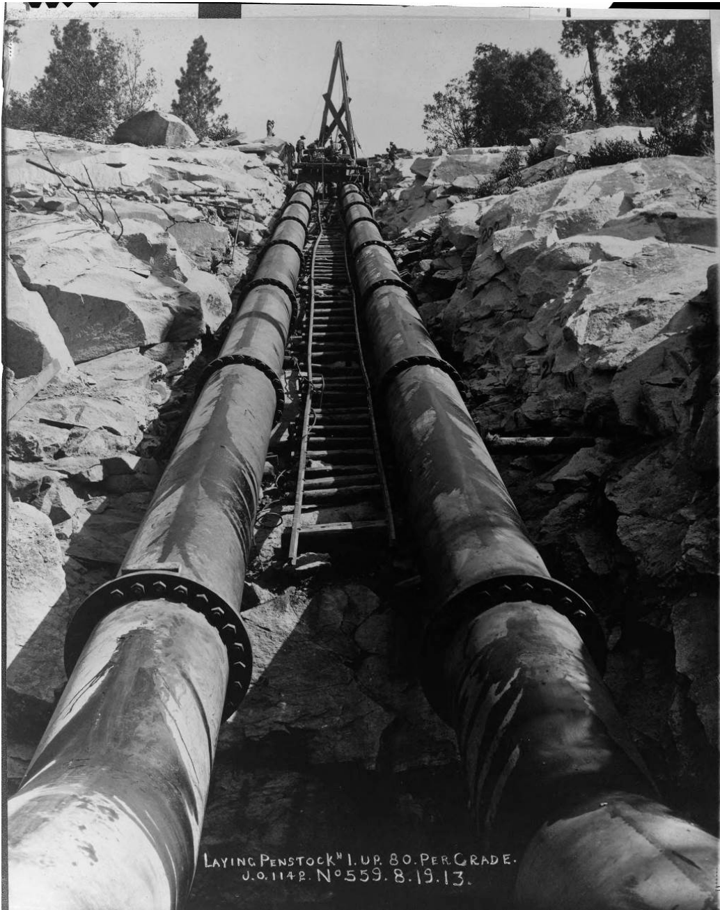
Figure 15: Powerhouse No. 1 Penstocks under construction, 1913. Image No. SCE-12-00042, Huntington Digital Library.
