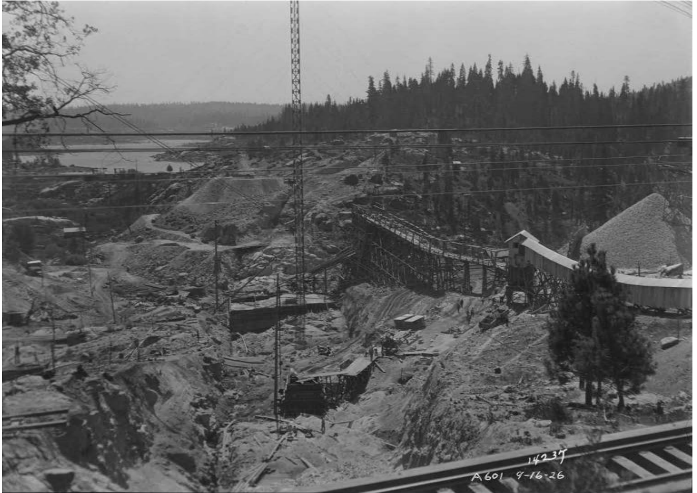
Figure 79: Shaver Lake Dam Construction, 1926. Image No. SCE-02-14237, Huntington Digital Library.
