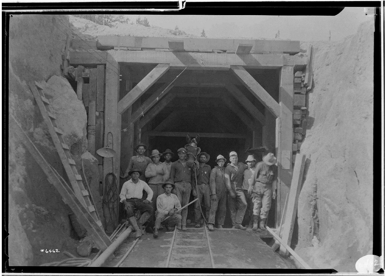
Figure 27: Group of 11 miners and tunnel mule at entrance to Tunnel No. 5 Flowline, 1920. Image No. SCE-02-06462, Huntington Digital Library.
