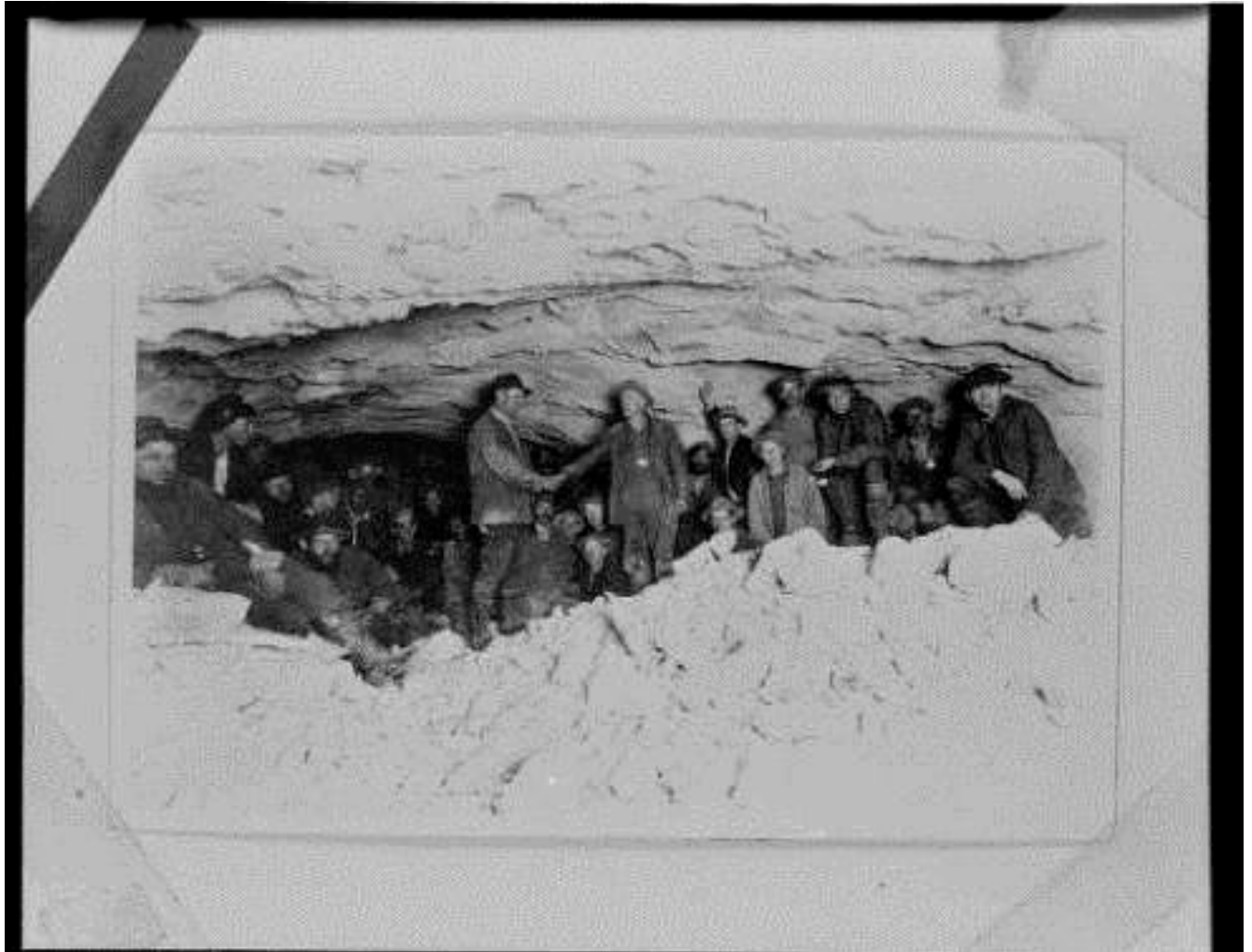
Figure 58: Two crews “tunneling through” Florence/Ward Tunnel, 1925. Image No. SCE-05-51096, Huntington Digital Library.
