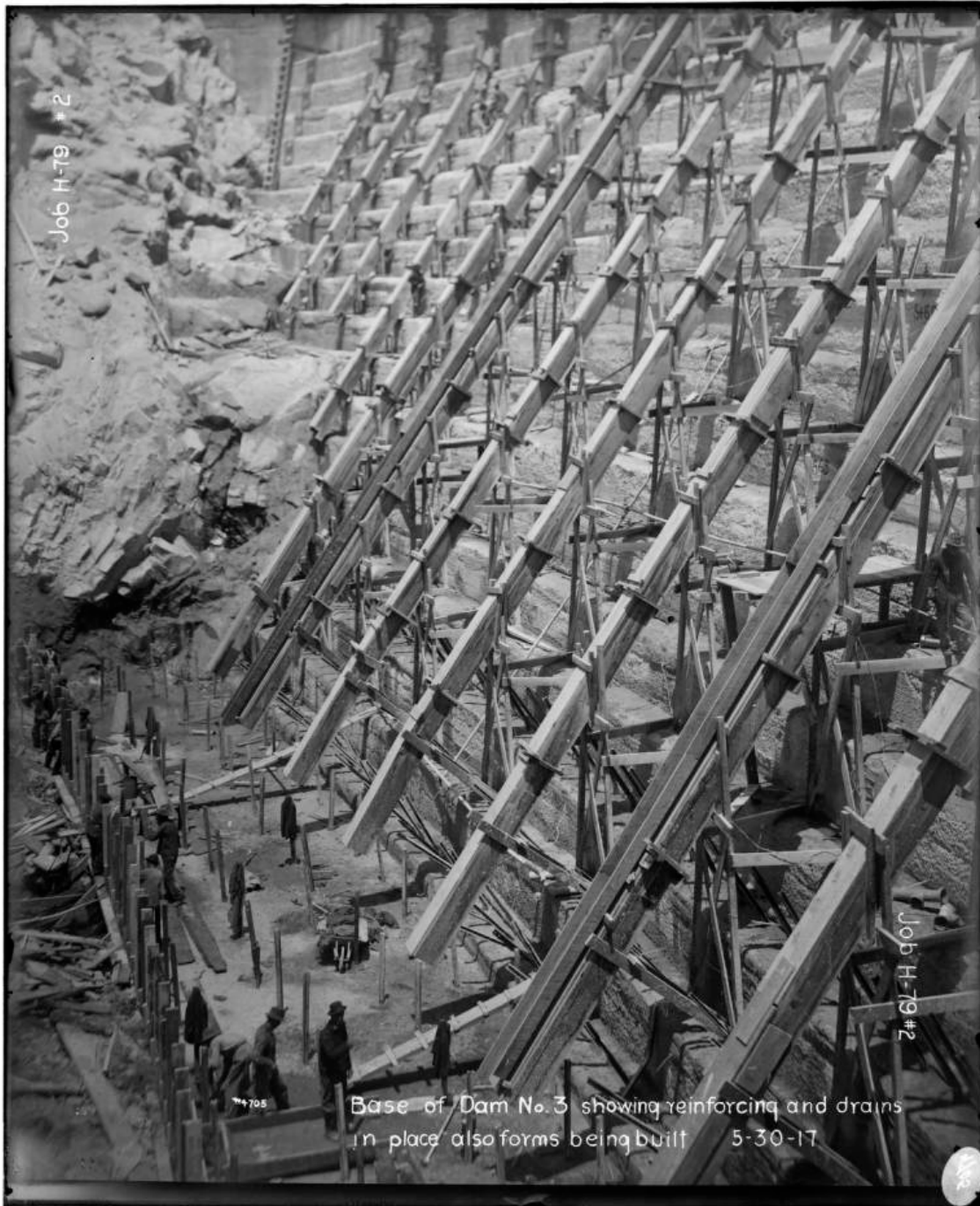
Figure 6: Huntington Lake Dam No. 3, 1917. Image depicts forms, reinforcing, and drains for raising of dam. Image No. SCE-02-04705, Huntington Digital Library.
