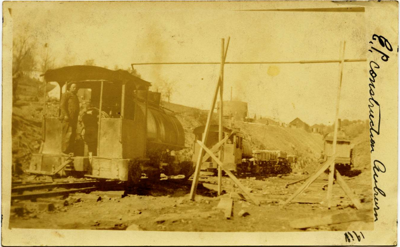
Figure 109: SJ&E grade under construction near Auberry, 1912. Courtesy of the Michael J. Semas Collection, Auberry.
