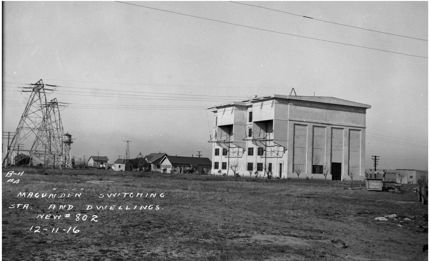
Figure 99: Magunden Substation, with Big Creek East and West Transmission Lines and attendant housing, 1916. Image No. SCE-03-00802, Huntington Digital Library.
