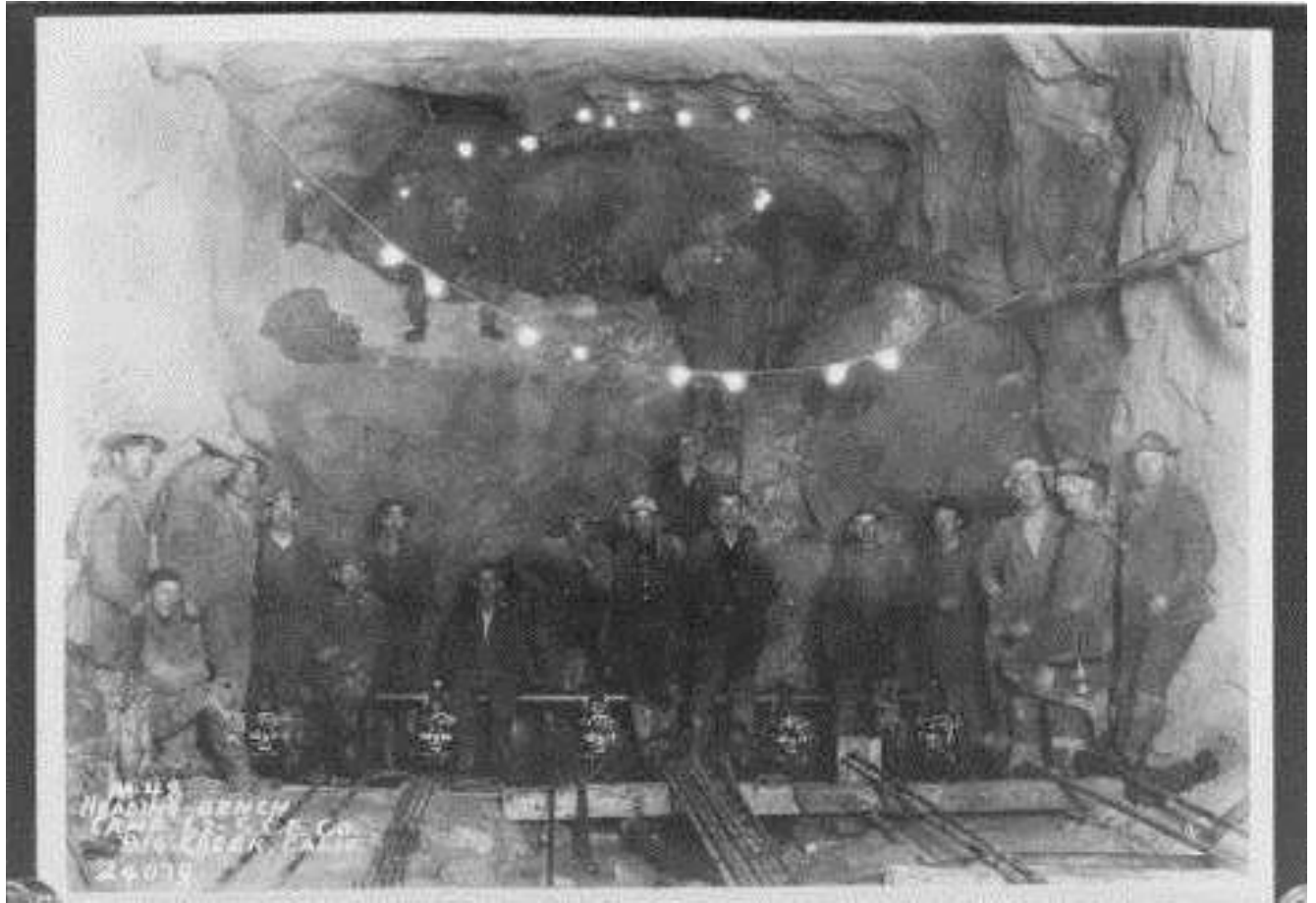
Figure 57: Florence/Ward Tunnel Digging, circa 1924. Image No. SCE-02-24079, Huntington Digital Library
