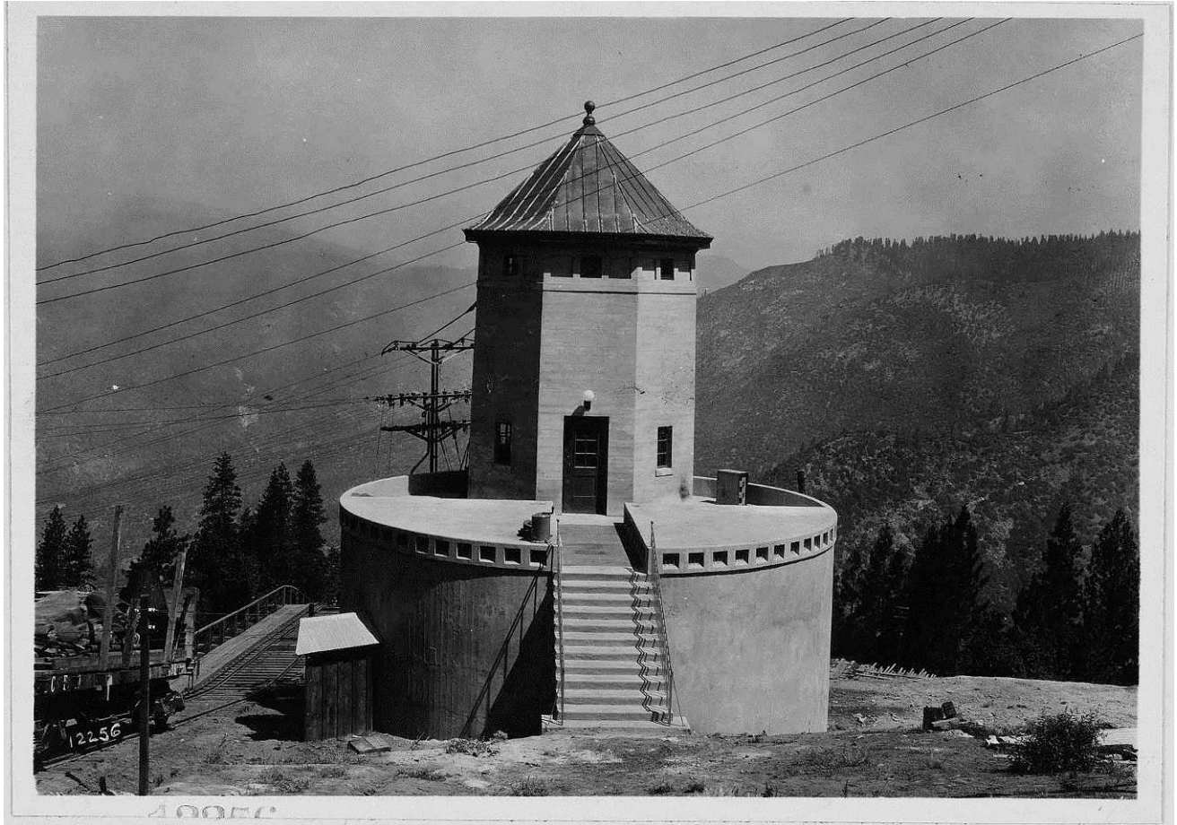
Figure 20: Tunnel No.2 Flowline Gate House (surge chamber) located at West Portal (termination of Tunnel No. 2), 1924.
