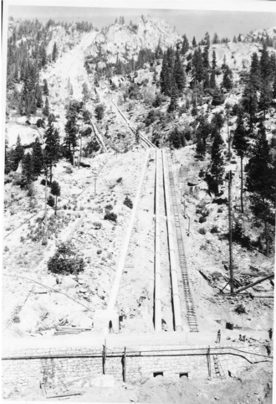
Figure 120: Incline No. 1 from Powerhouse No. 1 roof, 1913. Call No. Stone & Webster, 13-Vol. 028, PO35, Huntington Digital Library.
