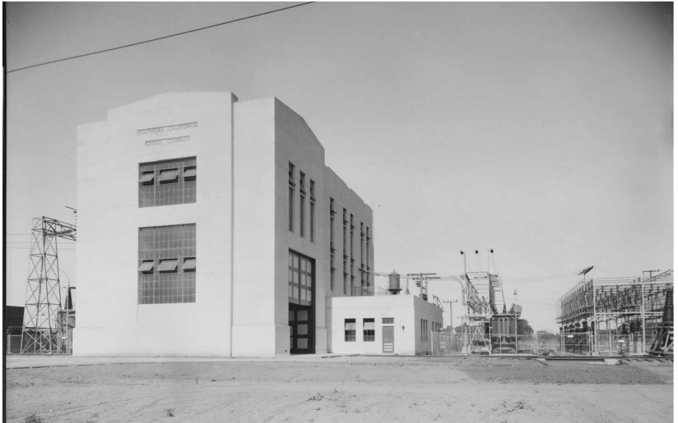
Figure 104: Rector Substation, 1928. Image No. SCE-02-15380, Huntington Digital Library.
