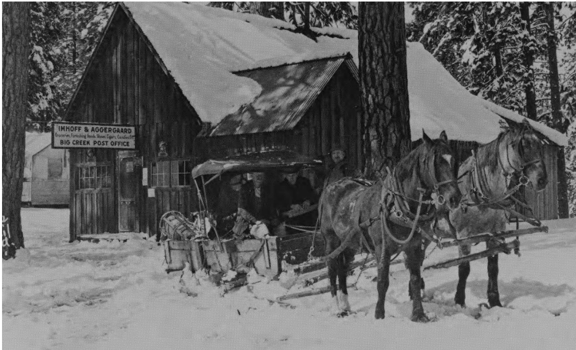
Figure 152: Big Creek Post Office, circa 1912. Image No. SCE-12-00200, Huntington Digital Library.
