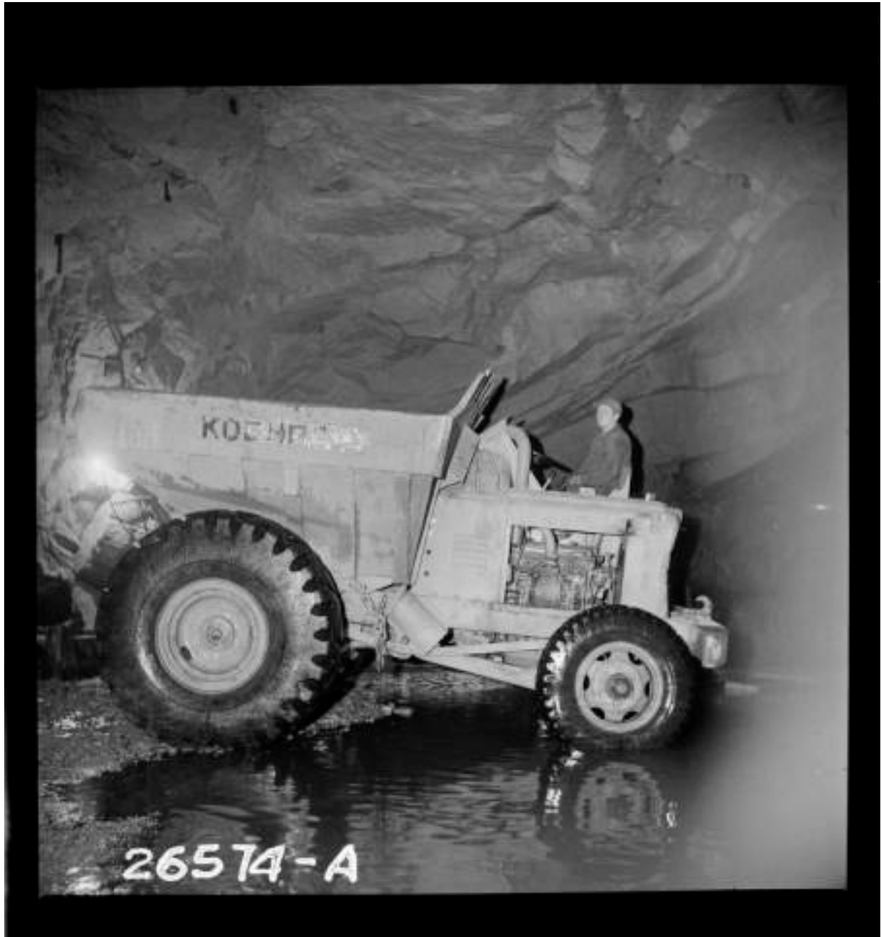
Figure 60: Repairs to Ward Tunnel, GM Dumpster Truck 1945. Image No. SCE-02-26574A, Huntington Digital Library.
