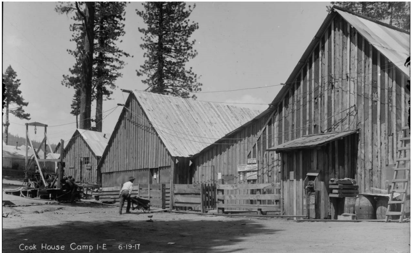
Figure 137: Camp 1-E Cookhouse, 1917. Photo No. SCE-02-04722, Huntington Digital Library.
