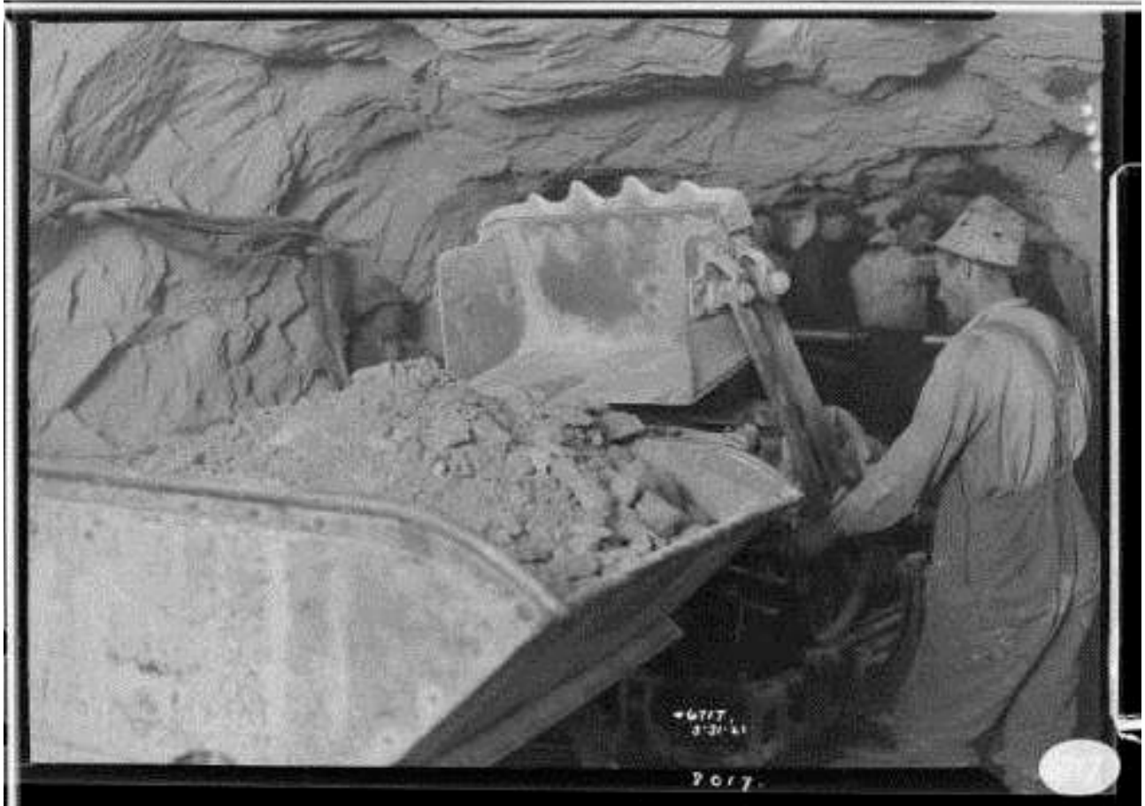
Figure 28: Men working at the heading of Tunnel No. 5 with Armstrong Mucker “shuveloader,” 1921. Image No. SCE-02-06717, Huntington Digital Library.
