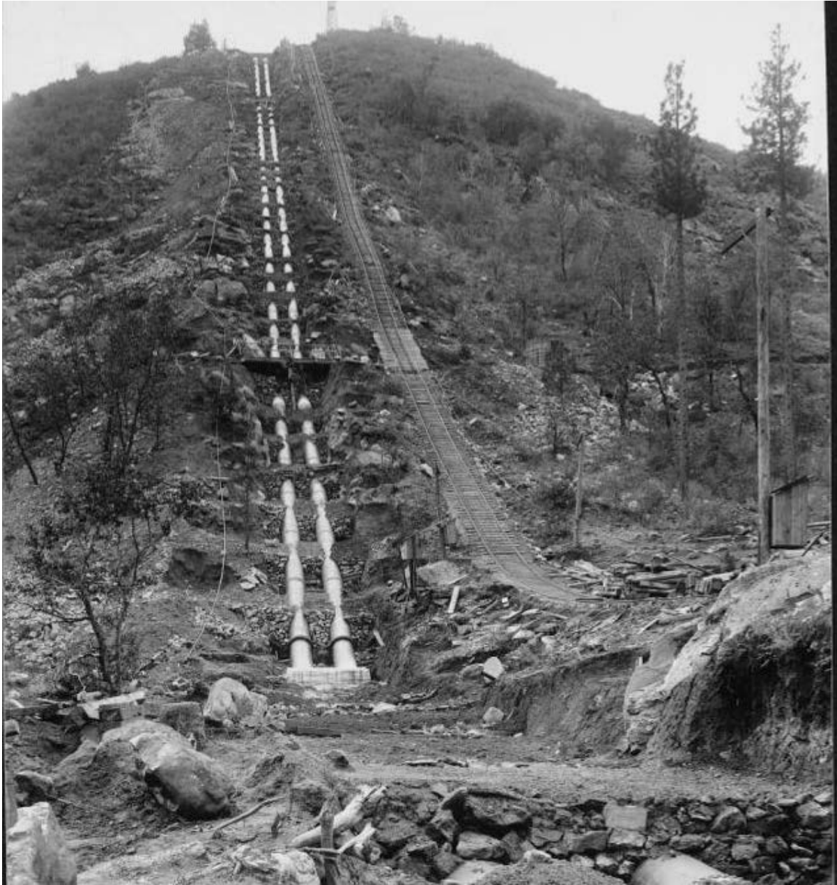
Figure 121: Incline No. 2, with Powerhouse No. 2 Penstocks at left, 1912-1913. Call No. Stone & Webster, 13-Vol. 15, PO66, Huntington Digital Library.
