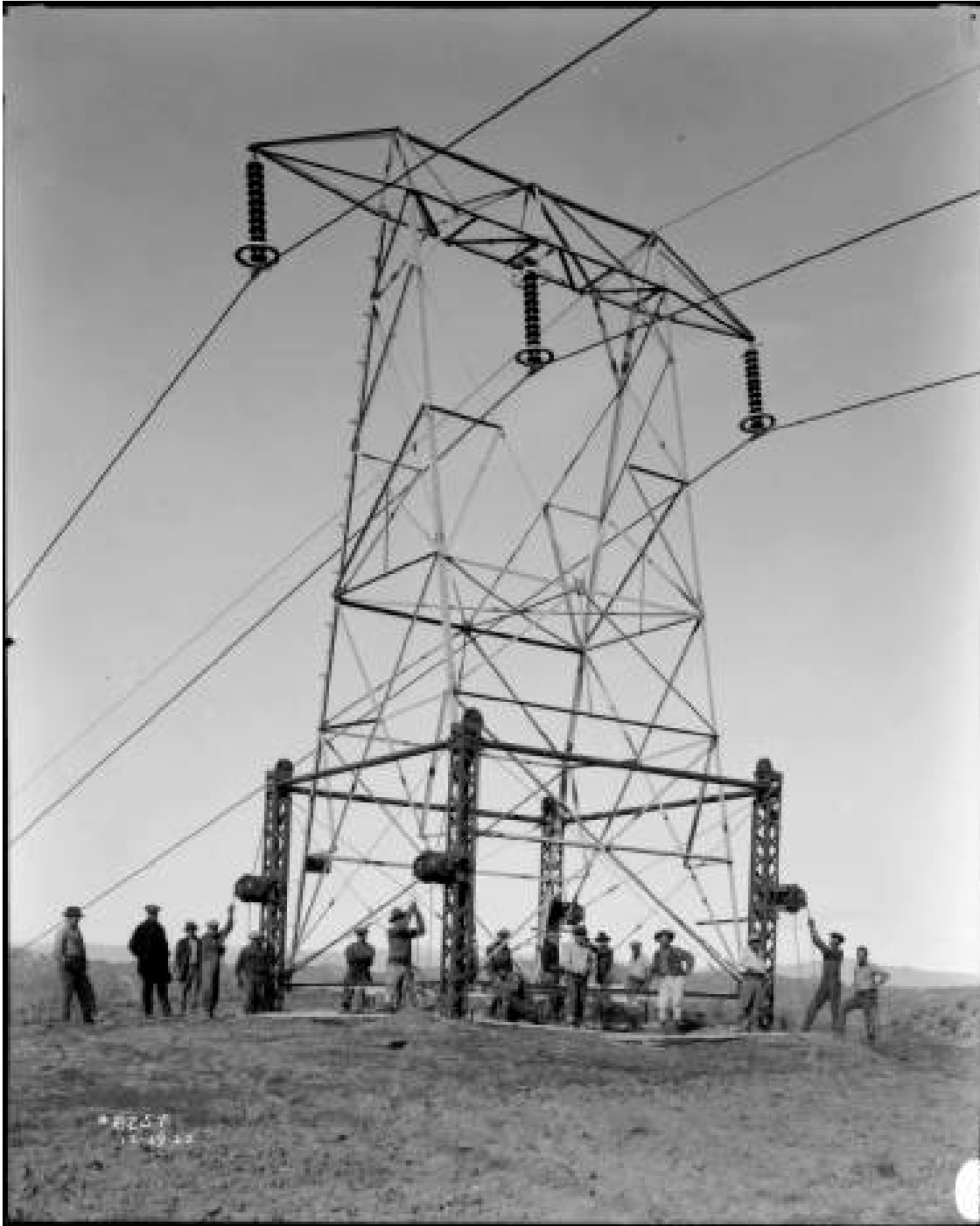
Figure 91: Raising Big Creek East and West Transmission Lines for 220 kV, 1922. Image No. SCE-02-08257, Huntington Digital Library.
