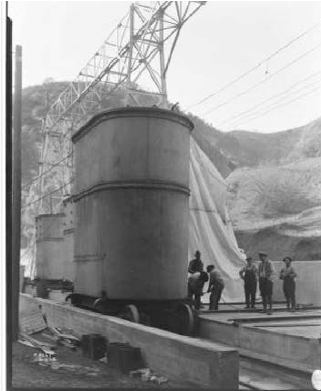
Figure 96: Eagle Rock 220 kV Transformer Installation, 1923. Image No. SCE-02-08263, Huntington Digital Library.
