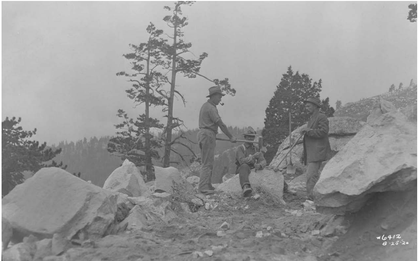
Figure 128: Kaiser Pass Road “double jack drillers,” 1920. Image No. SCE-02-06412, Huntington Digital Library.
