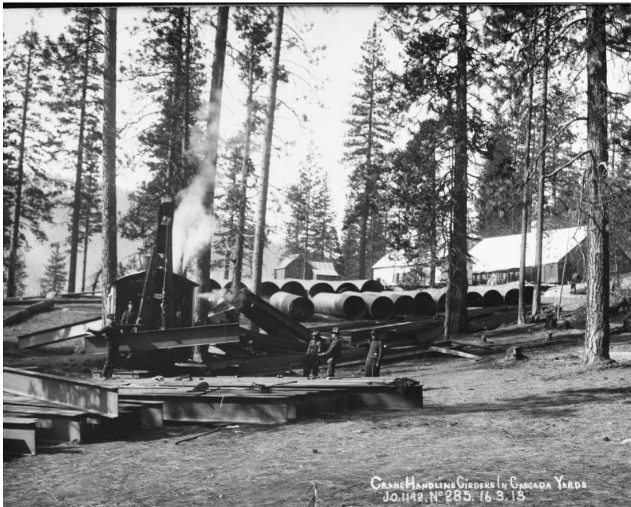
Figure 136: Cascada/Big Creek, 1913. Stone & Webster Construction Photographs, 13-Vol. 12, PO49, Huntington Digital Library.
