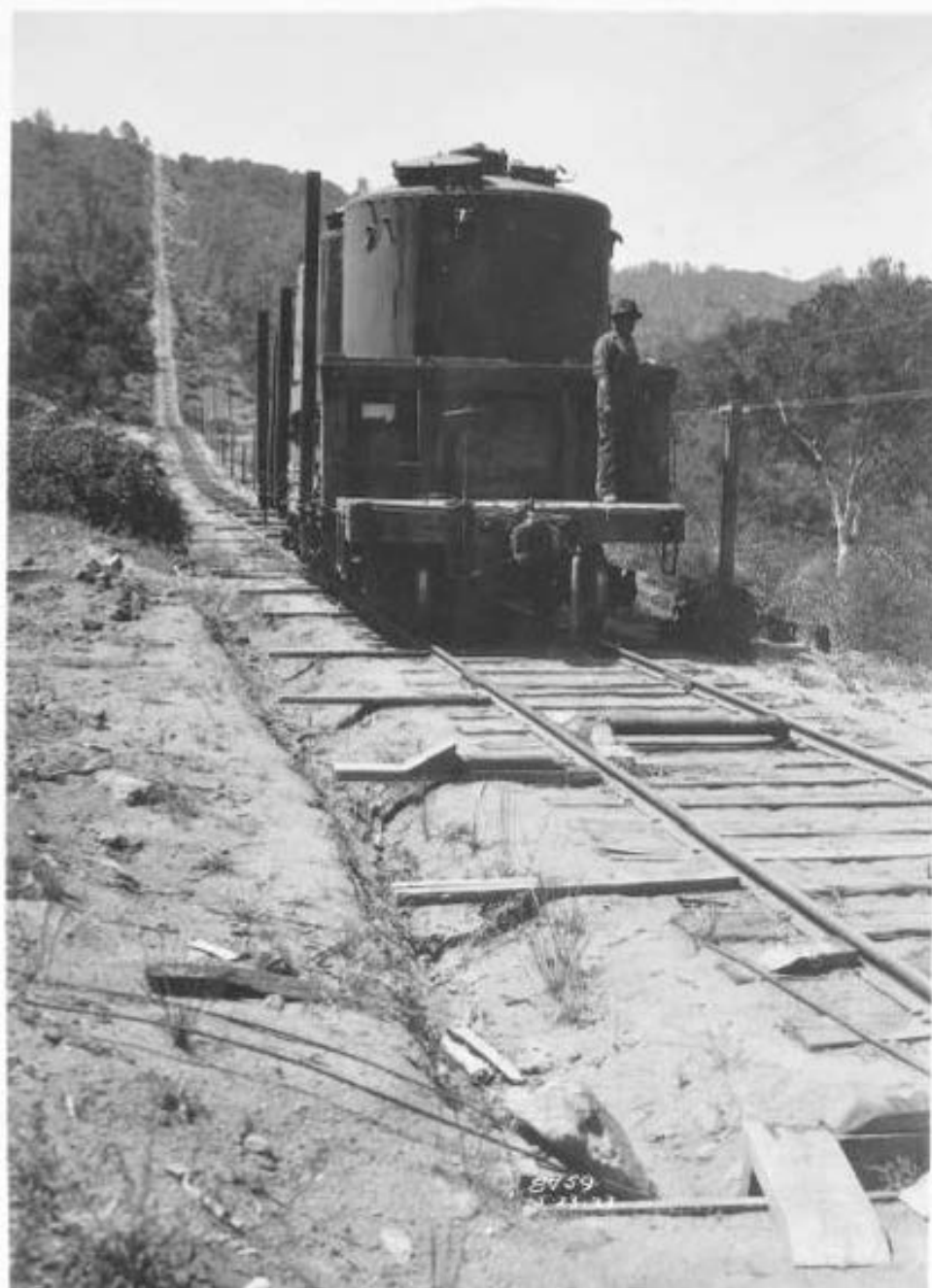
Figure 127: Incline No. 3 with 220 kV Circuit Breaker for Powerhouse No. 3, circa 1923. Call No. SCE, Big Creek Powerhouse #3, Part 1, 13-Vol. 32, P002, Huntington Digital Library.
