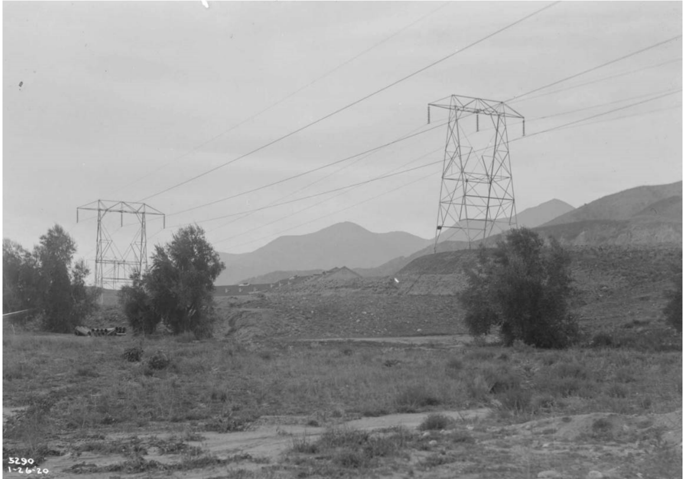
Figure 90: Big Creek East and West Transmission Lines near Los Angeles City Sanitarium near Silmar, 1920. Image No. SCE-02-08810, Huntington Digital Library.
