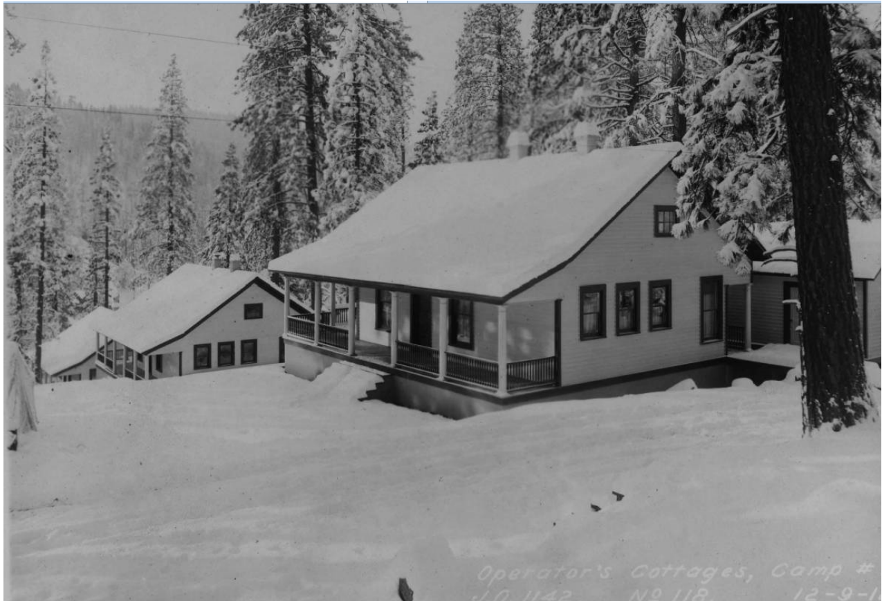
Figure 151: Big Creek Cottages, 1912. Image No. SCE-12-00034, Huntington Digital Library.
