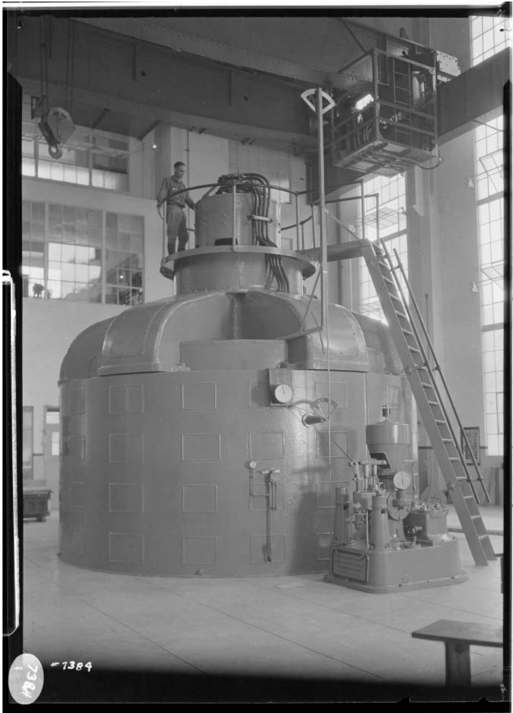
Figure 40: Powerhouse No. 8 Francis Type Turbine and Generator, 1921. Image No. SCE-02-07384, Huntington Digital Library.
