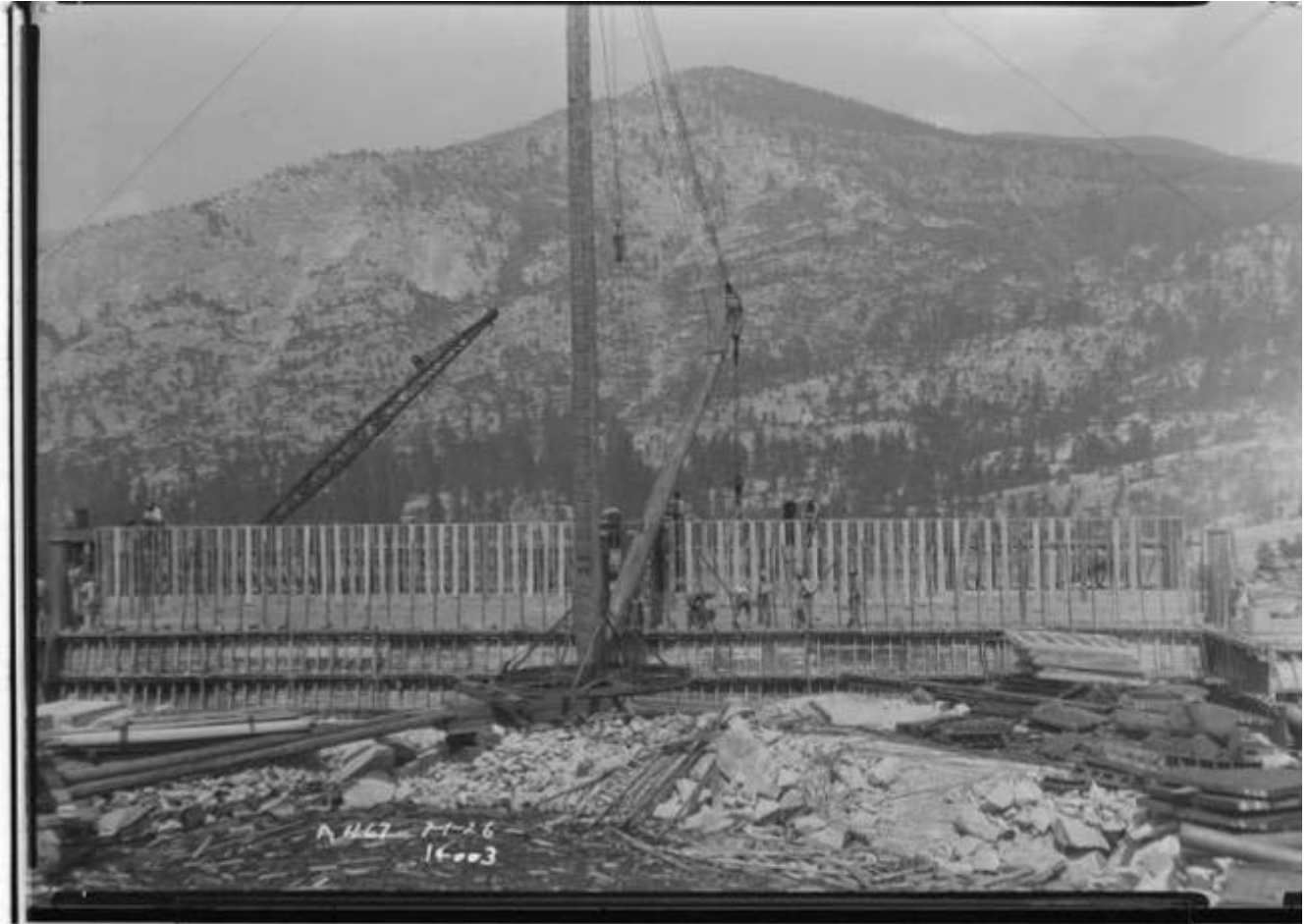
Figure 66: Florence Lake Dam Spillway, 1926. Image No. SCE-02-14003, Huntington Digital Library.
