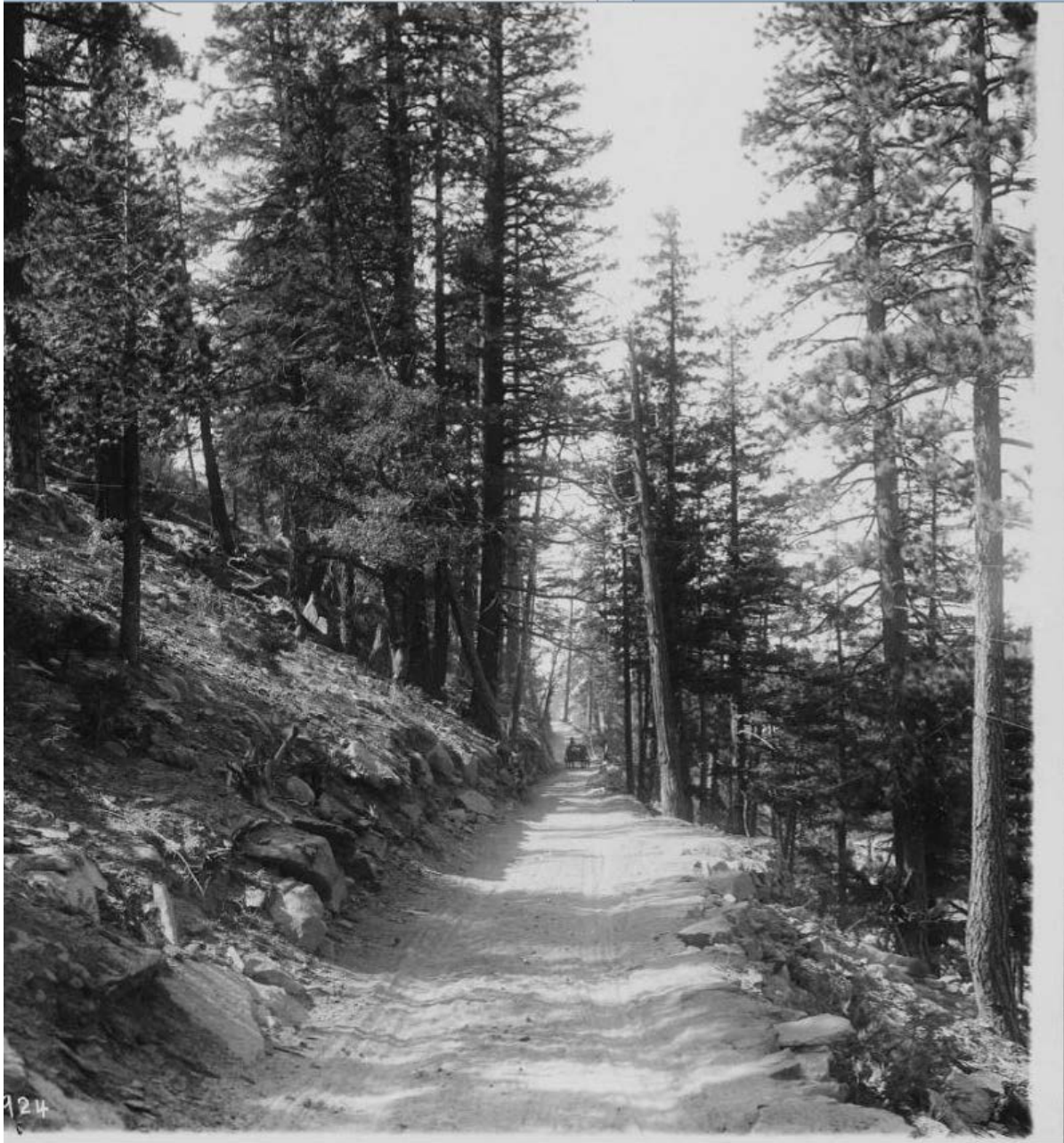
Figure 108: SJ&E grade under construction, 1912. Pacific Light and Power Corporation, 13-Vol. 018, Huntington Digital Library.
