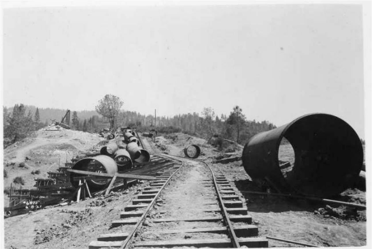
Figure 123: Incline No. 8 with penstock sections surrounding, circa 1920. Call No. SCE, Big Creek Powerhouse #8, Part 2, 13-Vol. 35, PO93, Huntington Digital Library.
