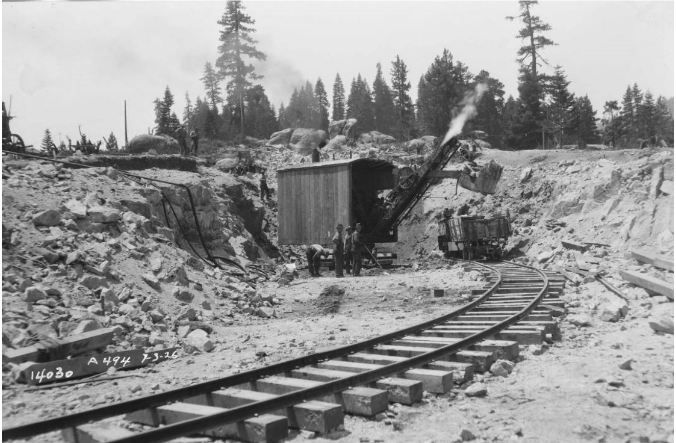
Figure 134: Dawn Railroad Spur, excavating Shaver Lake Dam with Marion Steam Shovel, 1926. Image No. SCE-02-14030, Huntington Digital Library.
