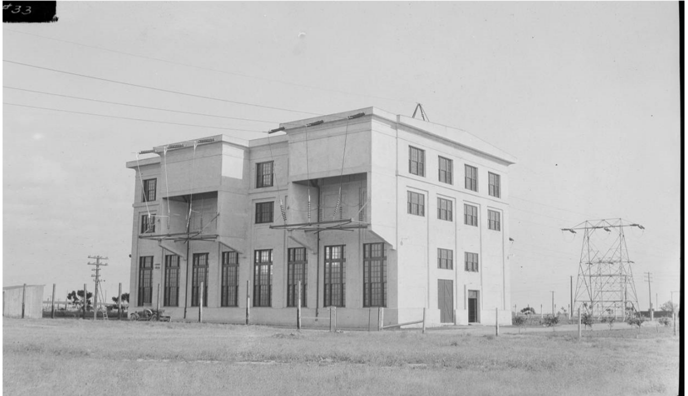
Figure 98: Magunden Substation, 1917. Image No. SCE-03-00956, Huntington Digital Library.
