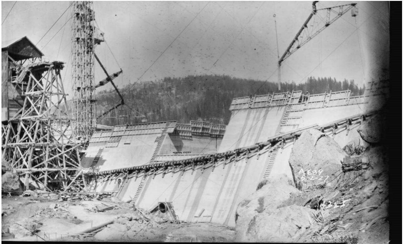
Figure 80: Shaver Lake Dam Construction, 1927. Image No. SCE-02-14325, Huntington Digital Library.
