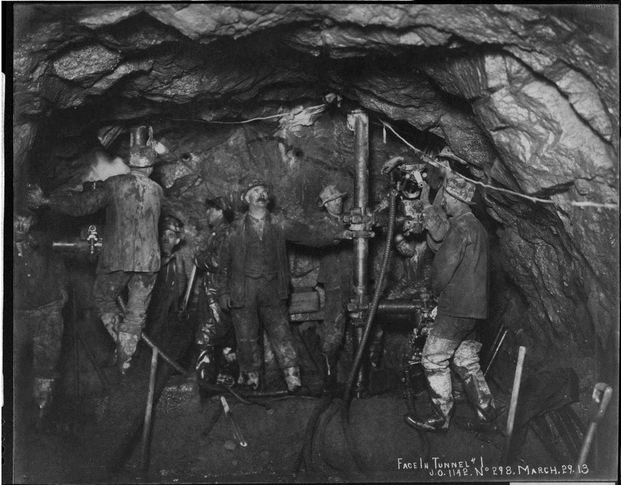
Figure 9: Working face in Tunnel No.1 Flowline, 1913. Image No. SCE-02-00029, Huntington Digital Library.
