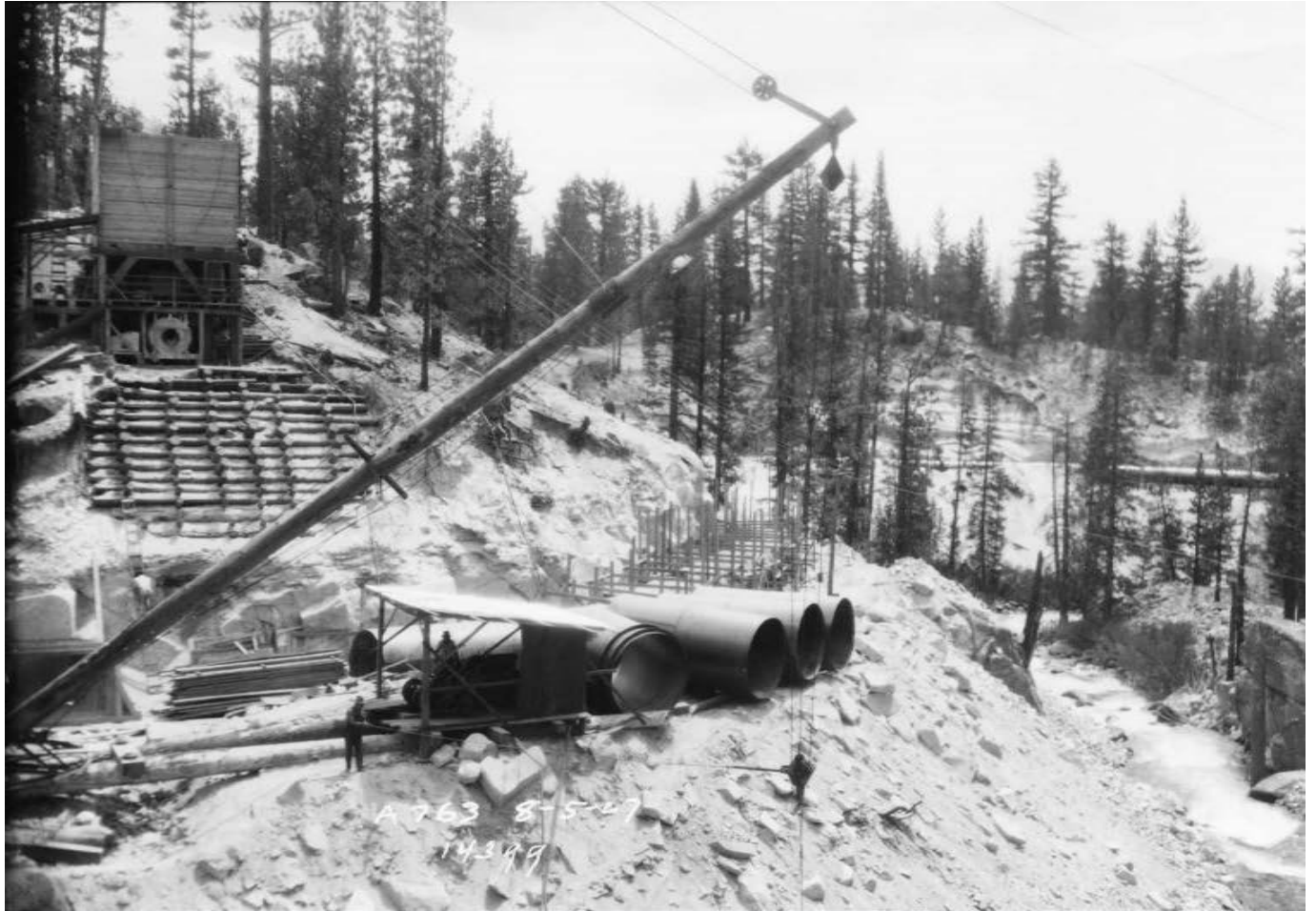
Figure 76: Mono Siphon construction, 1927. Image No. SCE-02-14399, Huntington Digital Library.
