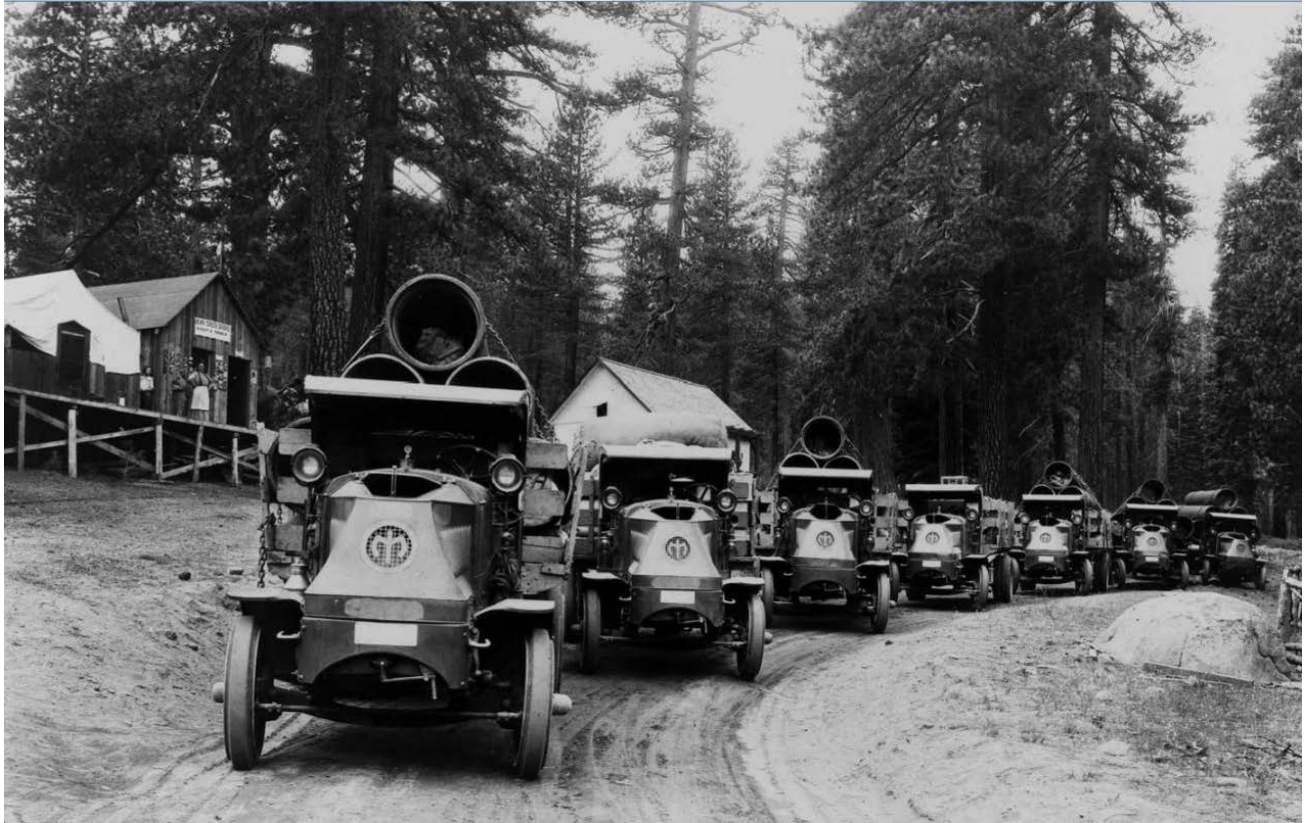
Figure 131: Mack Bull-Dogs at the base of Kaiser Pass Road with pipe for Mono-Bear Siphon, 1927. Image No. SCE-11-00233, Huntington Digital Library.
