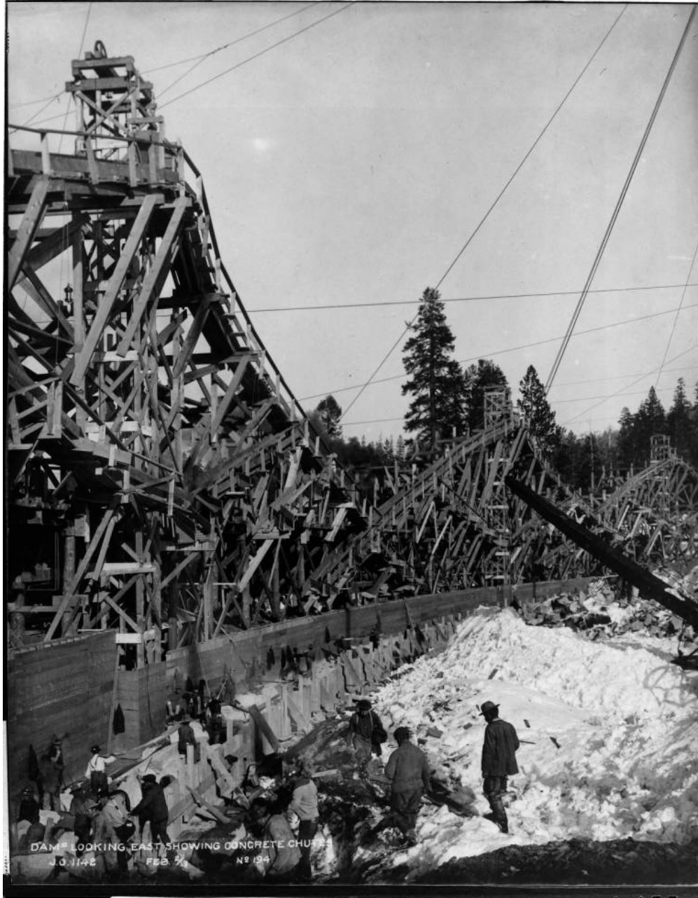
Figure 1: Huntington Lake Dam No. 1, circa February 1913.
