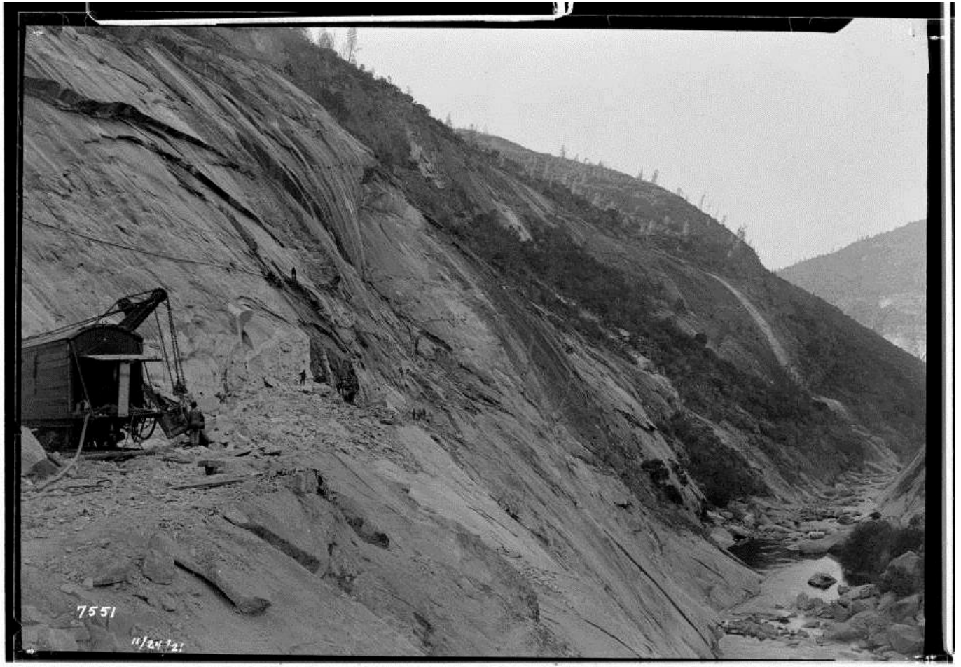
Figure 125: Million Dollar Mile Road excavation, 1921. Image No. SCE-02-07551, Huntington Digital Library.
