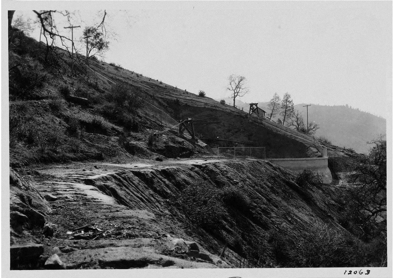
Figure 43: Tunnel No. 3 Surge Chamber, 1924. Image No. SCE-02-12063, Huntington Digital Library.
