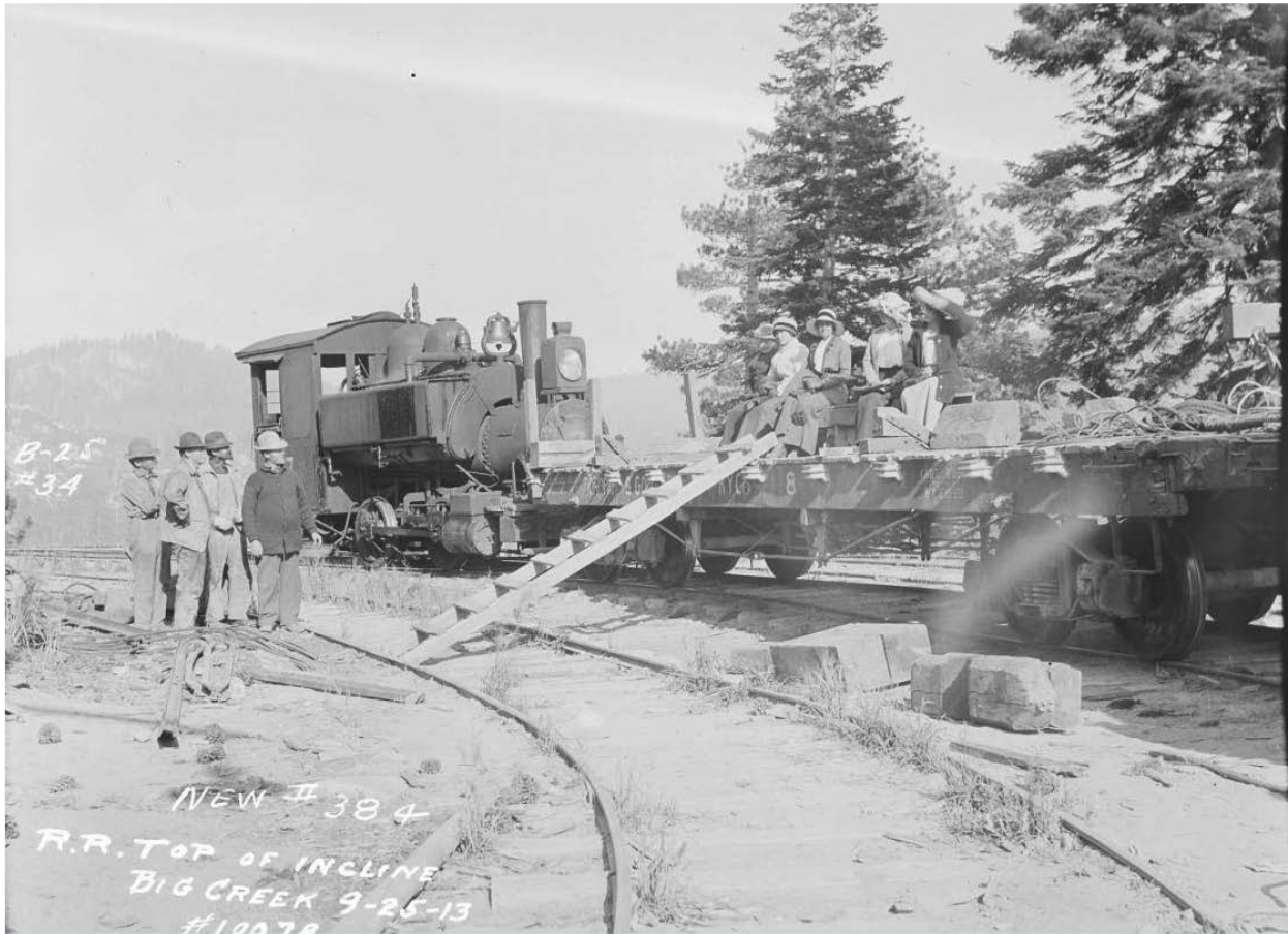
Figure 118: Basin Railroad at top of Incline No. 1, 1913. Call No. SCE-03-00384, Huntington Digital Library.
