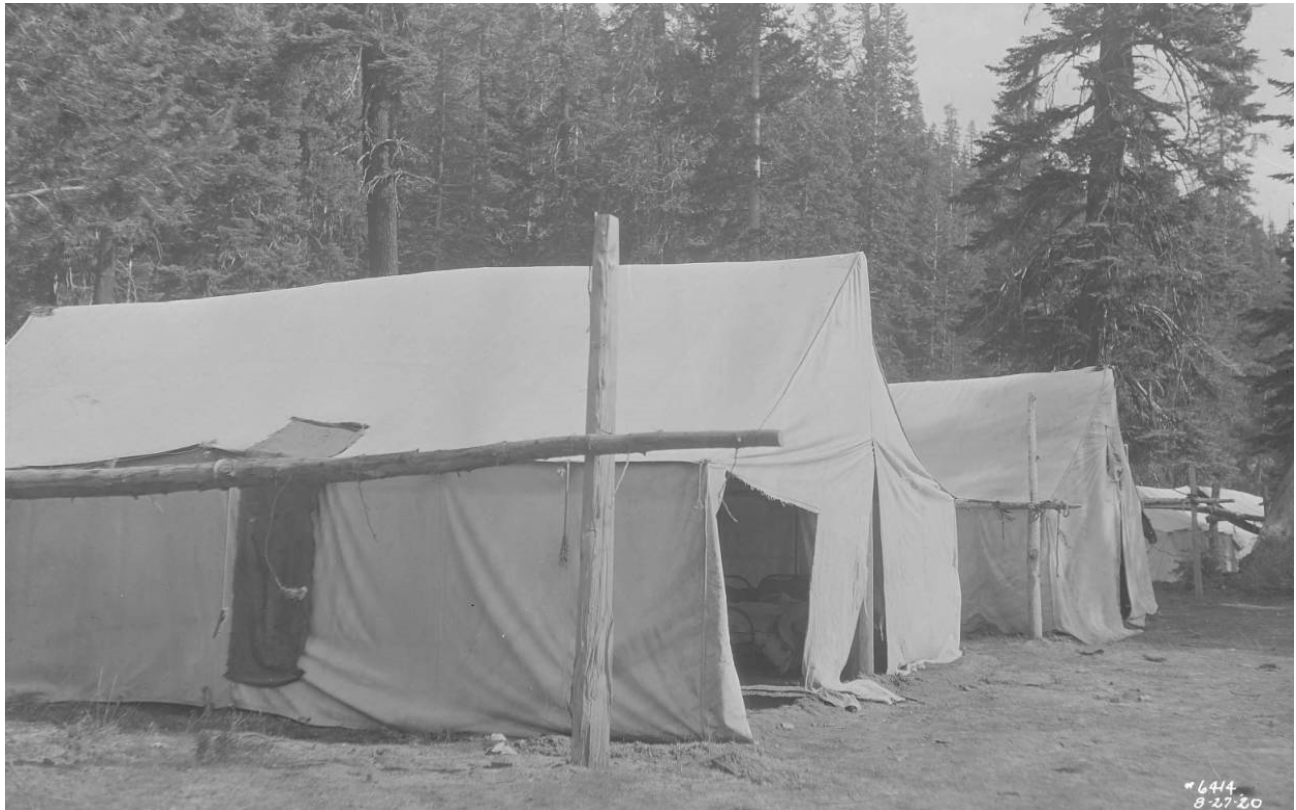
Figure 141: Kaiser Pass Road Construction Camp, 1920. Photo No. SCE-02-06414, Huntington Digital Library.
