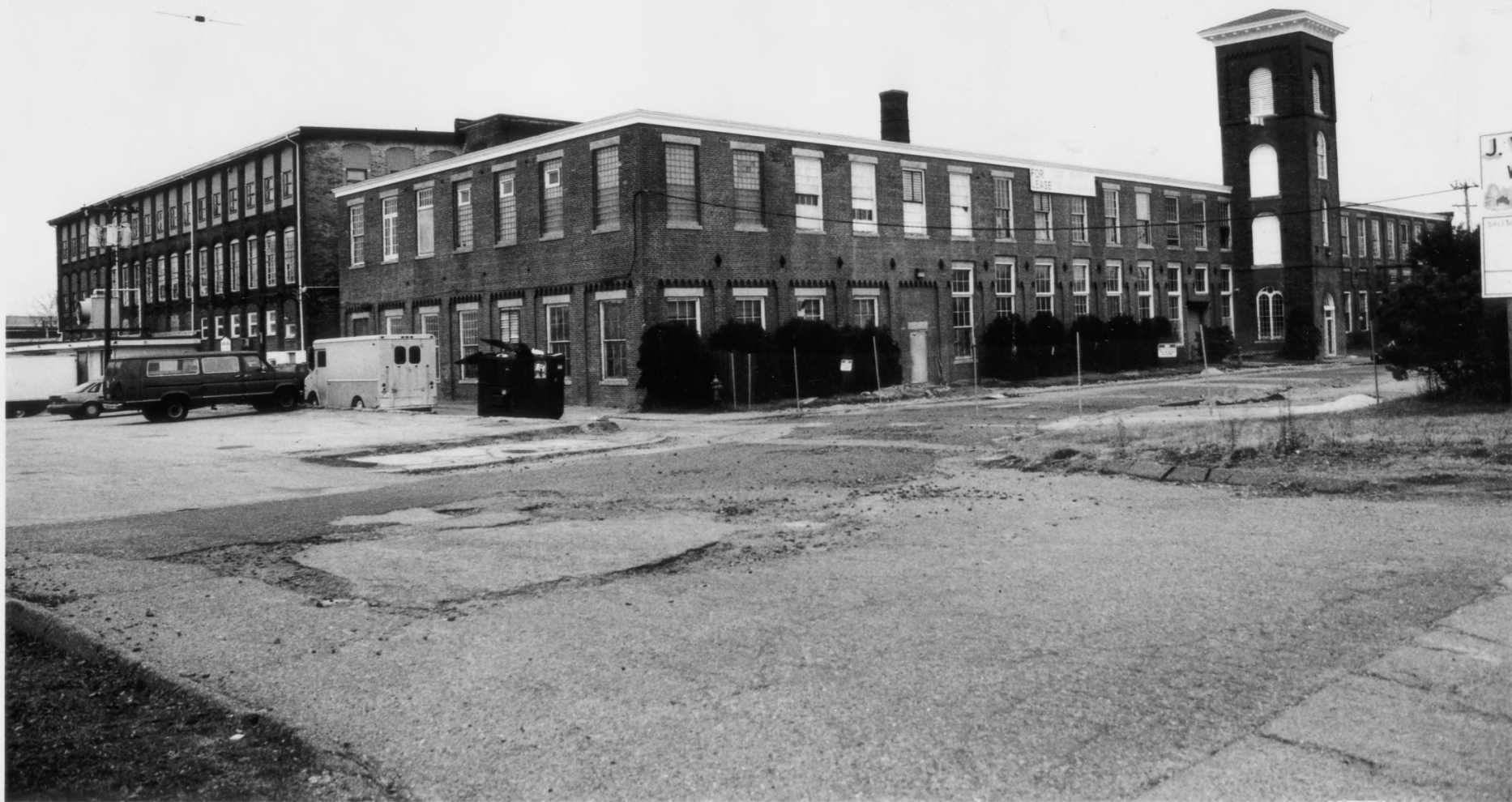
Building 11 and Building 12/Building 13 Shade Island Text, Sewing Plant, Providence County, Rhode Island Photograph No. 1
