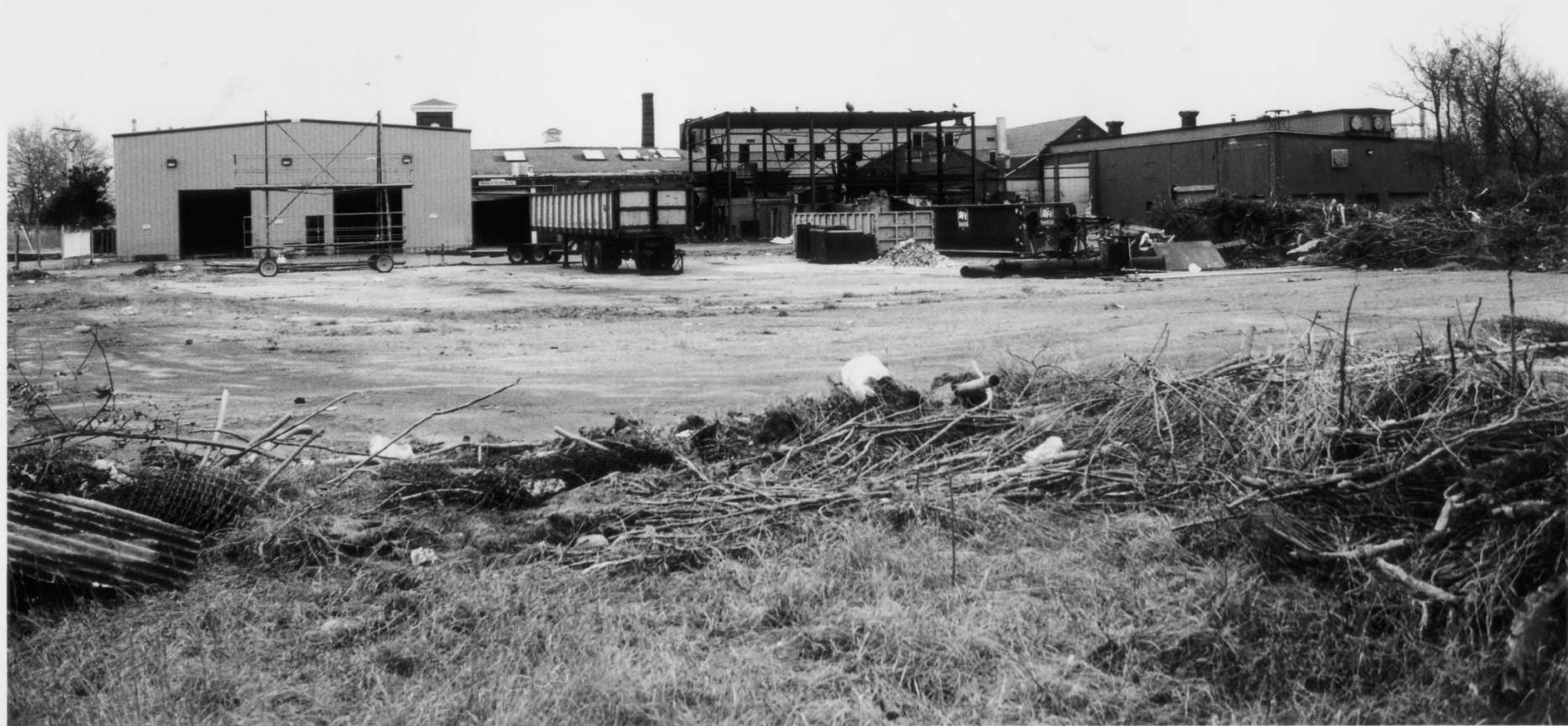
Building 27, Building 26, and Building 22 Rhode Island Tool Company Providence, Providence County, Rhode Island Photograph No. 6
