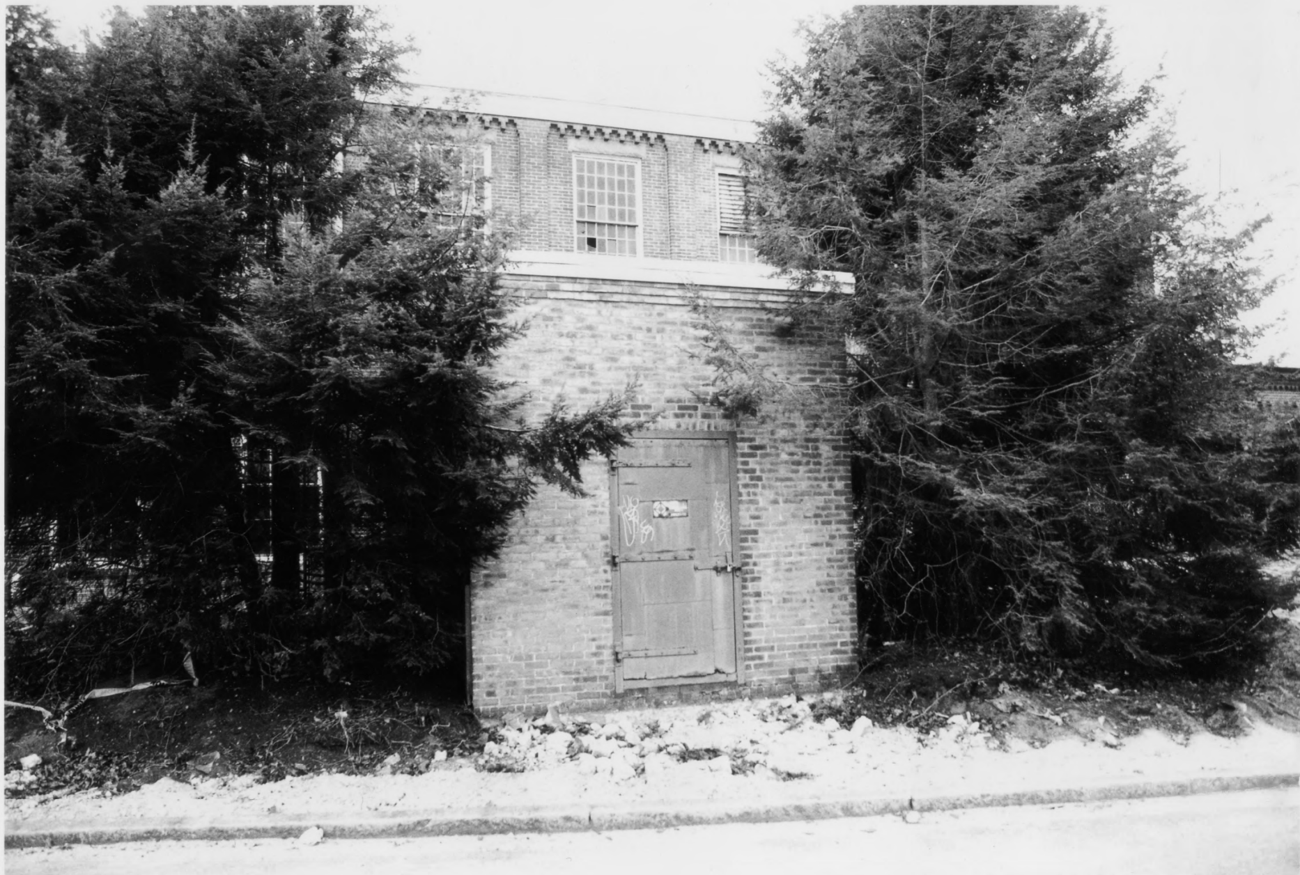
East Division of Electrical, Gas & Power Riviera Telephone Company Providence, Rhode Island Photograph 19-2
