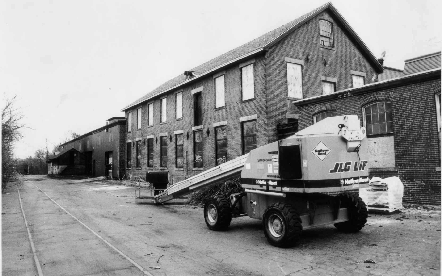
Building 22, Building 5 and Building 6 Rhode Island Tool Company Providence, Providence County, Rhode Island Photograph No. 10
