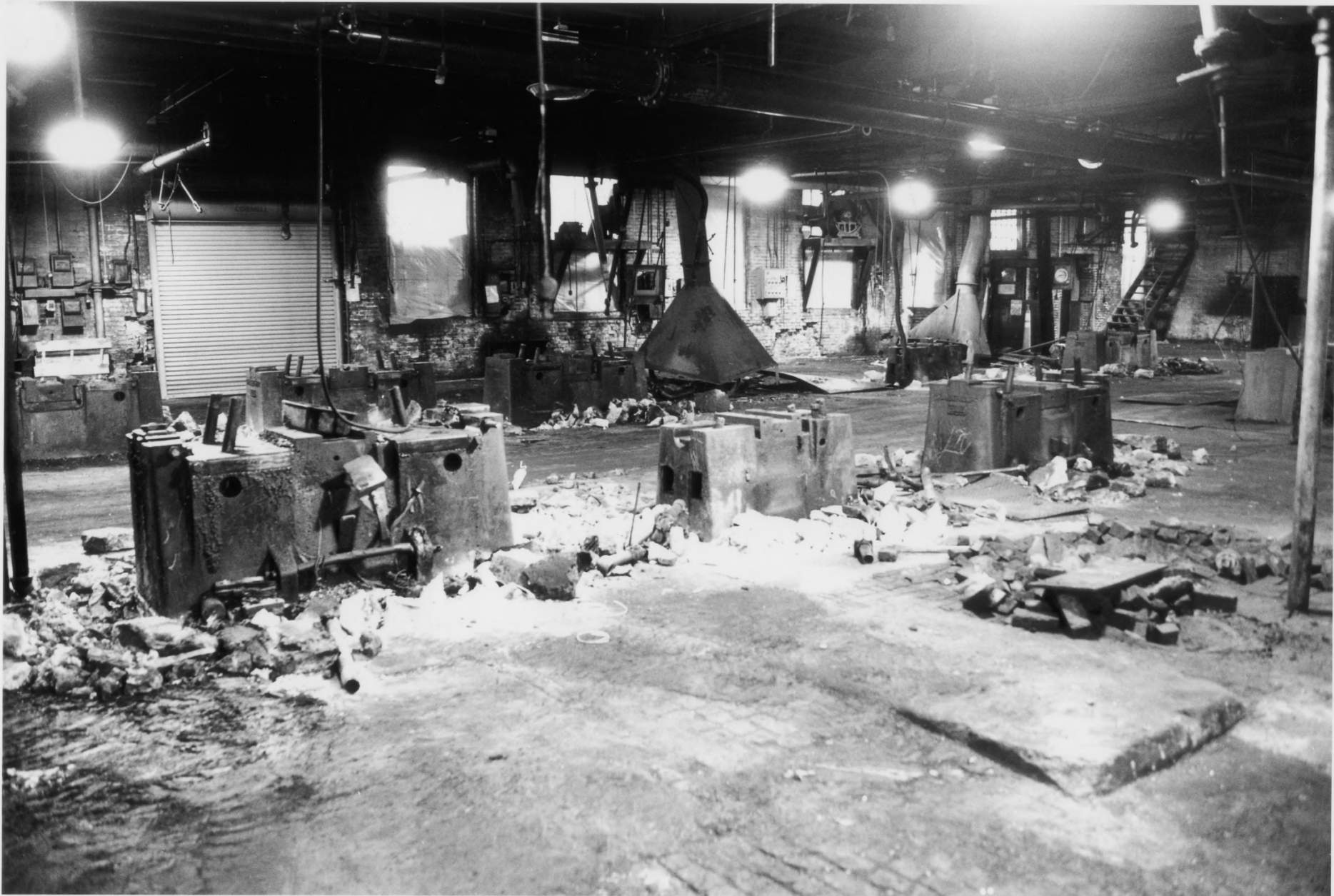
Interior of Building A looking West Rhode Island Tool Company Providence, Providence County, Rhode Island Photograph No. 16
