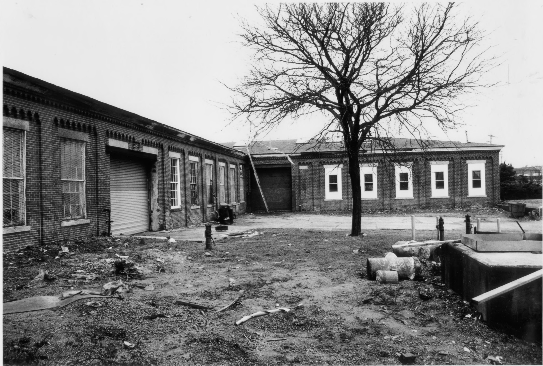
Building 2 and Building 3 Rhode Island Tool Company, Providence, Providence County, Rhode Island Photograph No. 4
