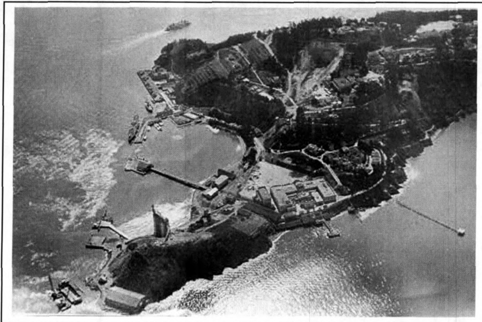
Figure 5. Yerba Buena Island during the San Francisco-Oakland Bay Bridge construction, circa 1934. Building 262 shown bottom left. [HABS No. CA-1793-3]
