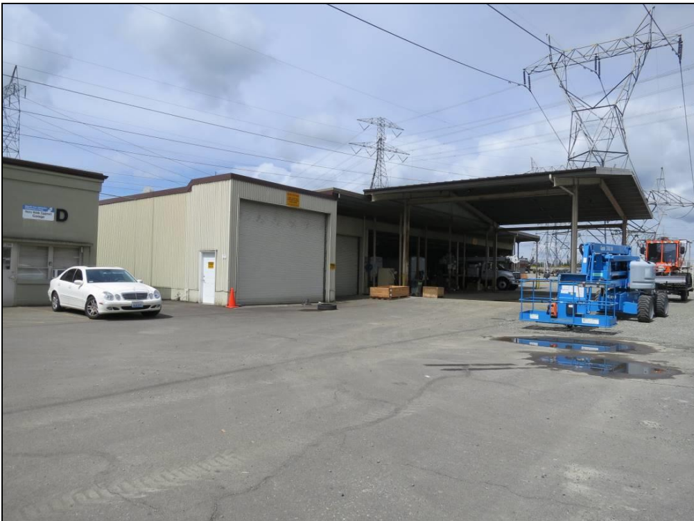
Photo 13 of 22: Automotive Storage (1959), looking west. (WA_KingCounty_CovingtonSubstation_0013)
