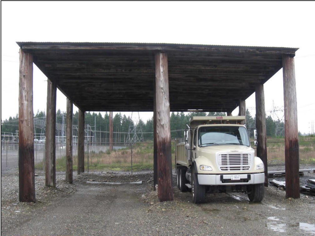
Photo 18 of 22: TLM Vehicle Canopy (1971), looking southwest. (WA_KingCounty_CovingtonSubstation_0018)
