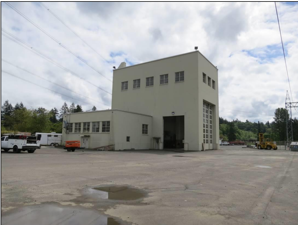
Photo 3 of 22: Non-public side of Untanking Tower (1942), looking east. (WA_KingCounty_CovingtonSubstation_0003)
