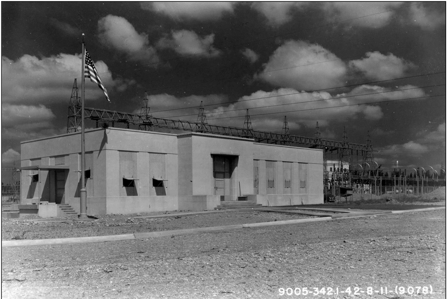
Figure 14. Covington Control House looking north in August 1942 with protective plywood over the window openings. BPA photo 9005-342.1-42-8-11-(9078).
