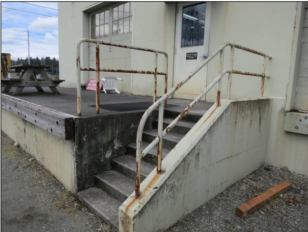
Photo 5 of 22: Loading dock of Untanking Tower (1942), southeast side, looking west. (WA_KingCounty_CovingtonSubstation_0005)
