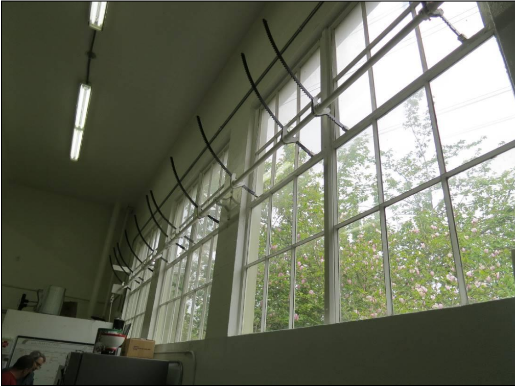
Photo 6 of 22: Window detail, workroom, Untanking Tower (1942), looking north. (WA_KingCounty_CovingtonSubstation_0006)
