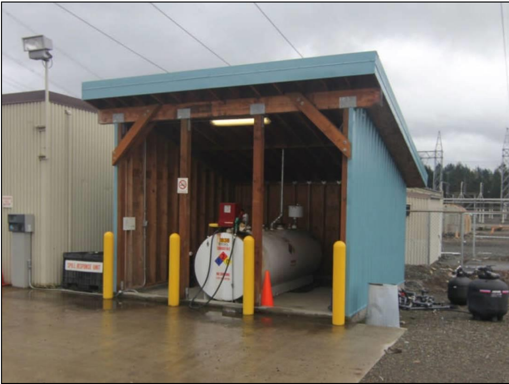
Photo 22 of 22: Fueling Station (2011), looking east. (WA_KingCounty_CovingtonSubstation_0022)
