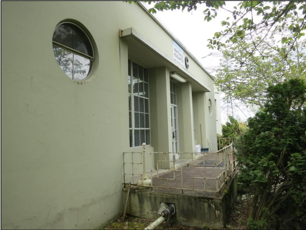
Photo 4 of 22: Public entry porch, Untanking Tower (1942), looking northwest. (WA_KingCounty_CovingtonSubstation_0004)
