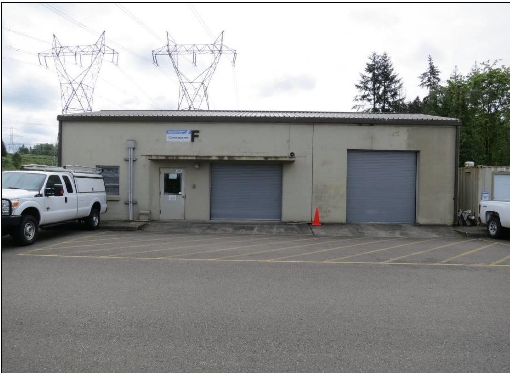
Photo 15 of 22: Communications Building (1958), looking southeast. (WA_KingCounty_CovingtonSubstation_0015)
