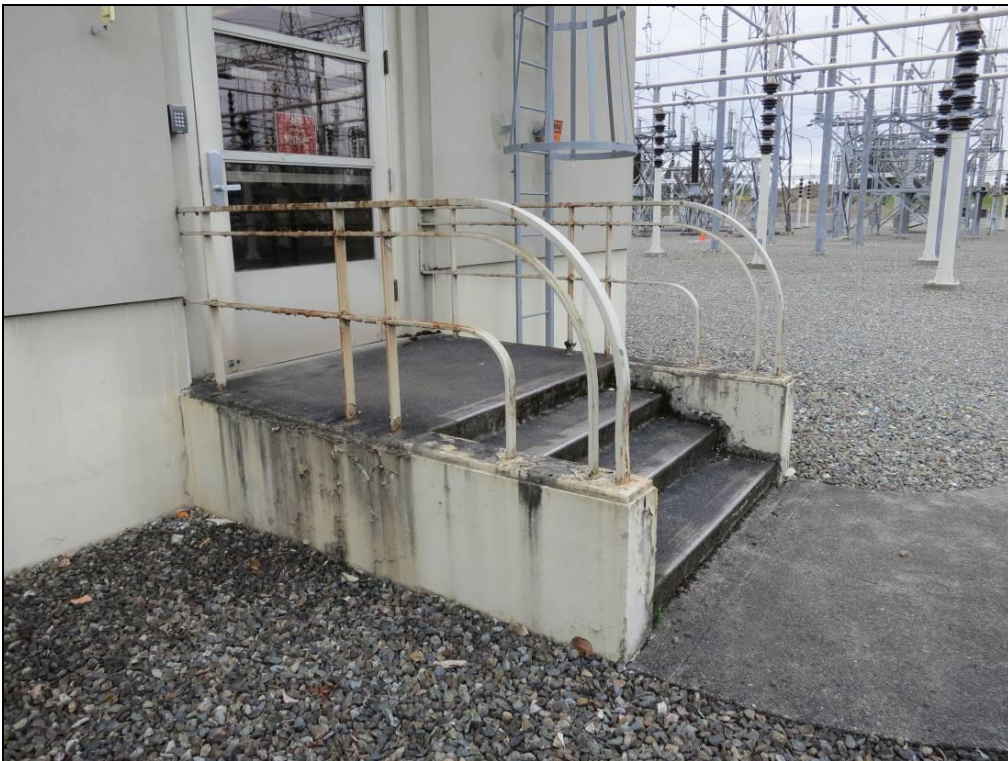
Photo 9 of 22: Side entry detail, northeast side, Control Building (1942), looking west. (WA_KingCounty_CovingtonSubstation_0009)
