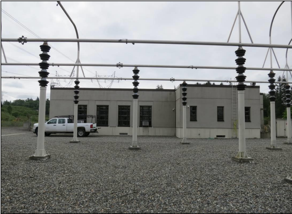
Photo 8 of 22: Switchyard side of Control Building (1942), looking southeast. (WA_KingCounty_CovingtonSubstation_0008)
