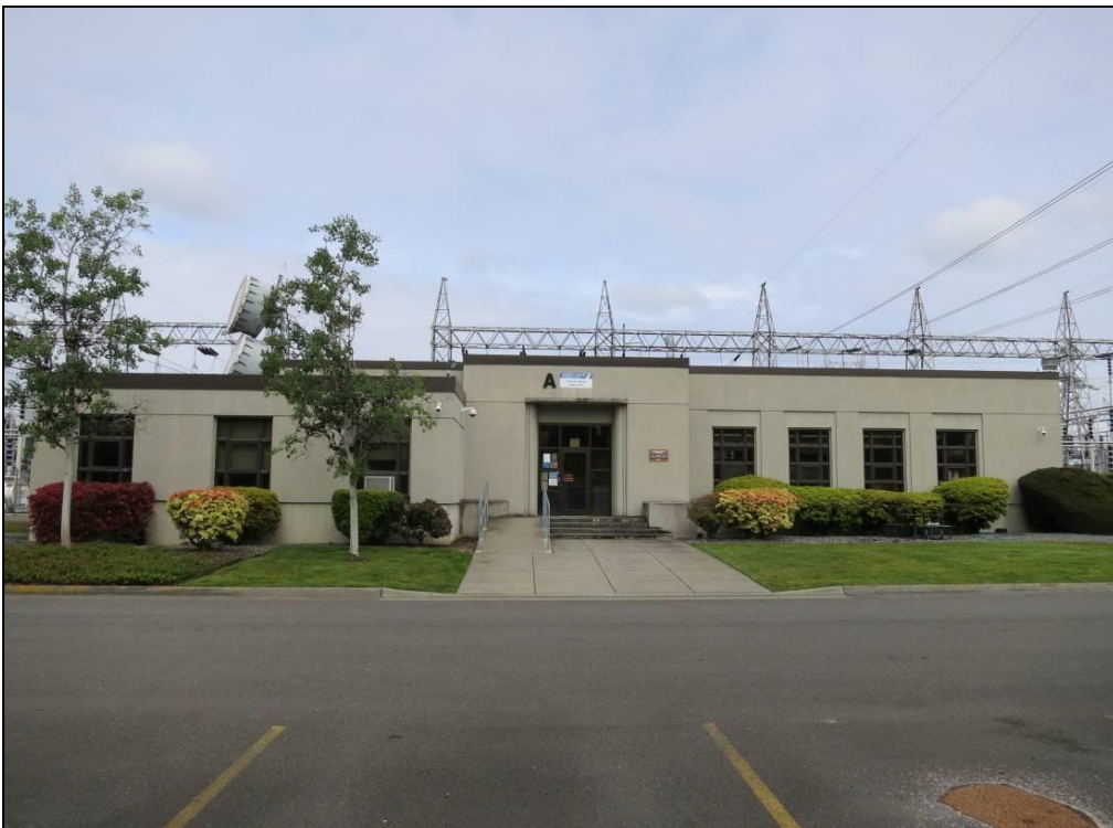
Photo 7 of 22: Public side of Control Building (1942), looking northwest. (WA_KingCounty_CovingtonSubstation_0007)
