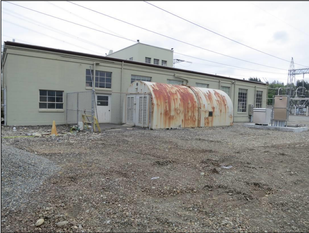
Photo 12 of 22: Rear façade, HMEM Shop (1953), looking east. (WA_KingCounty_CovingtonSubstation_0012)
