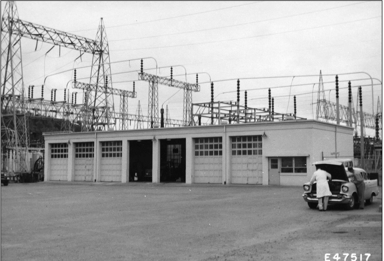
Figure 17. Covington Garage (aka HMEM Shop) looking south in June 1958 before door replacement. BPA photo E47517.
