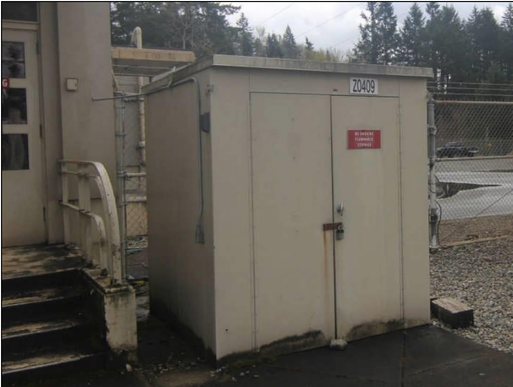
Photo 20 of 22: Control House Flammable Storage Building (1966), looking south. (WA_KingCounty_CovingtonSubstation_0020)
