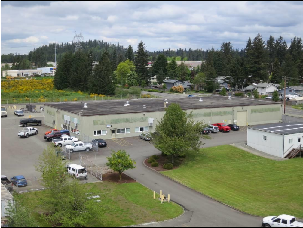
Photo 14 of 22: Maintenance Warehouse (1959), from roof of Untanking Tower, looking north. (WA_KingCounty_CovingtonSubstation_0014)
