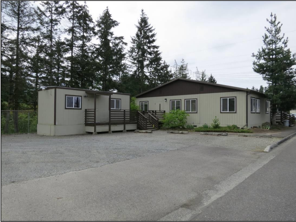
Photo 16 of 22: SPC Shop (2004) and PSC & SPC Office (1996), looking south. (WA_KingCounty_CovingtonSubstation_0016)
