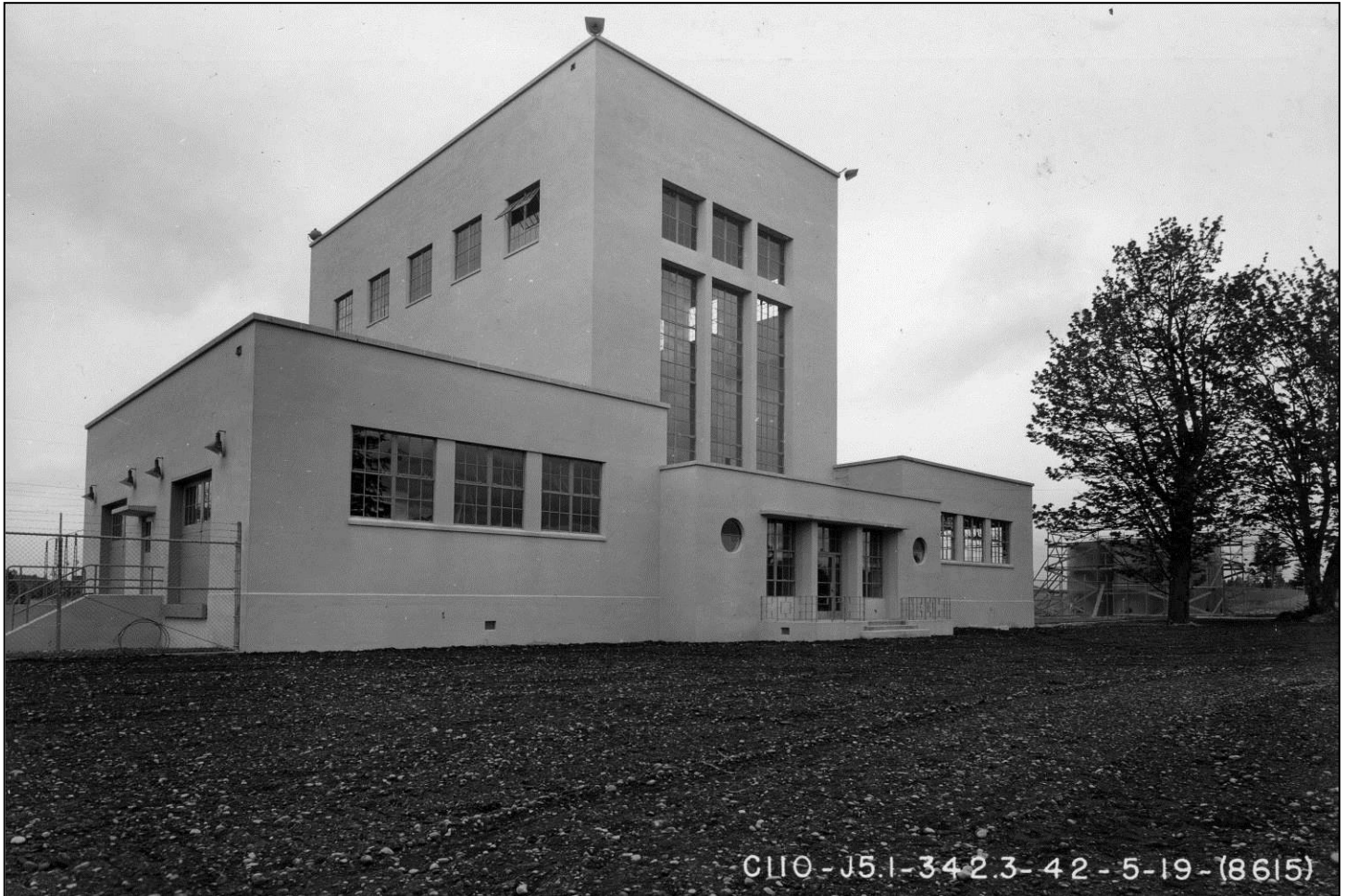
Figure 13. Covington Untanking Tower looking west in May 1942 soon after completion. Oil tanks still under construction at far right. BPA photo C110-J5.1-342.3-42-5-19-(8615).
