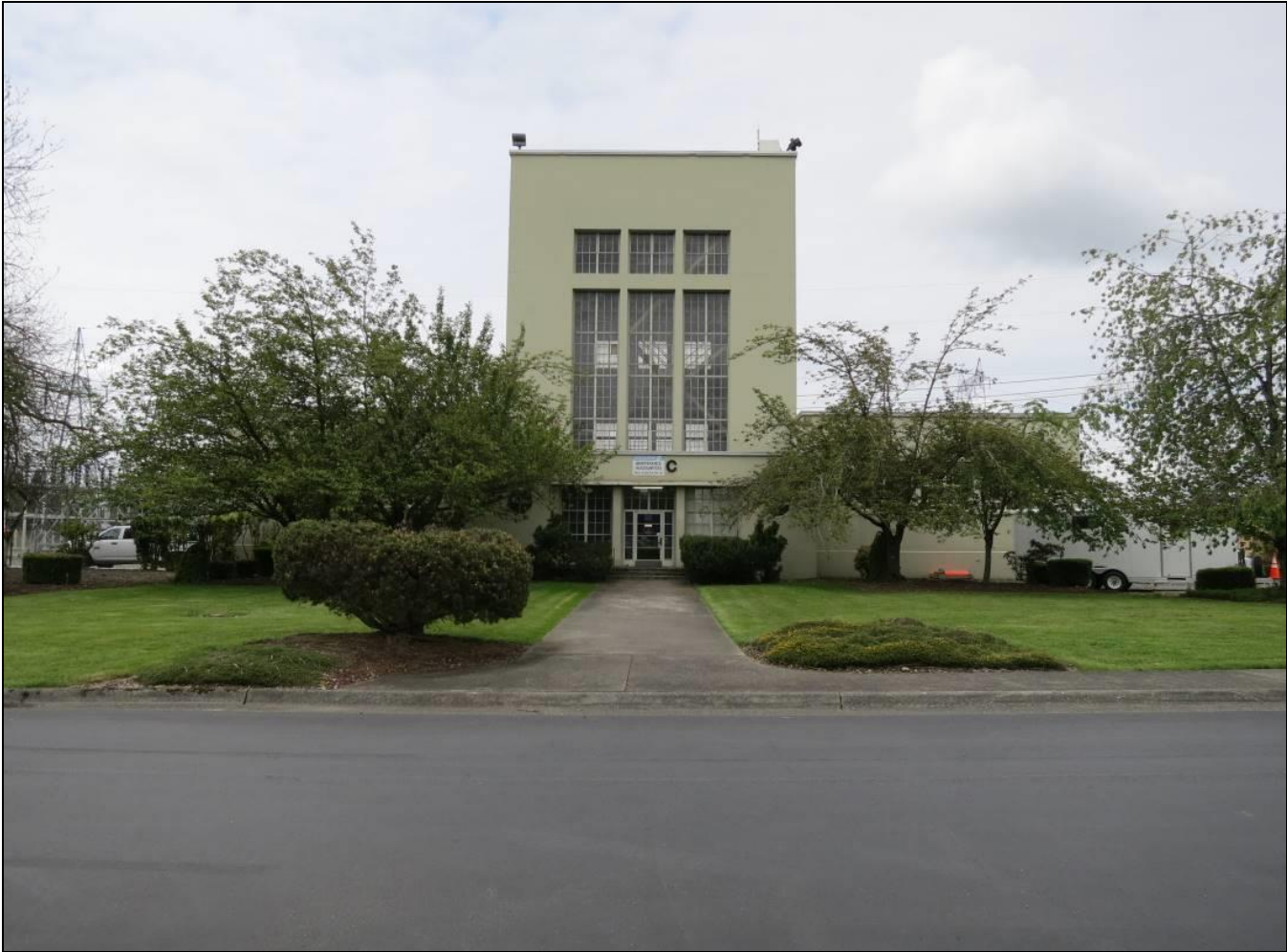
Photo 1 of 22: Public side of Untanking Tower (1942), looking southwest. (WA_KingCounty_CovingtonSubstation_0001)
