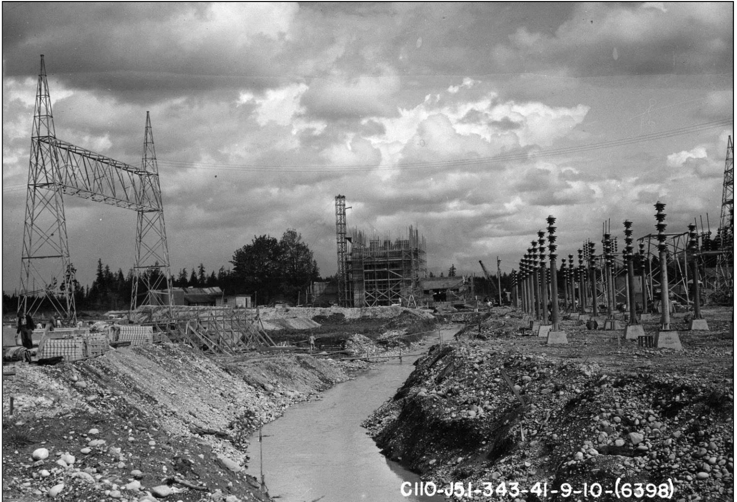
Figure 11. View looking northeast through the Switchyard towards the Untanking Tower under construction in September 1941. Jenkins Creek still in the middle of the Switchyard before diversion to the southeastern edge of the complex. BPA photo C110-J5.1-343-41-9-10-(6398).
