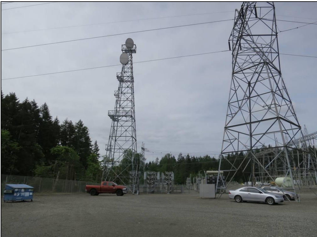
Photo 19 of 22: Microwave Tower (c.1968), looking southwest. (WA_KingCounty_CovingtonSubstation_0019)
