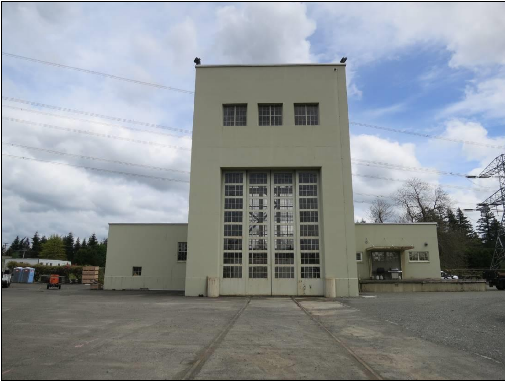
Photo 2 of 22: Non-public side of Untanking Tower (1942), looking northeast. (WA_KingCounty_CovingtonSubstation_0002)
