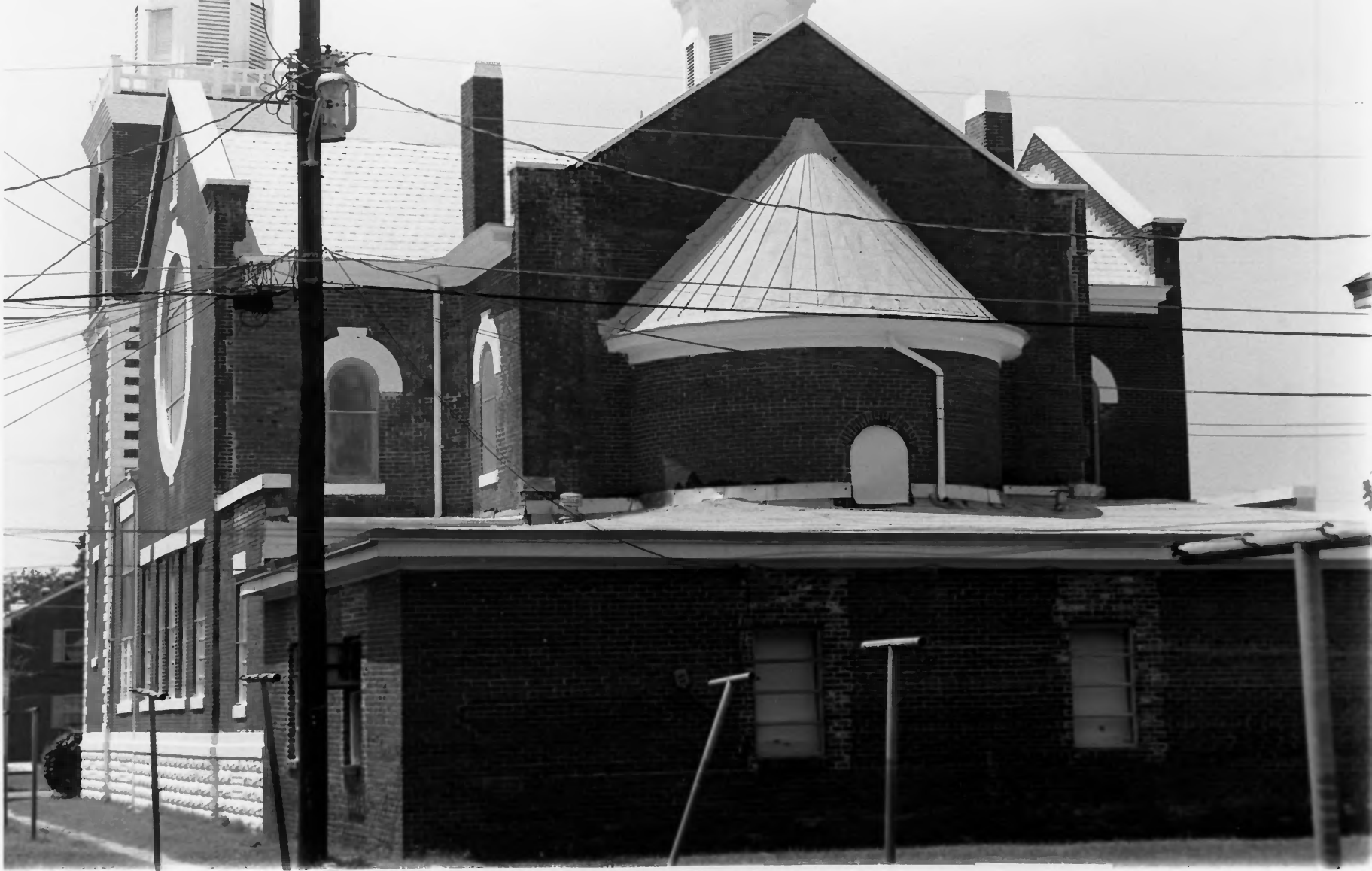
Photograph #2 Brown Chapel AME Church, Selma, AL Perry Varner, August 1997 Rear (east) and side (south) elevations, showing nave and rear addition.
