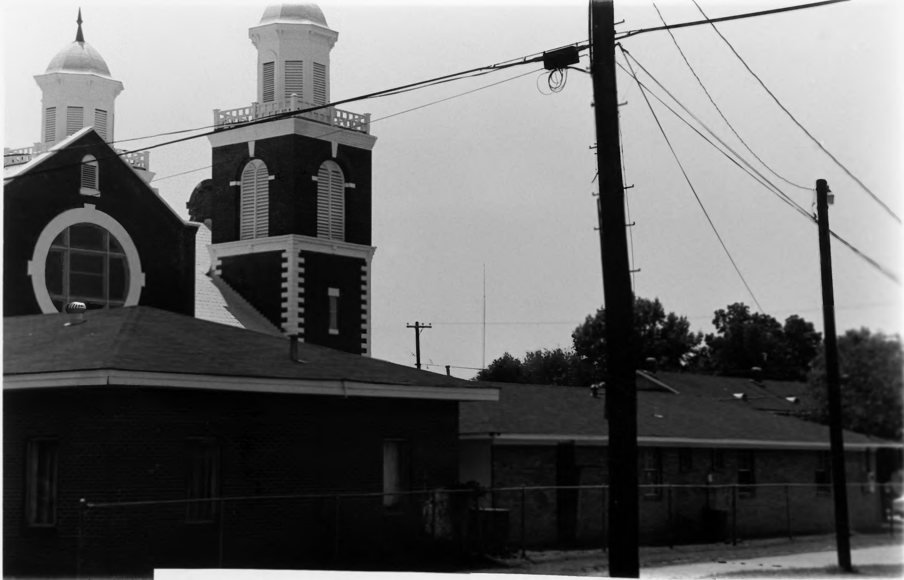
Photograph #3 Brown Chapel AME Church, Selma, AL Perry Varner, August 1997 Side (west) elevations, showing addition (left) and parsonage (right).
